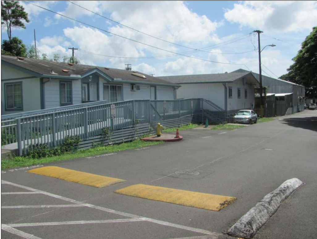
Figure 14. Grading, parking, utility, and building construction in the central part of study area, view to the southeast.
