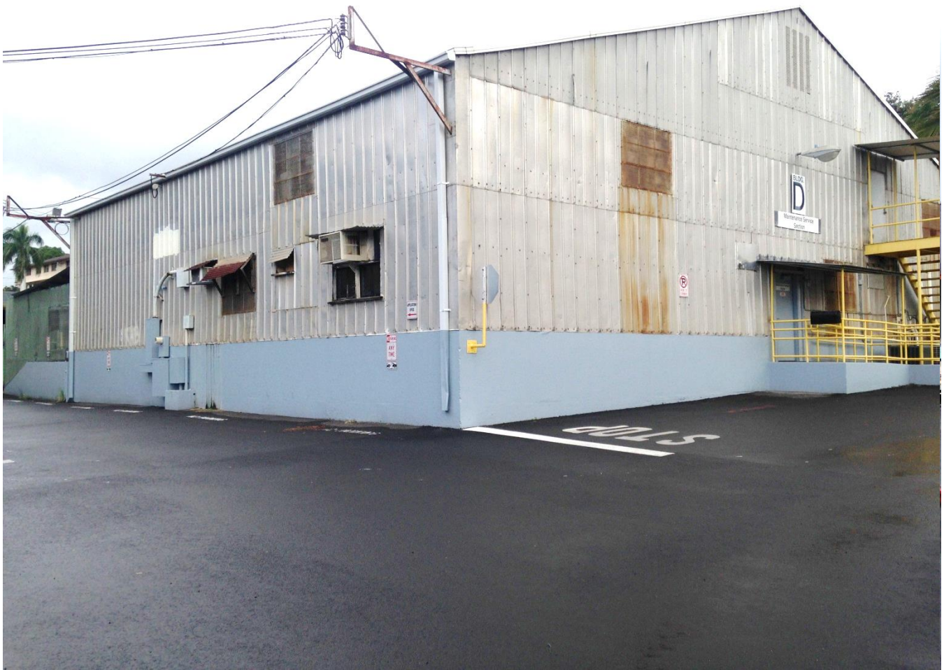
Building D: Maintenance Service Section, view facing north.
