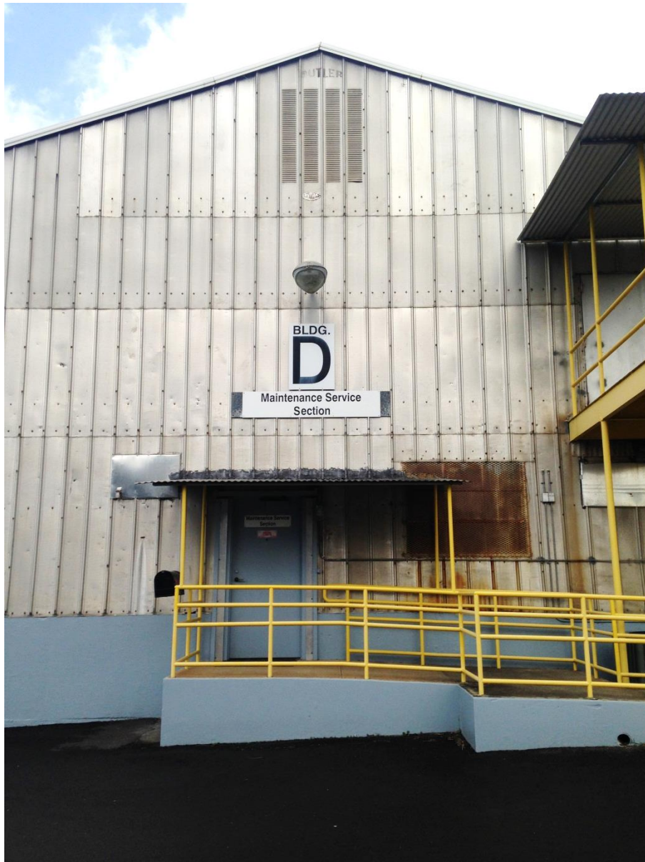
Building D: Maintenance Service Section, view facing northwest. "Butler" logo visible near ridge.
