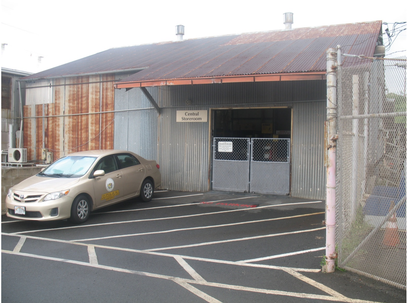
Central Storeroom Building, view facing west.
