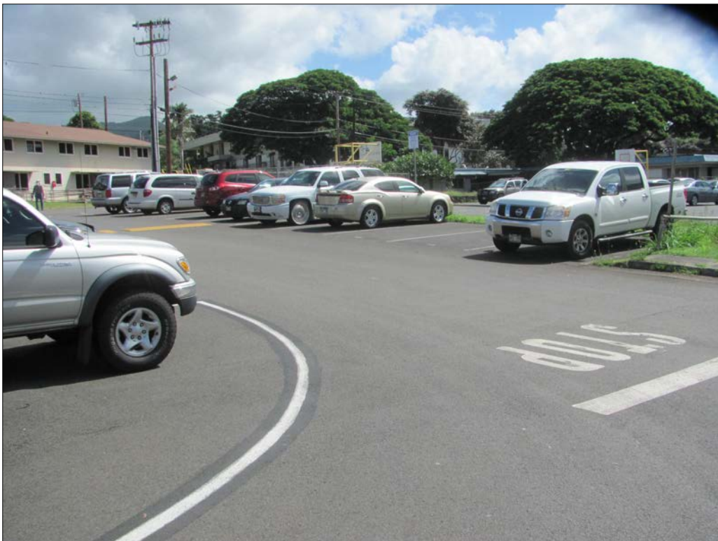
Figure 15. Grading, parking, drainage, utility, and building construction along the northeast side of the study area, view to the east.
