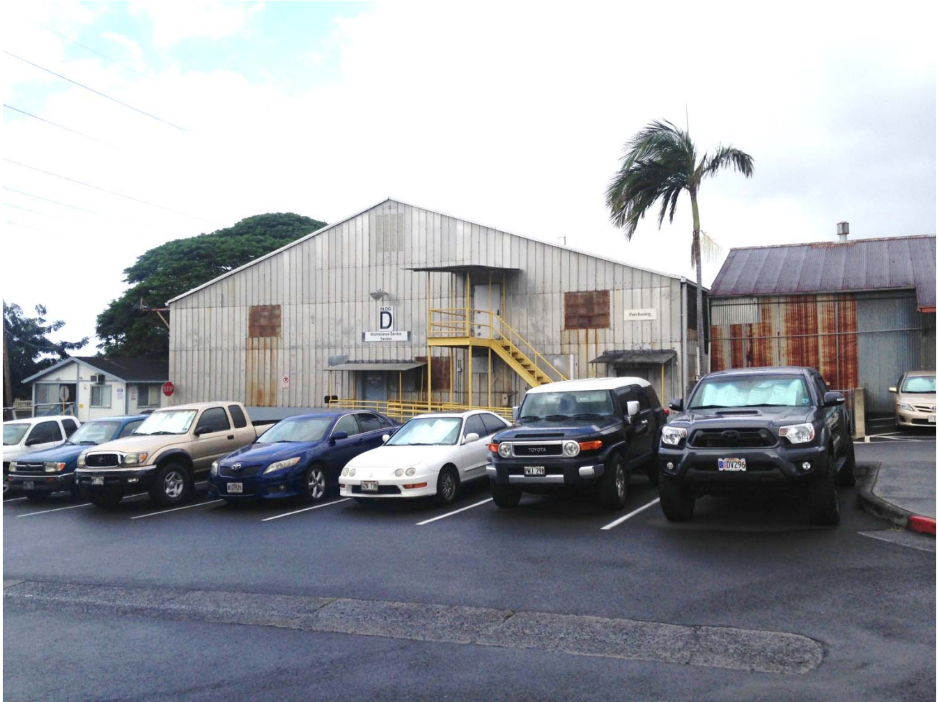
Building D and Central Storeroom Building: view facing northwest.
