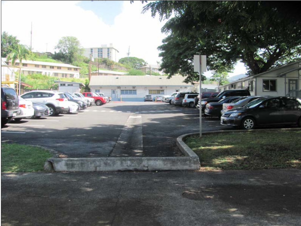
Figure 10. Grading, parking, drainage, and building construction in the central part of study area, view to the northeast.
