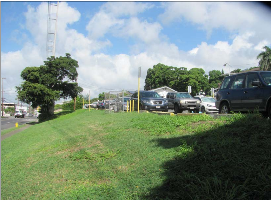
Figure 5. Construction and associated infrastructure at the northwest end of the project area, view to the north-northwest.
