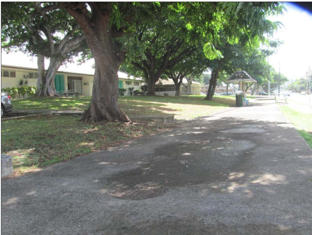
Figure 8. Grading, parking, drainage, and building construction along southwest edge of study area, view to the southeast.
