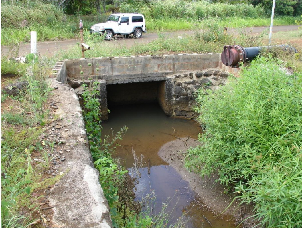
Figure 10: Box culvert on east side of Kapaia Cane Haul Road.
