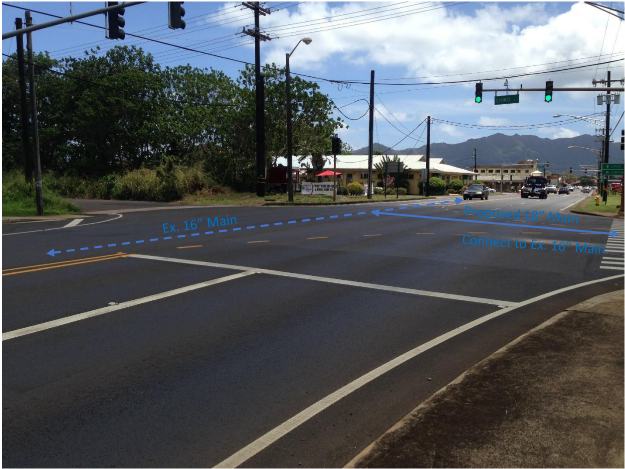
Photo #1, Kuhio Highway and Ehiku Street Intersection, Proposed 18" Main to Connect to an Existing 16" Main
