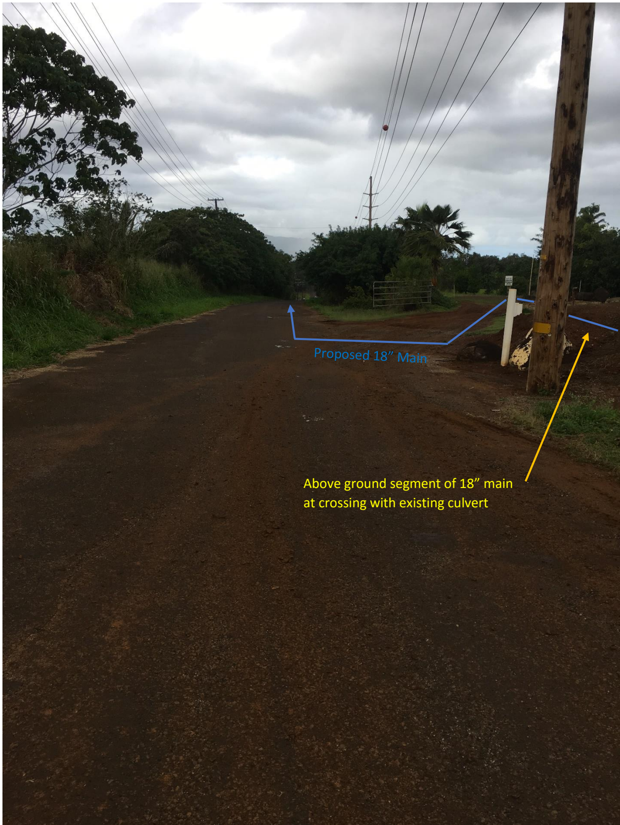
Photo #13, Haul Cane Road facing the direction of Maalo Road, Culvert Crossing
