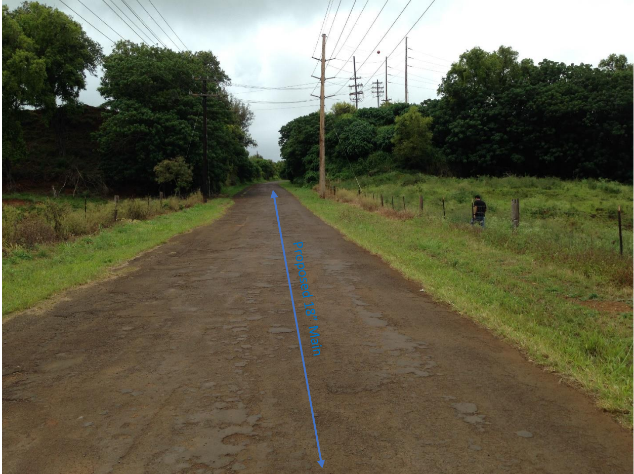
Photo #15, Haul Cane Road facing the direction of Maalo Road
