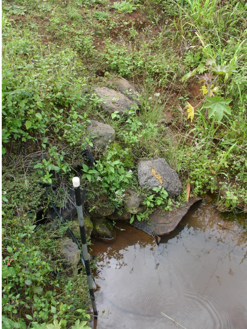
Figure 3: Metal Culvert, North Side of Kapaia Cane Haul Road
