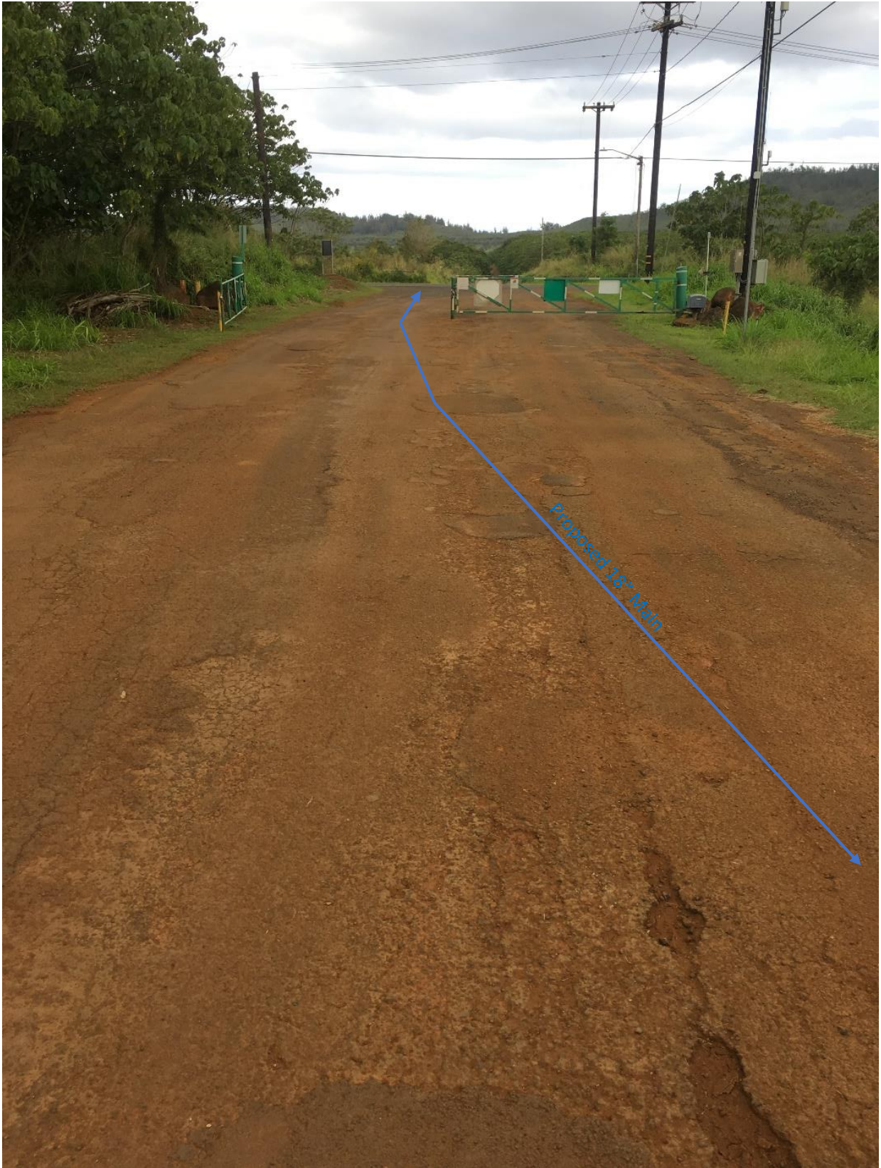
Photo #21, End of Haul Cane Road facing intersection with Maalo Road
