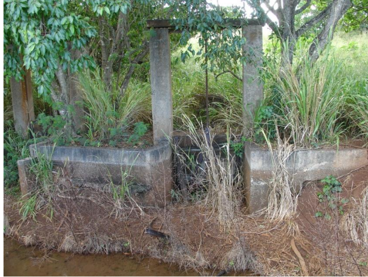
Figure 5: Water control gate on west side of the ditch.
