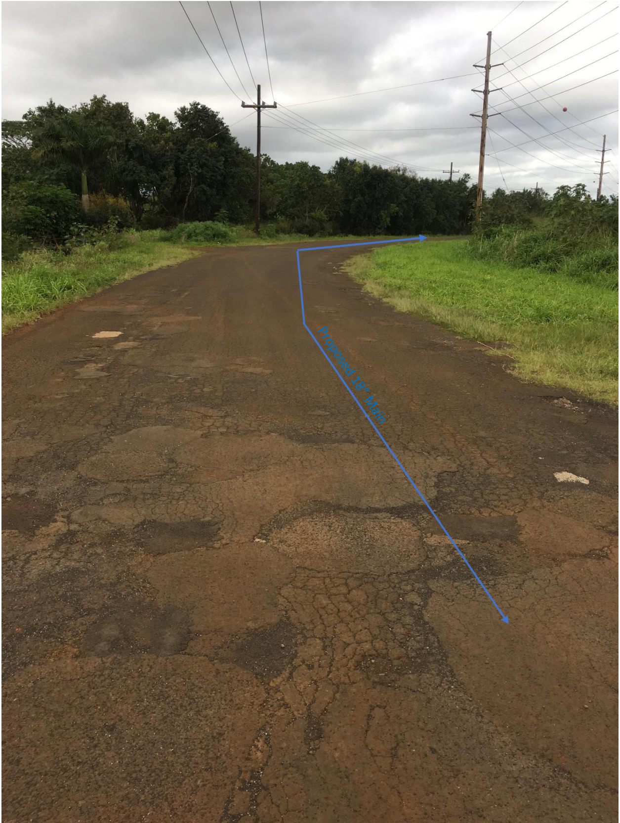
Photo #9, Haul Cane Road facing the direction of Maalo Road
