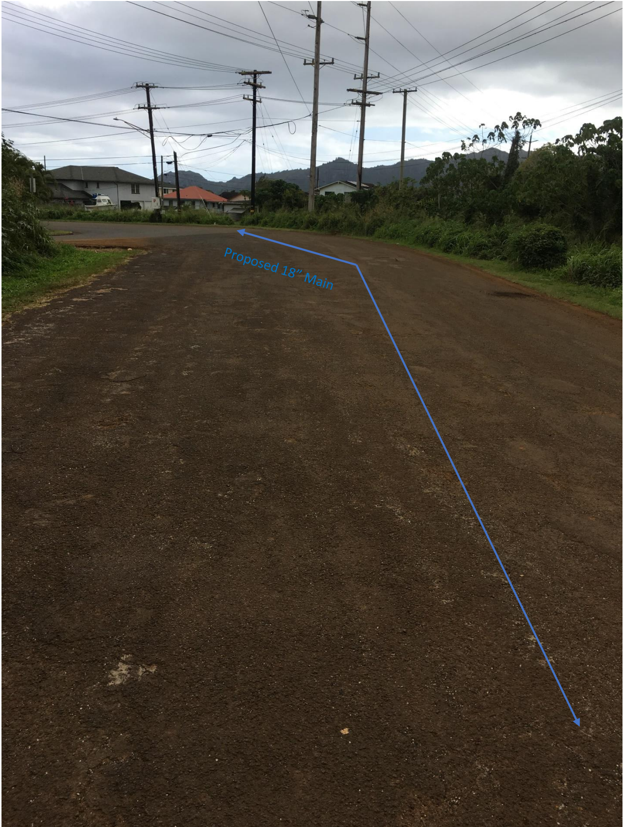
Photo #6, The beginning of Haul Cane Road facing Ehiku Street
