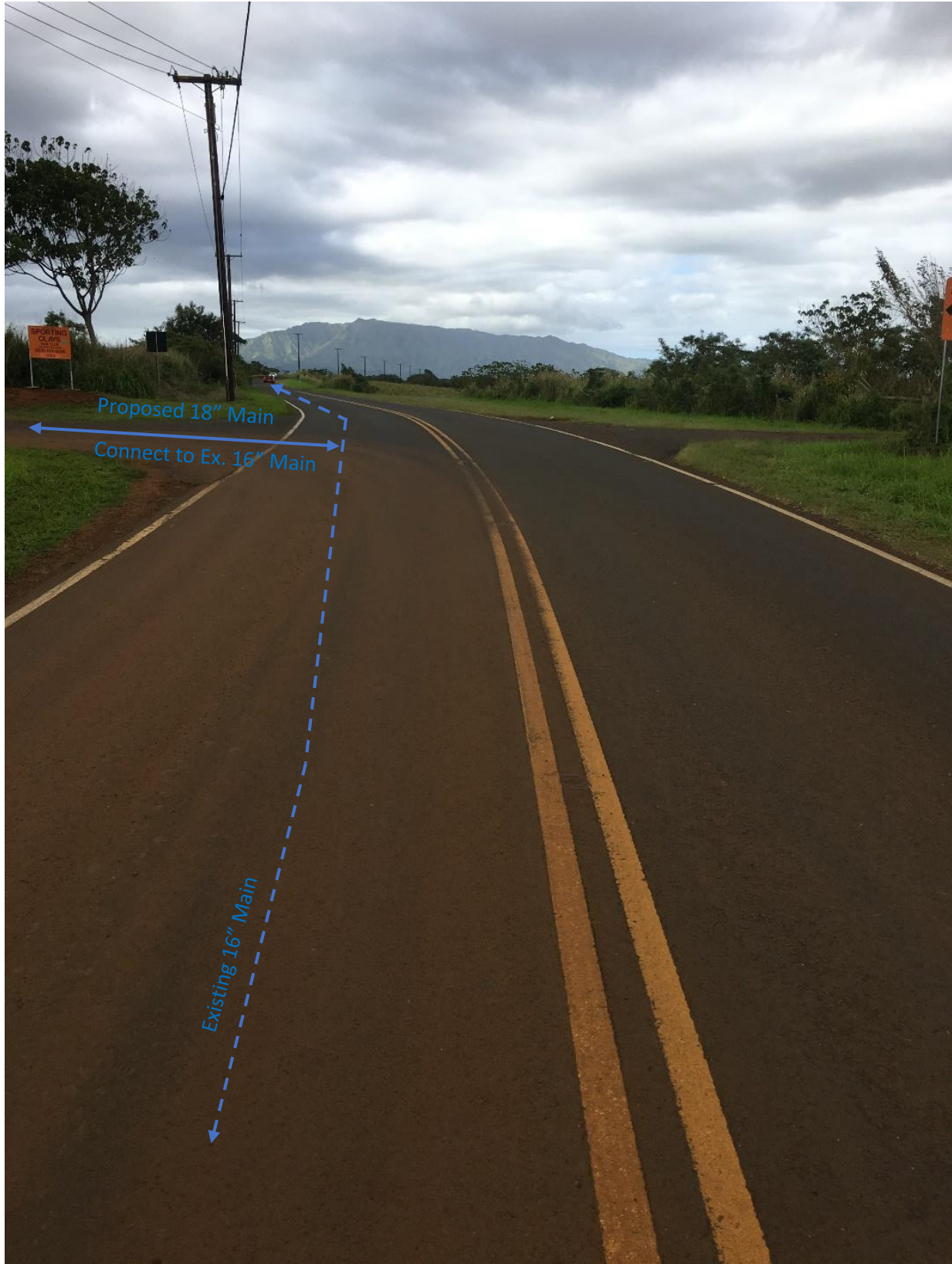
Photo #22, Maalo Road facing mauka towards intersection with Haul Cane Road
