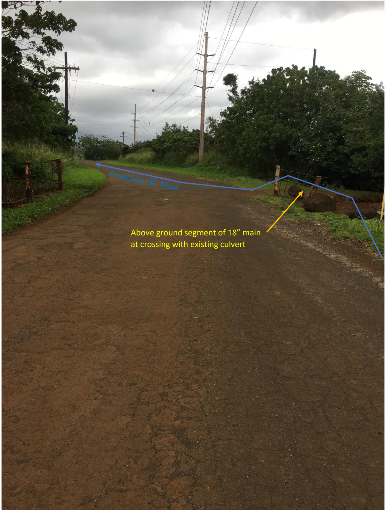
Photo #11, Haul Cane Road facing the direction of Maalo Road
