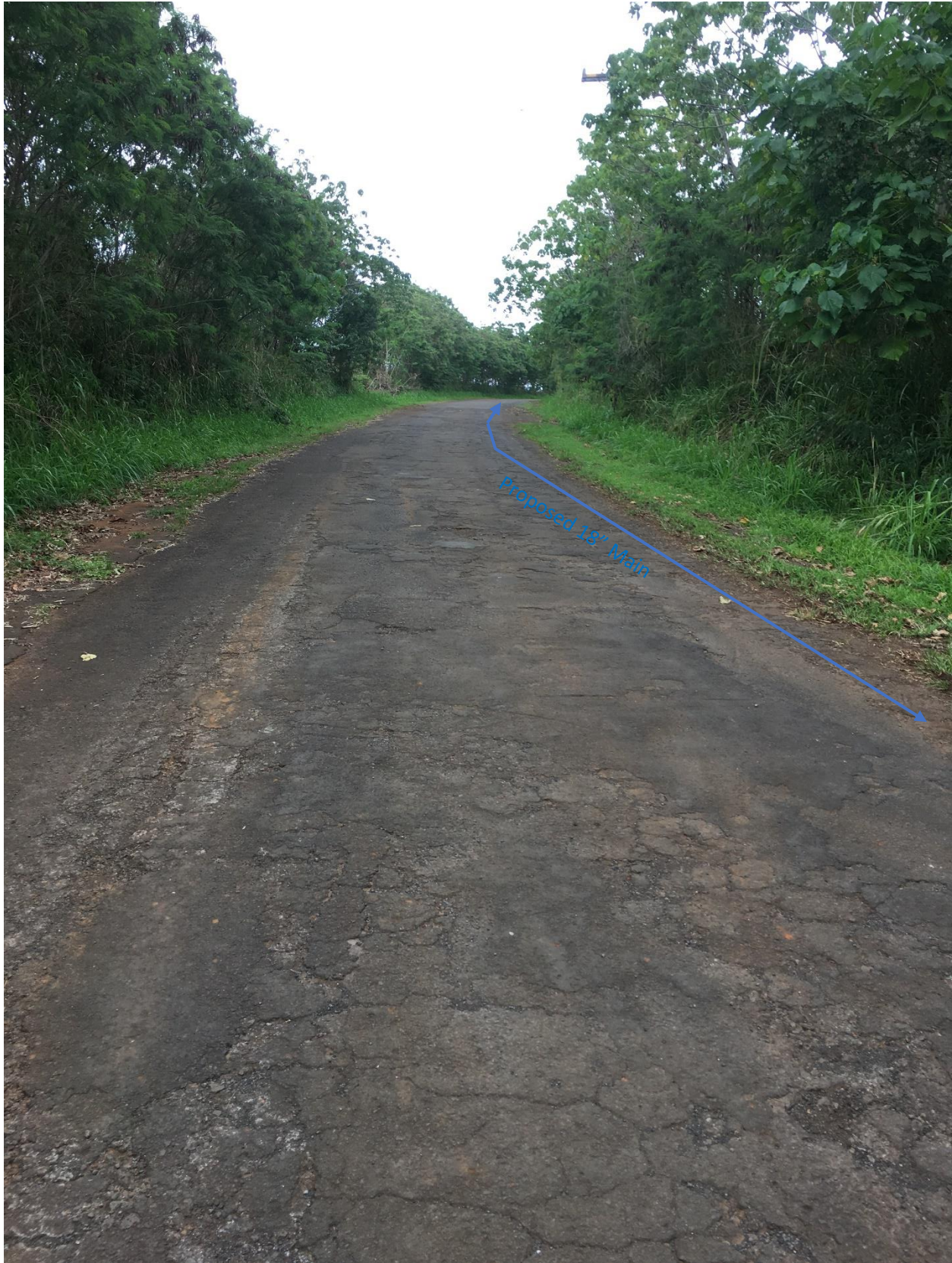
Photo #17, Haul Cane Road facing the direction of Maalo Road
