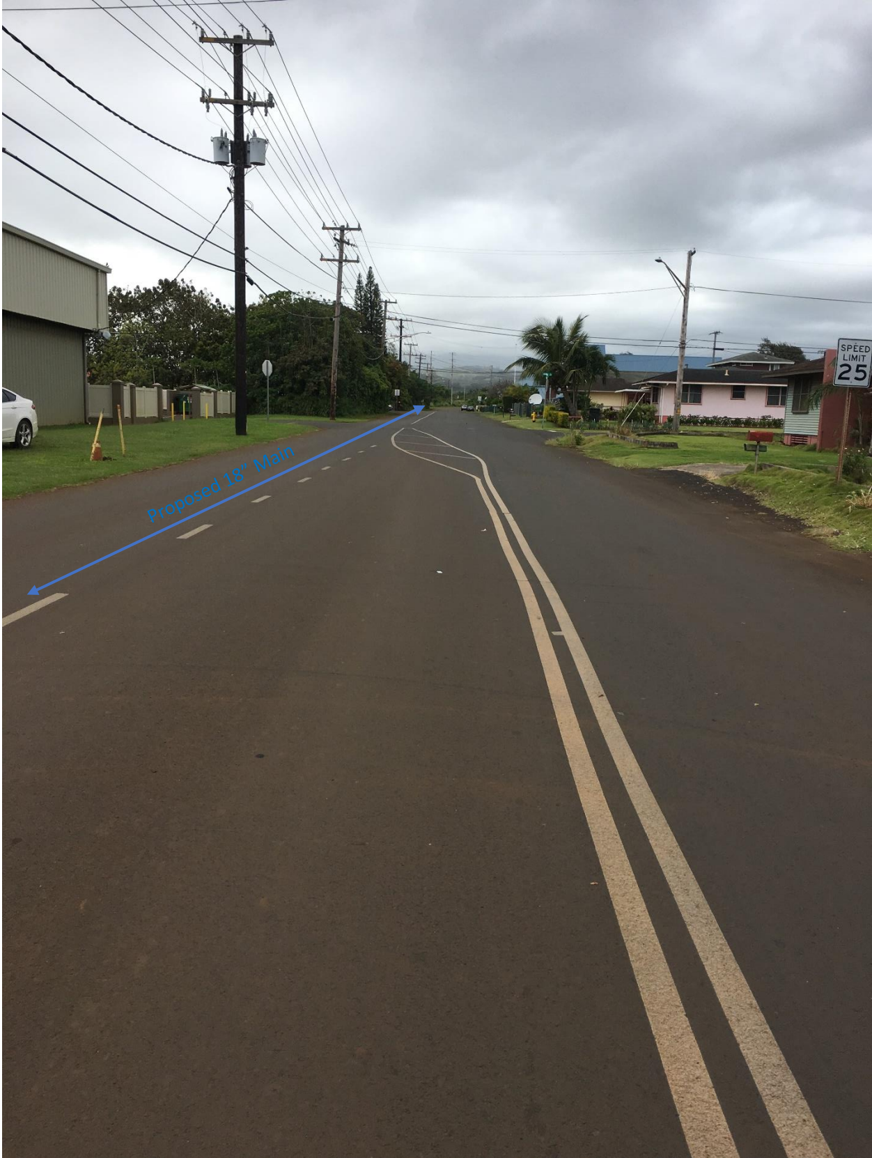
Photo #3, Ehiku Street nearby Kuhio Highway facing towards Haul Cane Road
