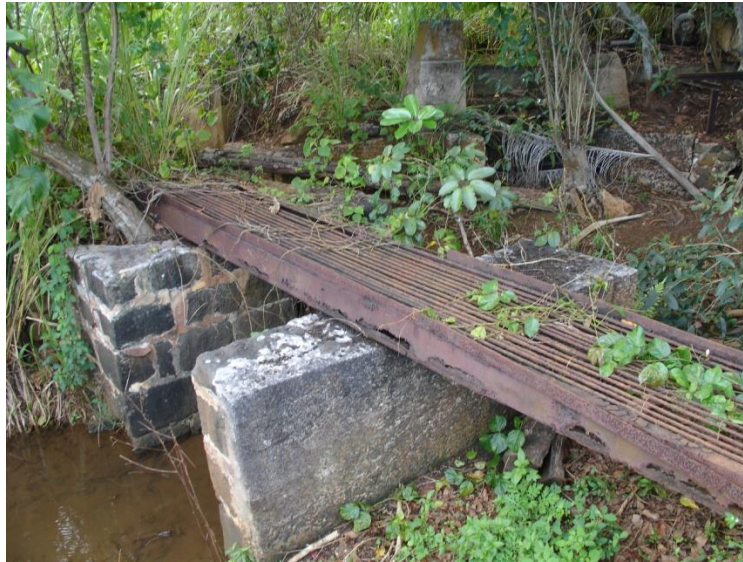
Figure 6: Railroad bridge foundation
