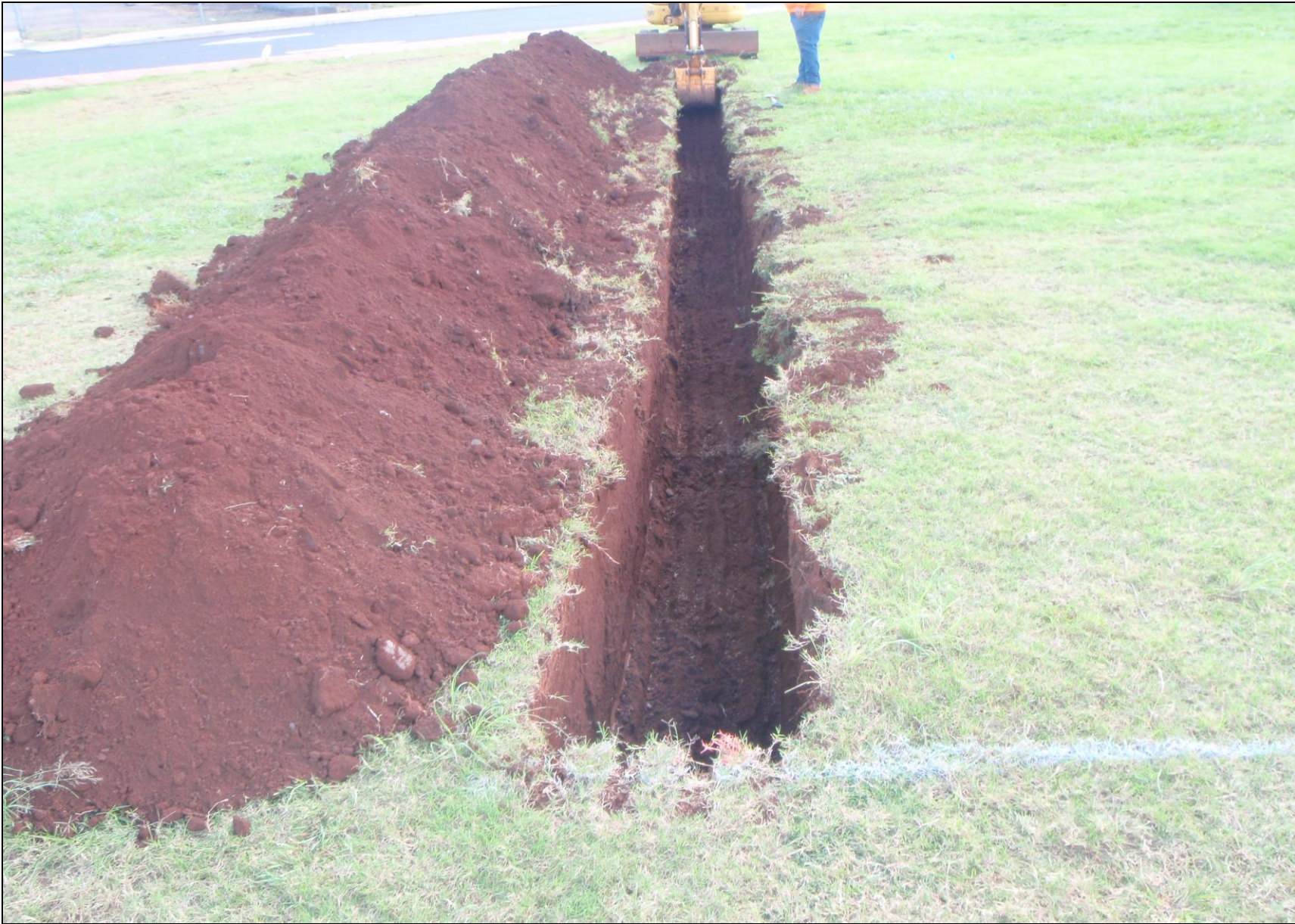
Figure 16: Photograph of TR-3, viewed to Southeast. There were no layers in TR-3, all sediment consisted of brownish black (10YR 3/2, moist) clay loam.
