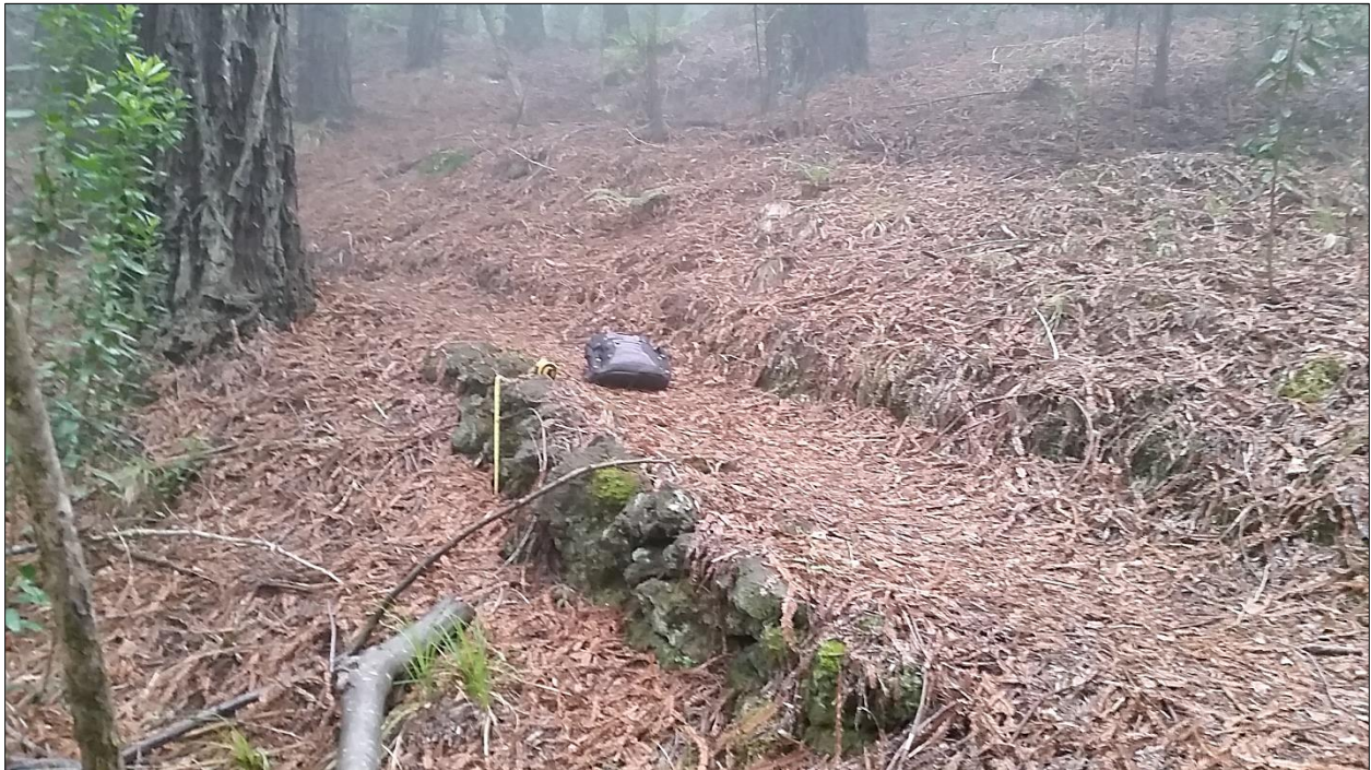
Figure 17. Small, dry-stacked, rock-retaining structure designated TCP 2 (GPS pt. 004 on the Results maps), view east
