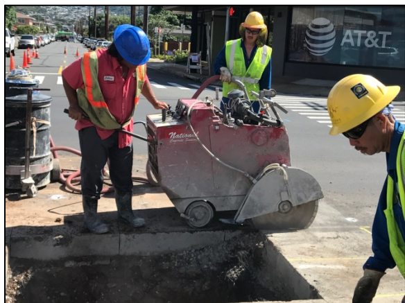
Pavement is saw-cut to prepare work area.
