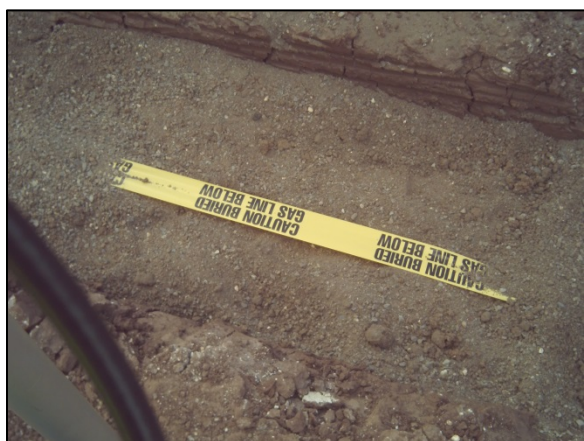
Warning tape is installed during the backfill process.
