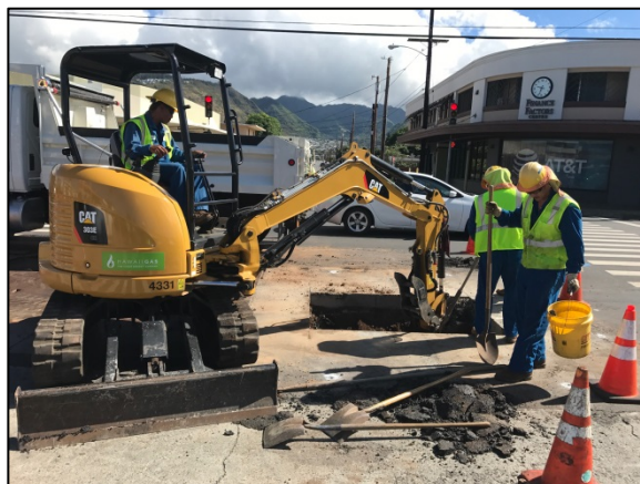
Trenching occurs with a combination of machinery and hand tools.
