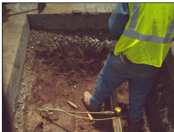
Another view of the pipeline and locator wire installation.
