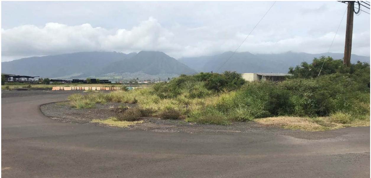
Baseyard driveway at site access road
