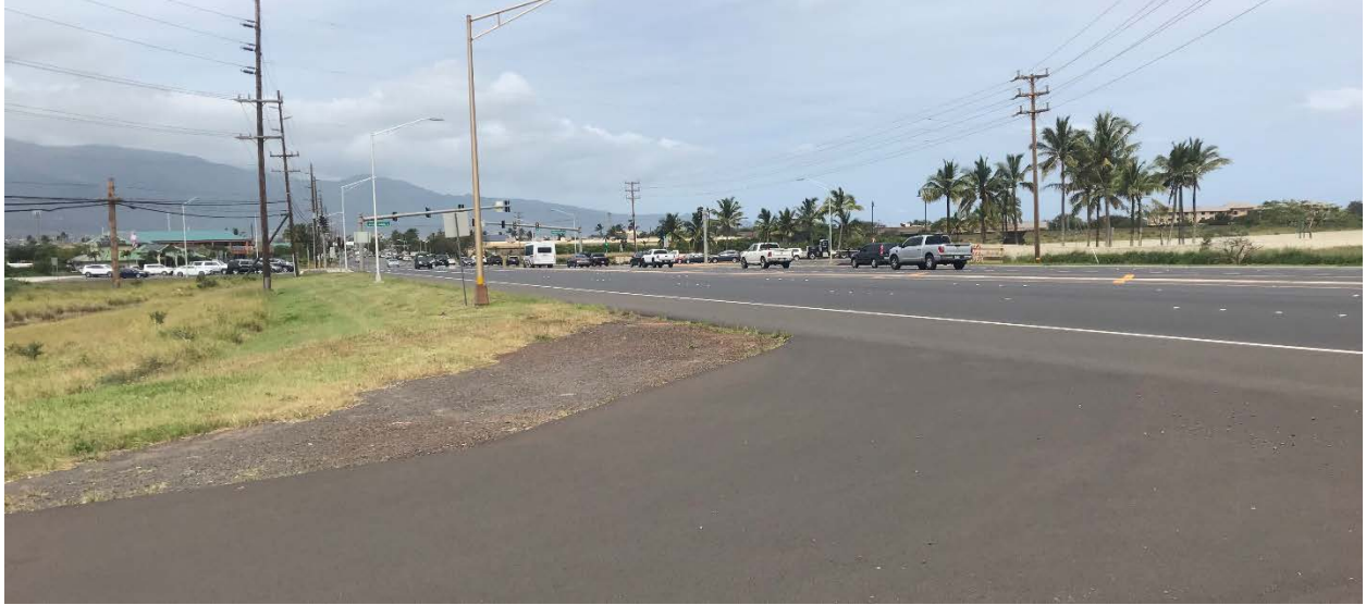
View from site access road looking west
