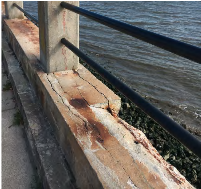
Figure L. Example End of Service Life of Sea Wall Due to Rebar Corrosion
