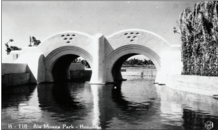
Figure 30. Art Deco style Ala Moana Equestrian Bridge understood as completed in 1934 (Hawai'i State Archives n.d.)
