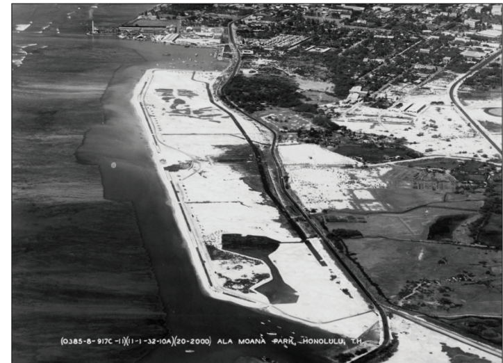
Figure 23. 1932 photograph of former reef area filled with dredged material to create Ala Moana Regional Park (Hawai'i State Archives 1932)
