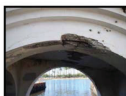
Severe spalling with missing concrete and exposed rebar at underside of bridge
