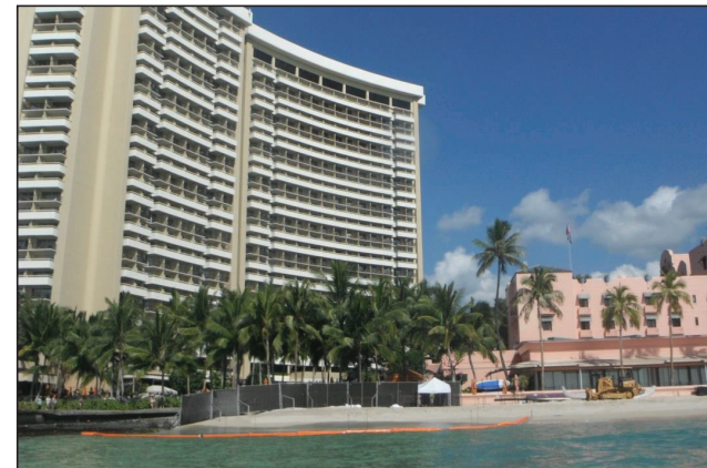
Figure 7-12 Example: floating silt curtain and small bulldozer used for sand placement in the 2012 Waikiki Beach Maintenance project.
