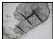
Severe spalling with missing concrete and exposed rebar at underside of bridge
