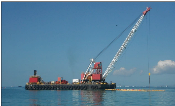
Figure 7-7 Healy Tibbitts Crane Barge used in the 2012 Waikiki Beach Maintenance Project
