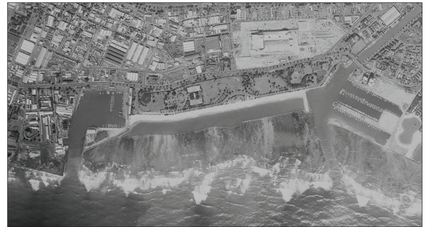
Figure 50. 1959 aerial photograph of Ala Moana Regional Park, with wide beach and swimming area; swimming area blocked from access to Kewalo Basin (left) by peninsula of fill land and from Ala Moana Yacht Harbor (right) by a jetty (UH SOEST 2012c)
