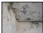
Moisture infiltration at underside of the Ewa side of the bridge has loosened plaster and paint
