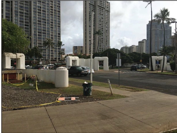
Figure 60. Roosevelt Portal, northeast corner of the park, view to northeast
