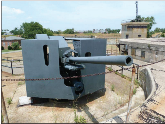
Figure 41. Typical AMTB Battery with 90 mm gun (Fort Monroe, Virginia) (Fort Wiki 2015)
