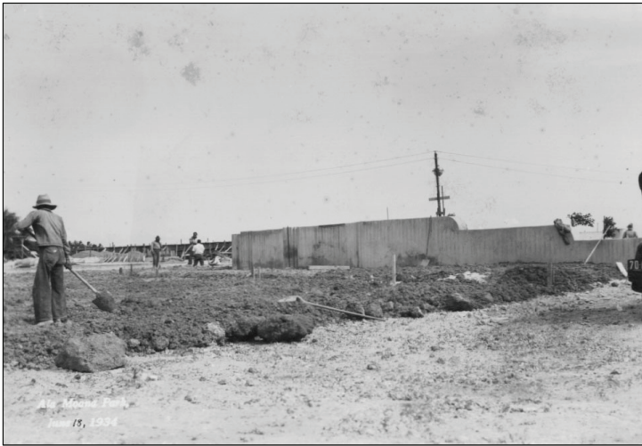
Figure 32. 1935 photographs showing dredged material and topsoil stockpiled and spread on new fill land of Ala Moana Regional Park (Hawai'i State Archives 1935b)
