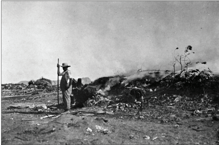
Figure 17. Open-air burning of trash in area between Kewalo Basin and Ala Moana Regional Park, 1921 photograph (Hill 1921, reprinted in Scott 1968:578)
