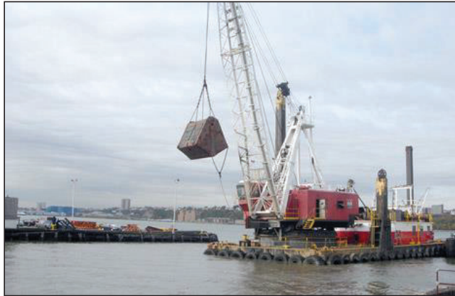
Figure 7-2 Example: Clamshell Dredge with Environmental Bucket ( http://www.conedison.com/ehs/2009annualreport/environmental_stewardship )
