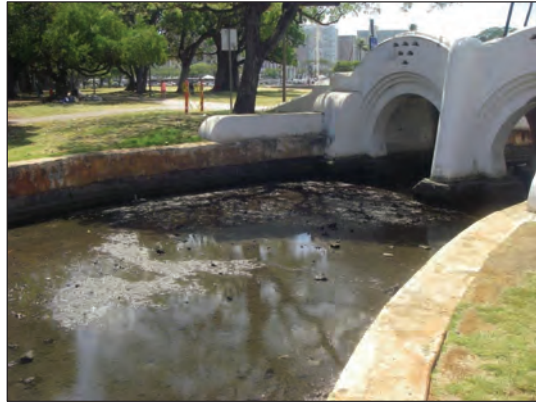
Figure 8. Partly dry canal at the easement bridge.
