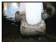
Moisture infiltration at underside of the Ewa side of the bridge has loosened plaster and paint
