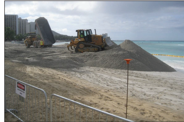
Figure 7-11 Sand placement, 2012 Waikiki Beach Maintenance Project.
