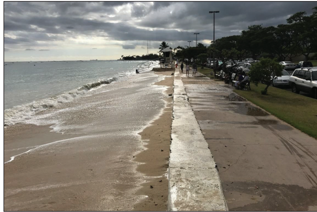
Figure 2-20 Inundation of beach area near Tower 1C (May 26, 2017)
