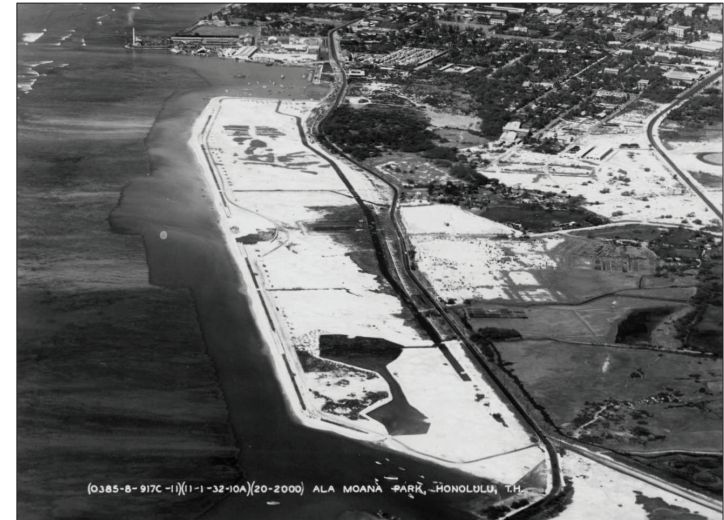
Figure 25. 1932 photograph of former reef area filled with dredged material to create Ala Moana Regional Park (Hawai'i State Archives 1932)
