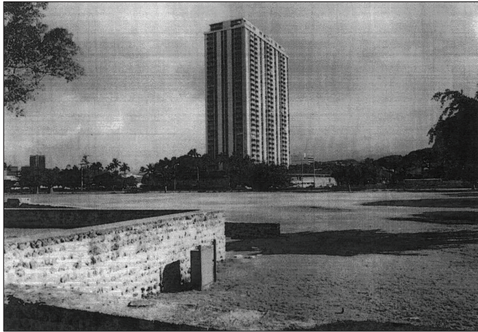
Figure 37. Boulder walls in the park, bare (upper) and stuccoed (lower) (photographs by Robert R. Weyeneth in Weyeneth 1987)
