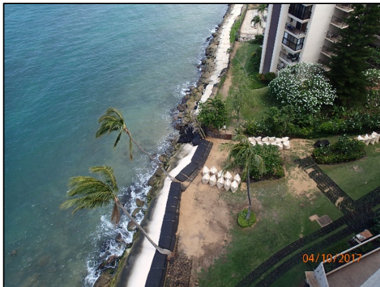
Photo #4 (4/10/17): Geotextile sandbags fronting the Royal Kahana and Hololani Condominium looking south.
