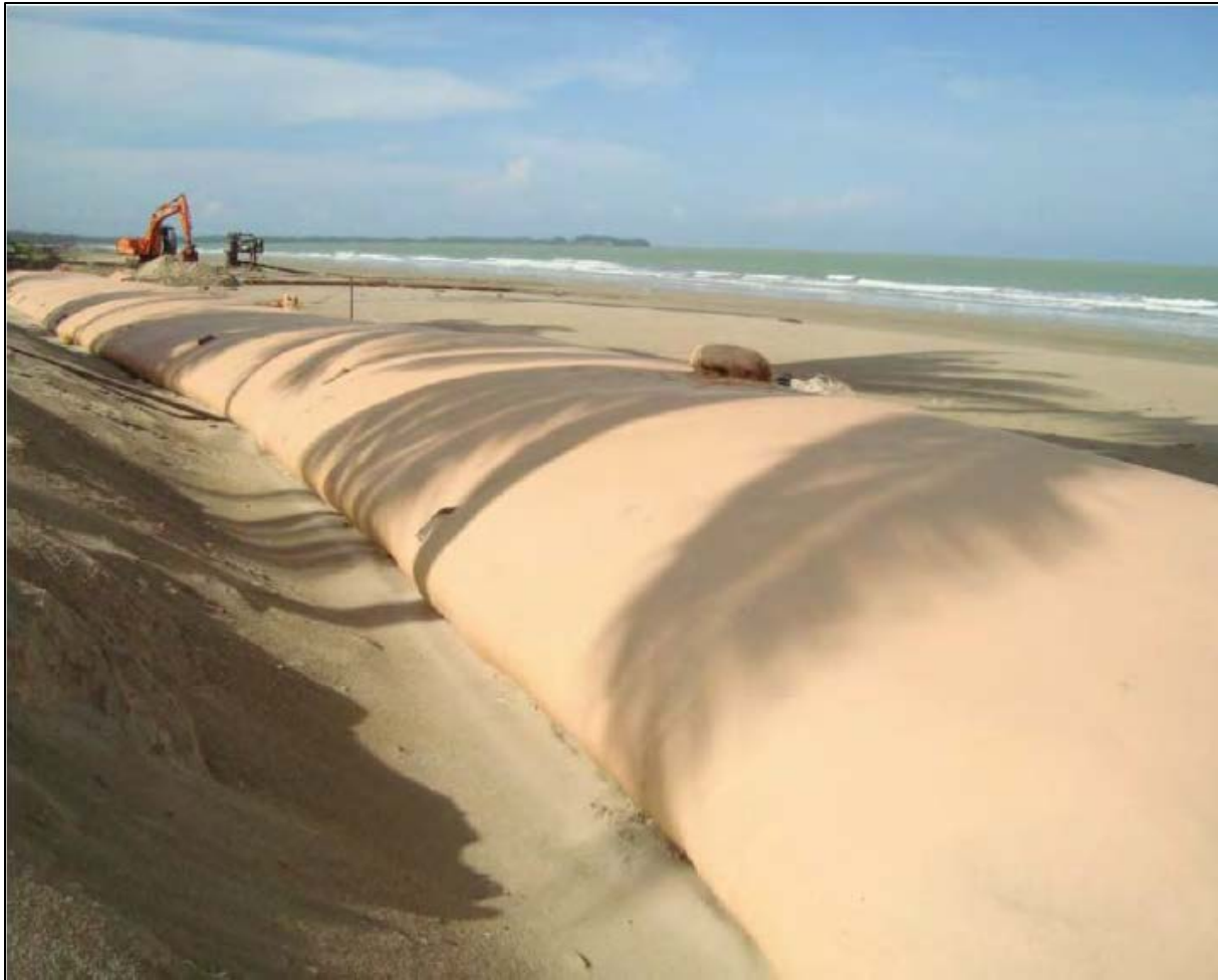
Figure 2-4: Geotube Use in Beach Nourishment Projects
