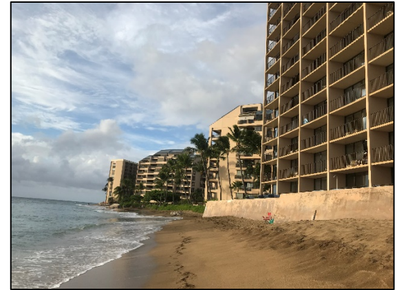
Photo #12 (7/13/18): Looking north at the seawall fronting the Kahana Beach Resort.
