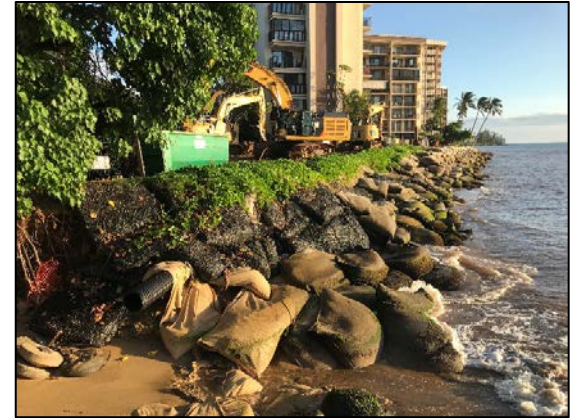
Photo #3 (9/20/18): Hololani sheetpile installation and geotextile containers looking south.
