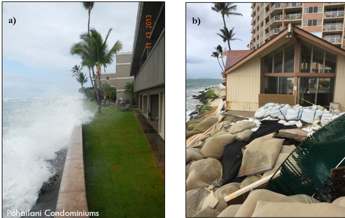
Figure 1-5: (a) Wave Overtopping a Seawall Fronting the Pohailani Condominium, (b) Resulting Damage Following a Storm Event
