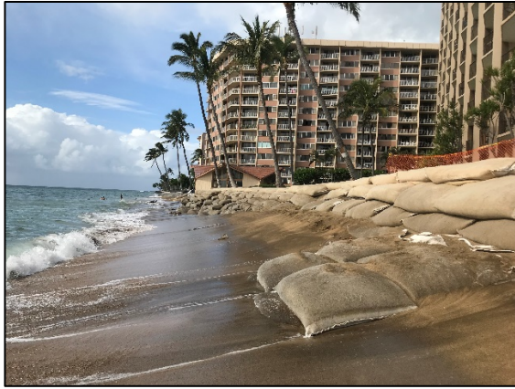
Photo #7 (7/13/18): Looking north at geotextile shoreline protection at Valley Isle Resort.
