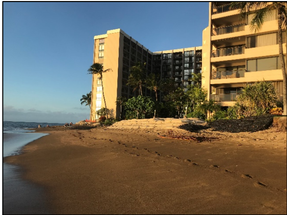
Photo #10 (9/20/18): Looking north at geotextile shoreline protection at Sands of Kahana.
