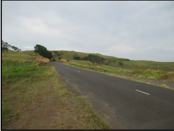
Photograph 1. A view of Old Mamalahoa Highway from the subject property, facing west (05 February 2018).
