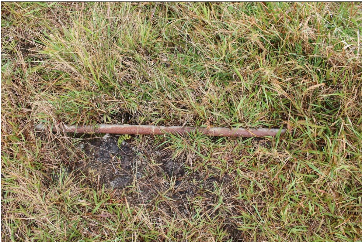
Figure 15. Remnant 1-inch galvanized steel waterline, overview.
