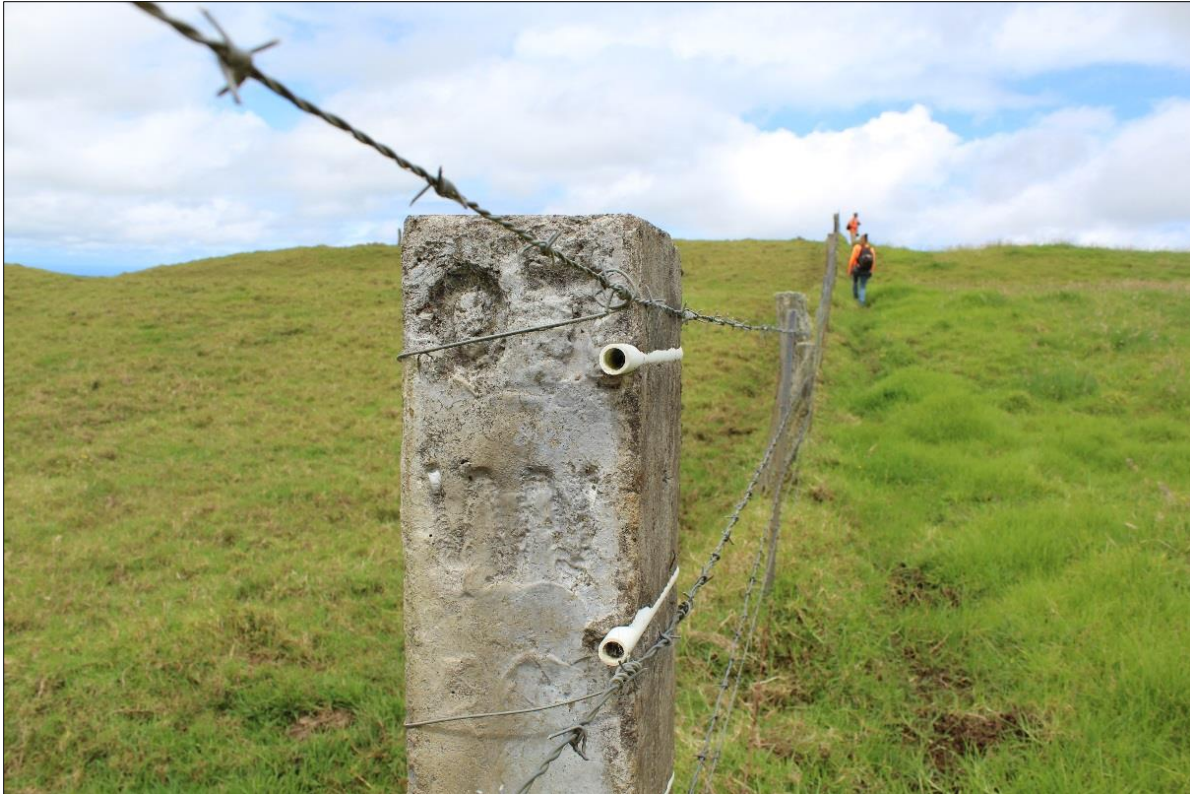
Figure 20. Concrete fence post with embedded PVC pipe and inscription reading “07” and unidentifiable brand, view to the north.
