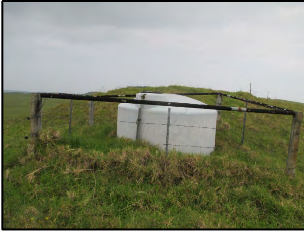
Photograph 28. A view of the 400-gallon water tank observed on the subject property. The water tank was serviced by a private waterline that enters the subject property from the south (05 February 2018).
