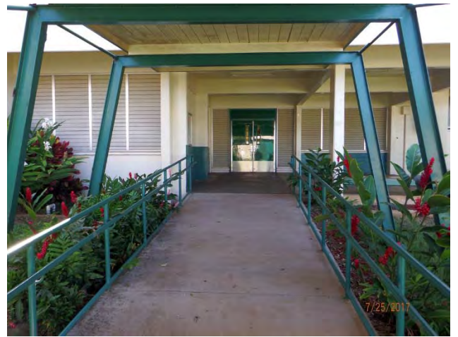
4. Existing library entrance and covered entrance ramp. (View to east)
