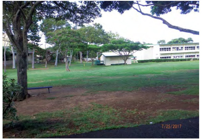
10. Site of proposed library with Building PO-1 and Building B in background. (View to south)
