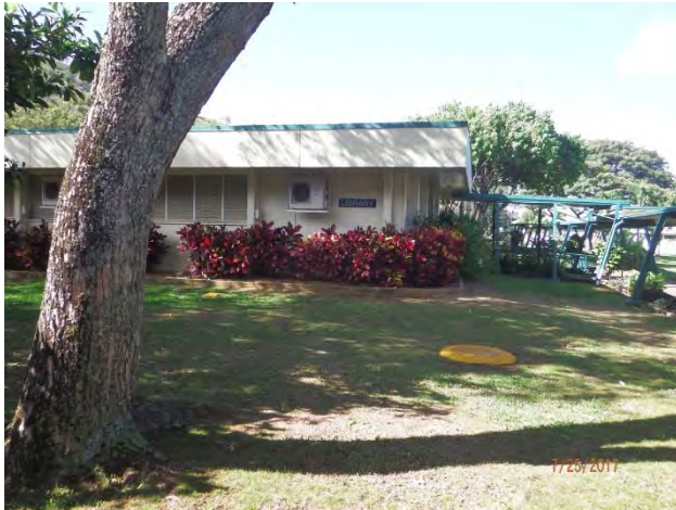
3. Existing library with covered entrance ramp on right. (View to south).
