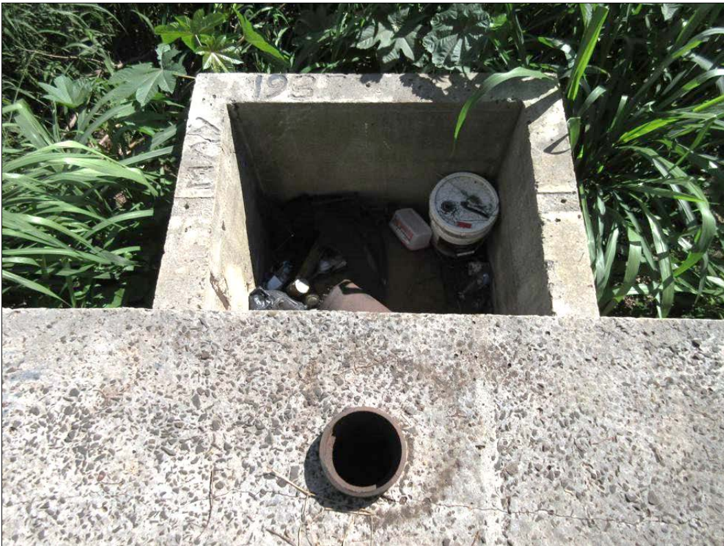
Figure 76. Site 8778 Feature D pipe and basin filled with debris; note "MAY 1937" inscribed on basin walls.
