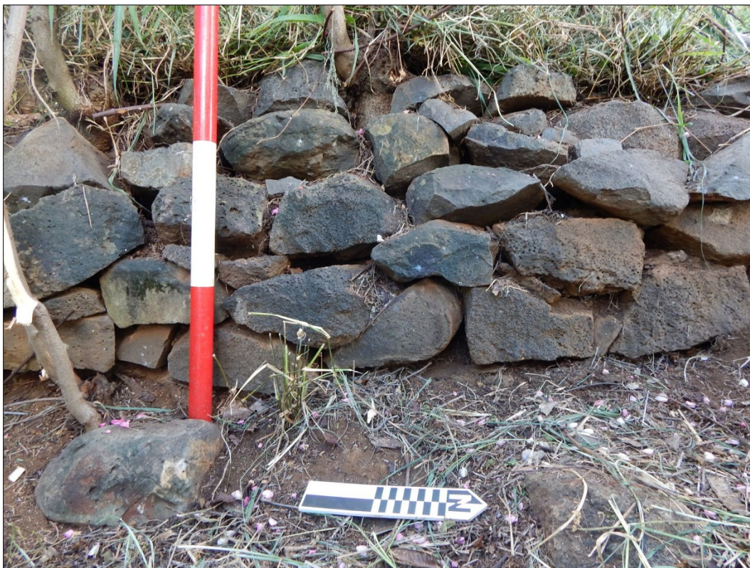
Figure 64. Dry-stacked rock retaining wall at southern end of Site 8778 Subfeature C1, view to the west.
