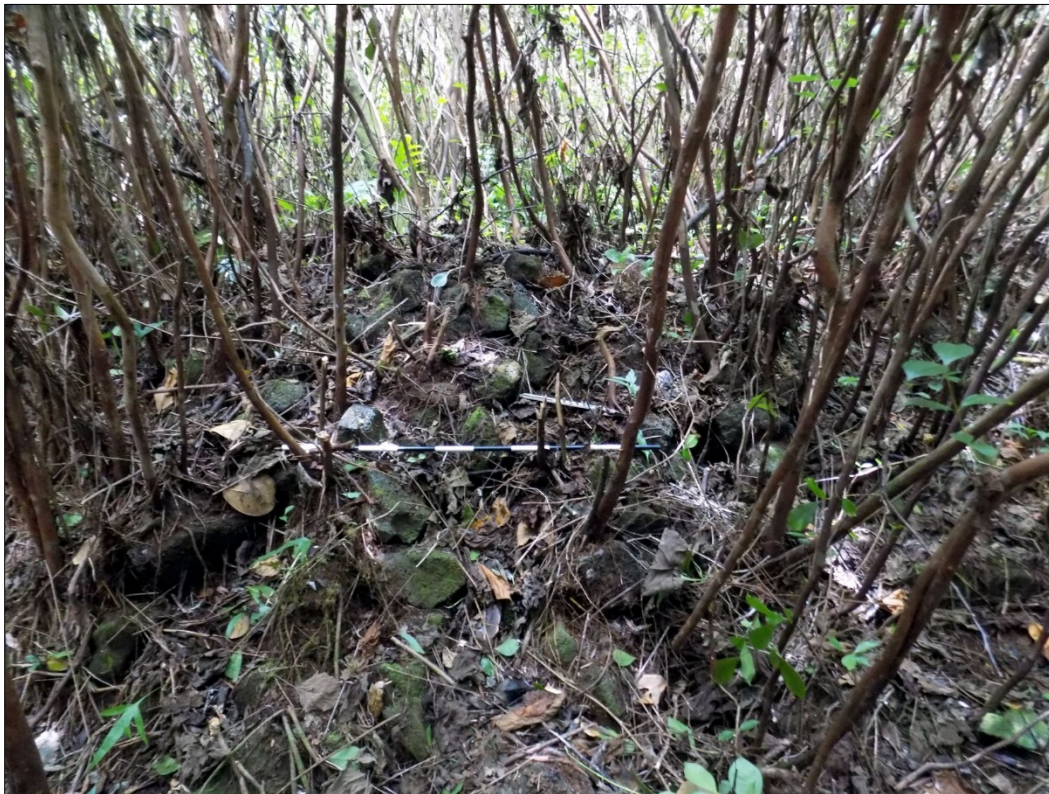
Figure 53. Site 30712 Feature 15 wall, view to the east.
