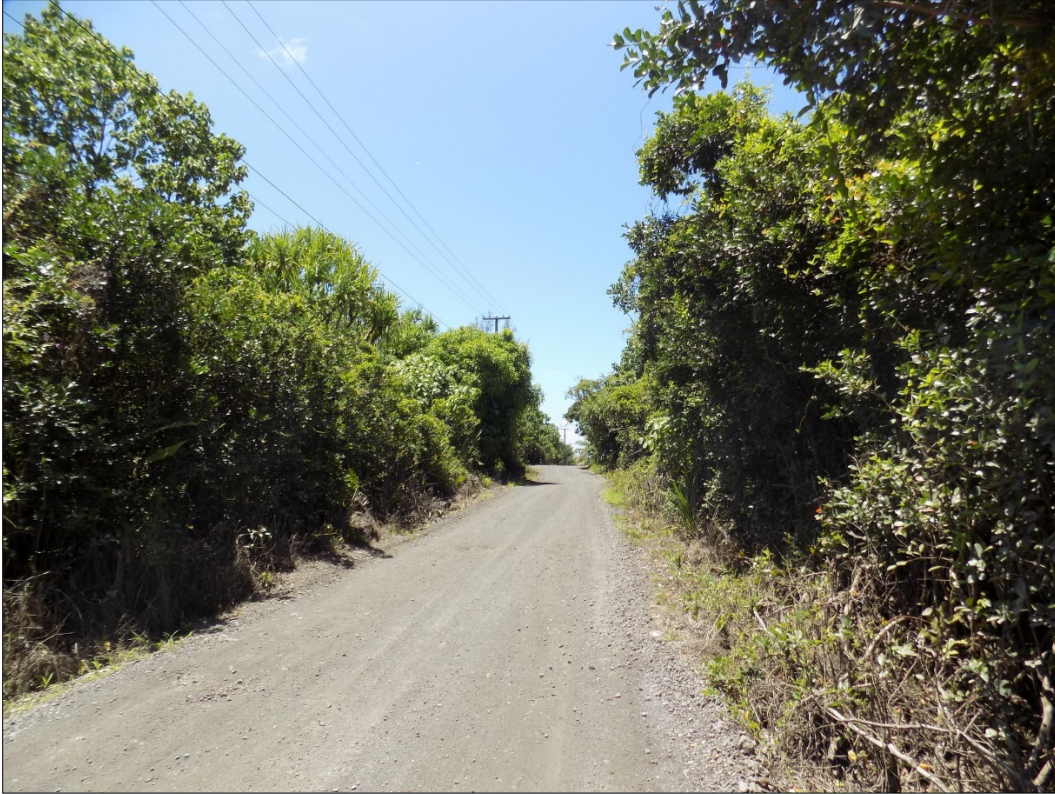
Figure 6. Old Government Road on the mauka boundary of the study area, view to the northwest.
