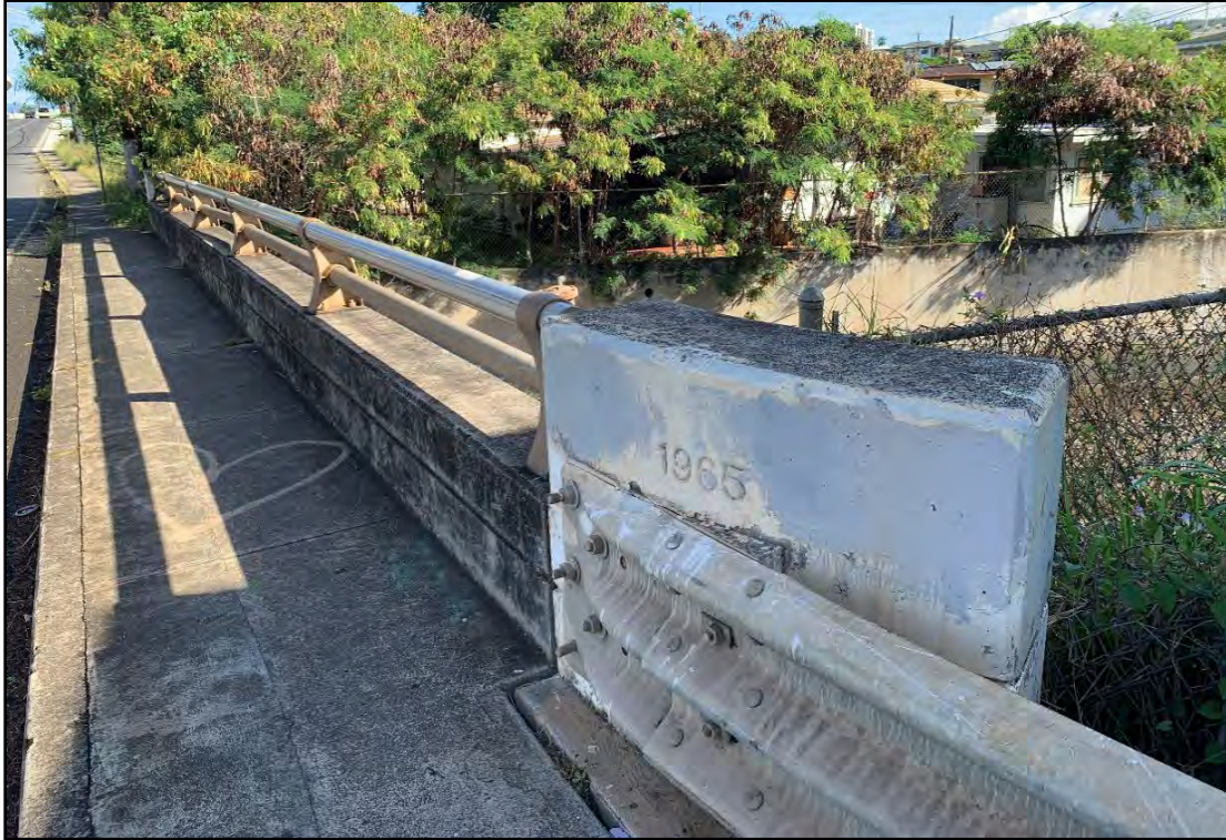
Figure 160. CSH 57, 'Aiea Stream Bridge, view to north
