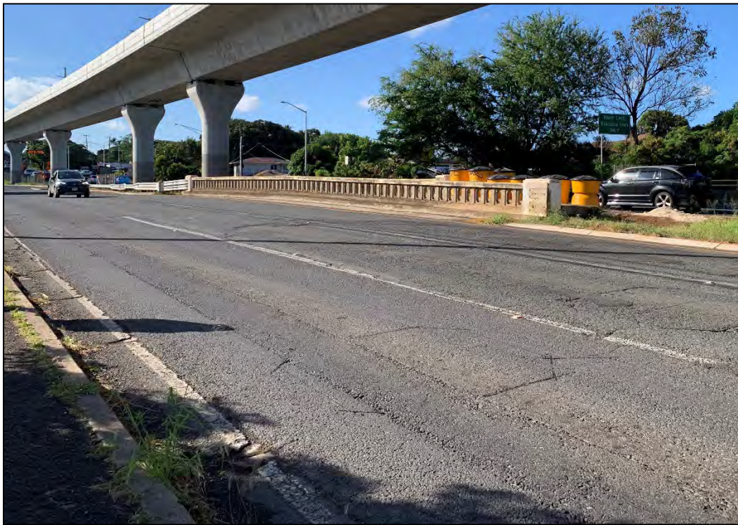
Figure 159. CSH 56, Kalauao Stream Bridge, view to south
