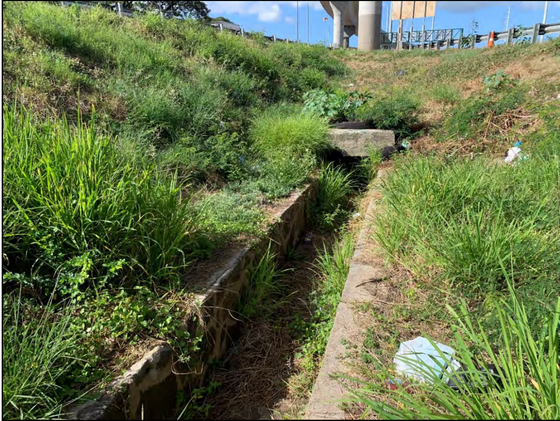
Figure 162. CSH 59, culvert and drainage channel, view to south
