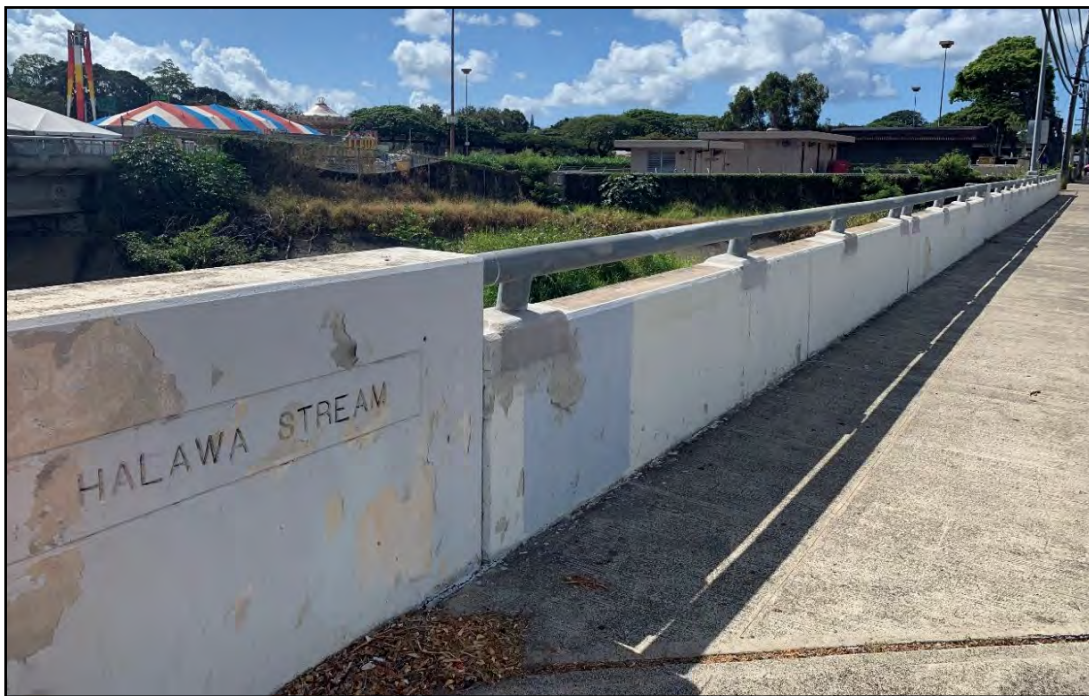
Figure 163. CSH 60, Salt Lake Boulevard Bridge–Hālawa Stream, view to southeast
