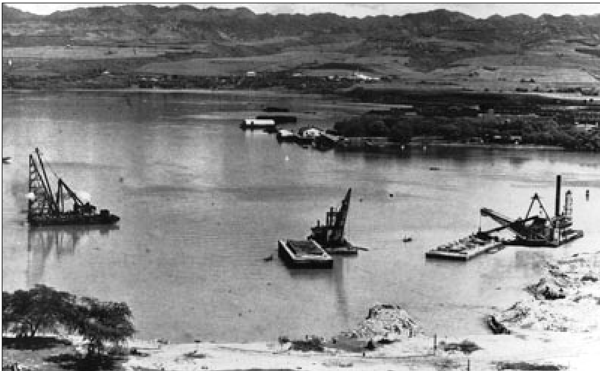
Figure 49. Dredging in Pearl Harbor ca. 1908 (Hawai'i State Archives)
