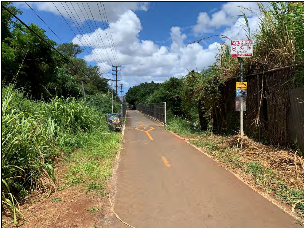
Figure 105. SIHP # 50-80-12-9714, OR&L spur steel bridge in Waikele Ahupua'a, view to east
