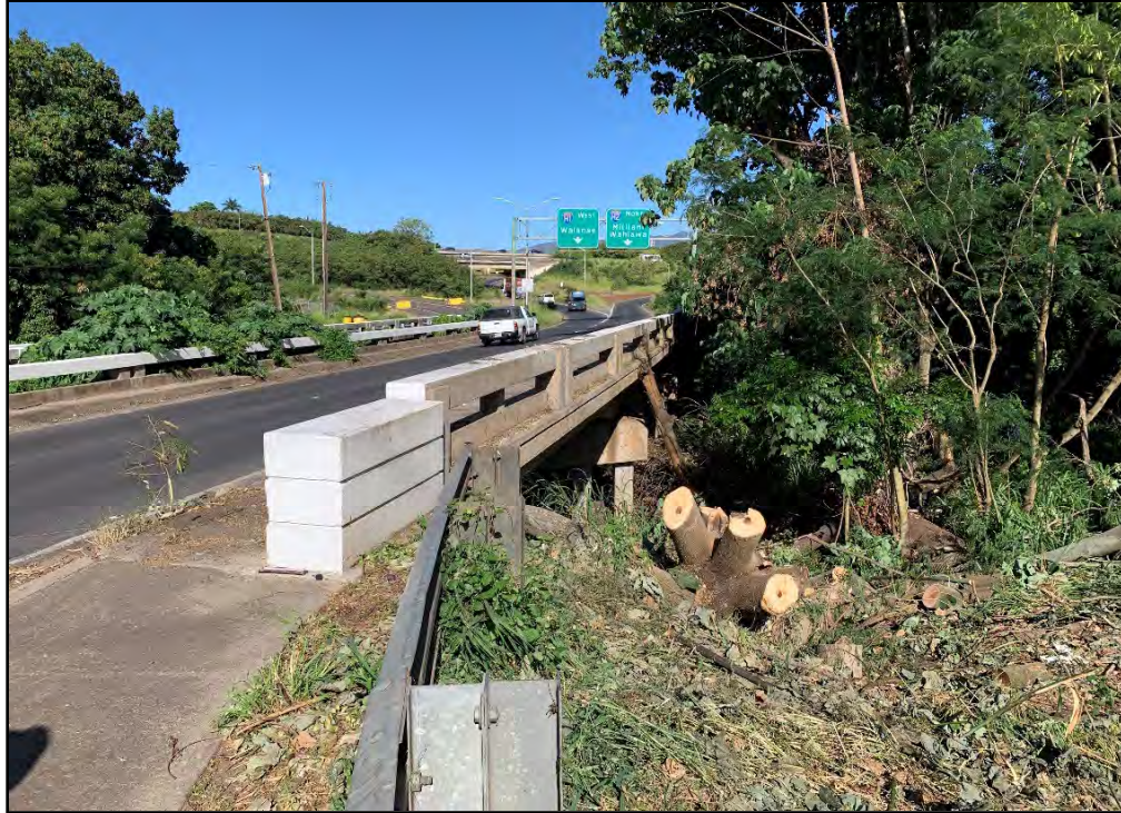
Figure 140. CSH 48, Waiawa Stream Bridge, view to west
