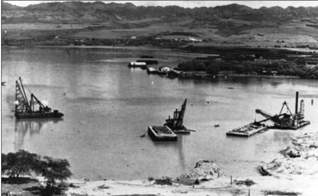
Figure 54. Dredging in Pearl Harbor ca. 1908 (Hawai'i State Archives)
