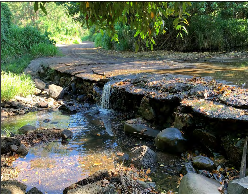
Figure 141. CSH 49, Waiawa Stream Culvert, view to northwest
