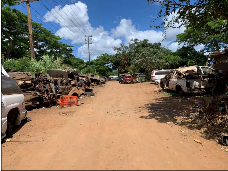
Figure 136. General view of the study area within Mānana Ahupua‘a, west of the existing Pearl City WWPS and adjacent to the Pearl Harbor Bike Path, showing dump sites along an unimproved road and surrounding undeveloped areas, view to west
