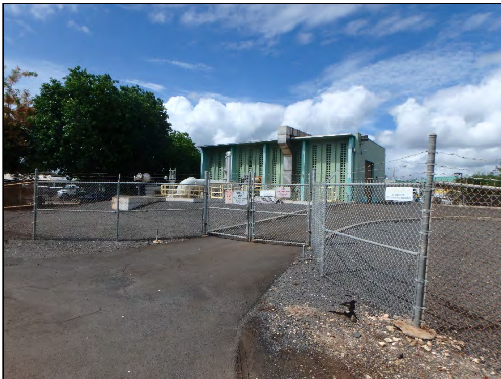
Figure 97. General view of the Waipahu WWPS and alternate areas, view to east
