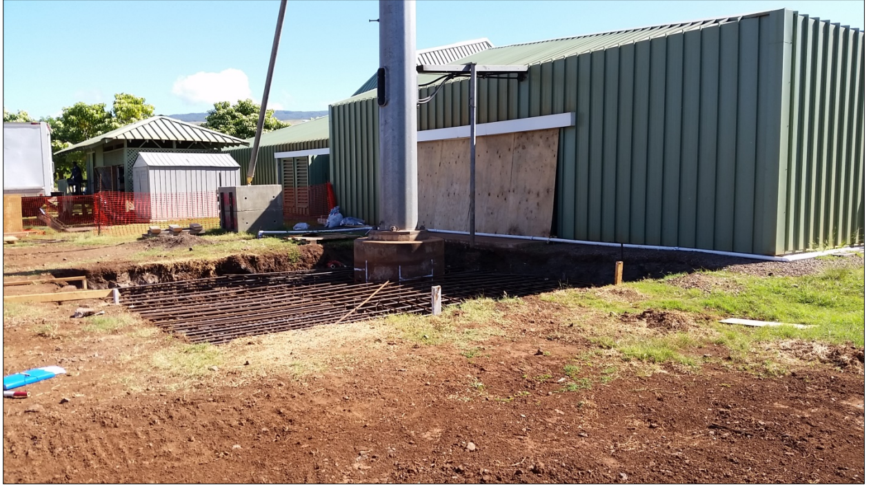
Figure 5. Location of large, square-shaped excavation around (and deeper than) existing cell tower and smaller (old) footing; view northeast
