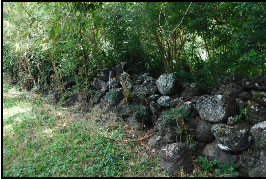
Figure 26. Feature 10.1 wall (view to southeast)
