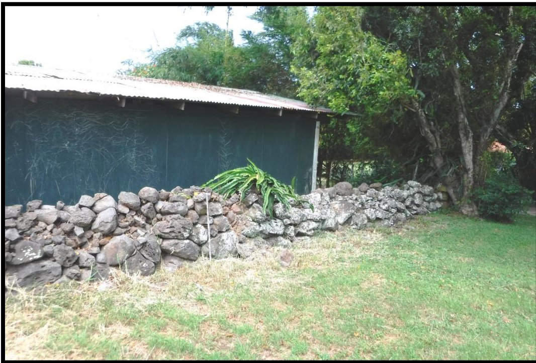
Figure 25. Modern shed built over historic Feature 7 concrete slab showing Feature 10.1 wall (view to north)
