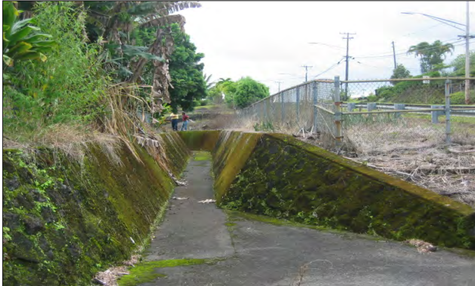
Figure 25. Palai Stream C looking upstream at stormwater ditch on HaiHai St.
