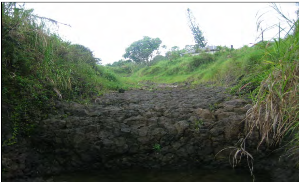
Figure 8. Waiakea Stream looking upstream from rock outcropping Approximate Stream Station 17+001.00
