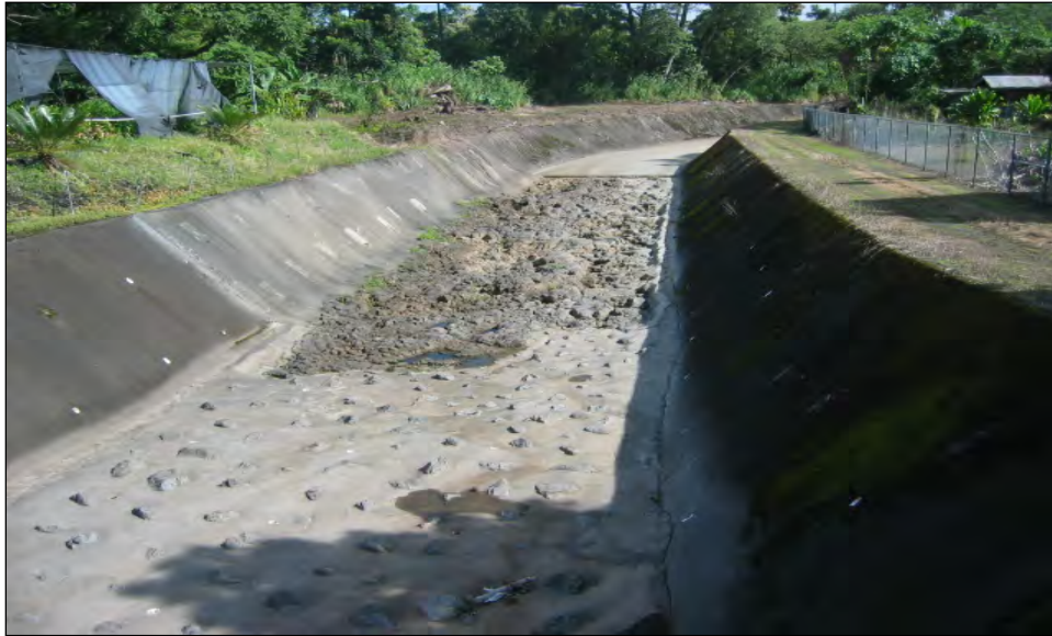
Figure 17. Waiakea Stream looking downstream from the T. Shiroma Bridge
