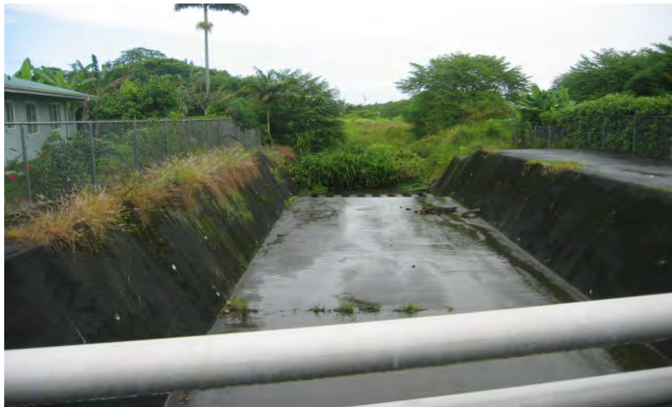
Figure 30. Palai Stream looking downstream from Heahea St Bridge
