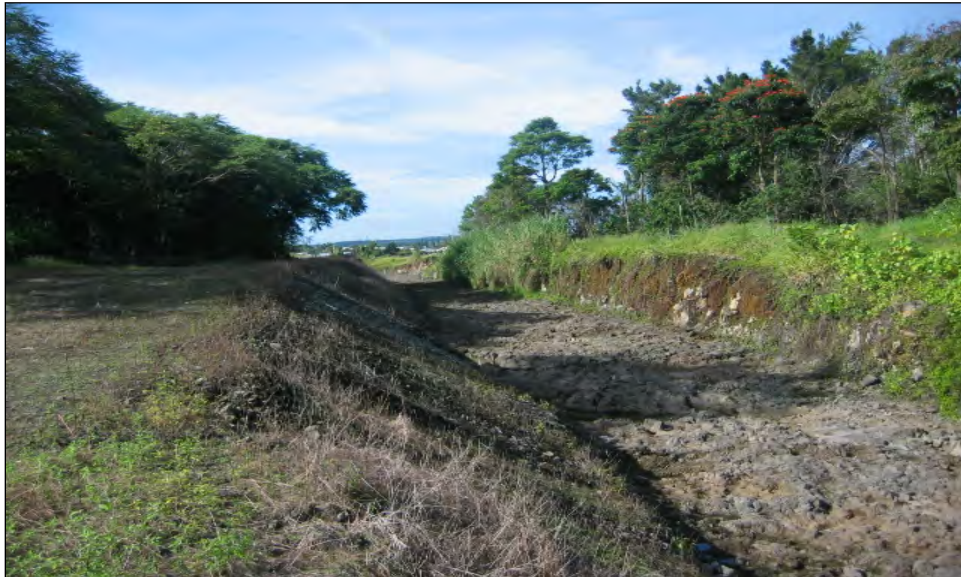
Figure 14. Waiakea Stream looking upstream from the upstream end of Waiakea-Uka channel
