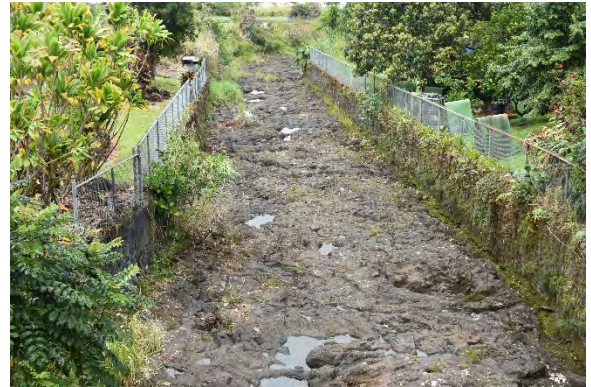
Fig. 6. Site 2 – Waiakea Stream at Kupulau Road bridge, looking downstream.
