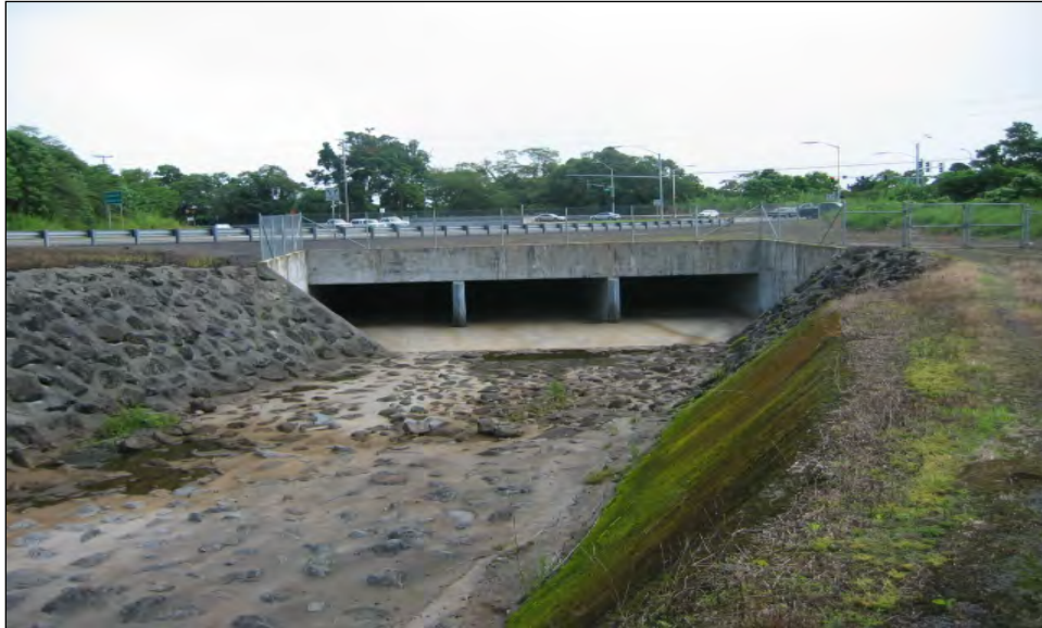
Figure 19. Waiakea Stream looking downstream at upstream face of Puainako St Bridge
