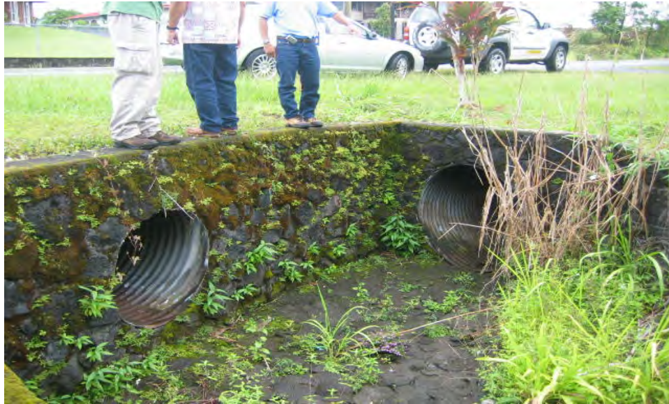
Figure 29. Palai stream looking at HaiHai St culvert
