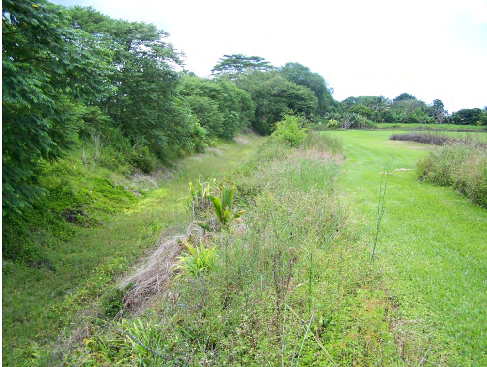
Figure 39. Eastern bank of the Kupulau Ditch within the New Hope Church property (view north).
