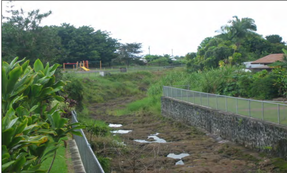
Figure 7. Waiakea Stream looking downstream from Kupulau Rd Bridge at Station 20+219.90
