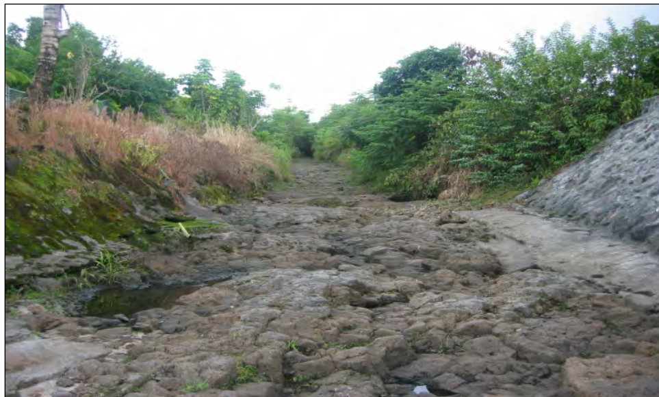
Figure 10. Waiakea Stream looking upstream from the end of the channel lining near Kawailani St
