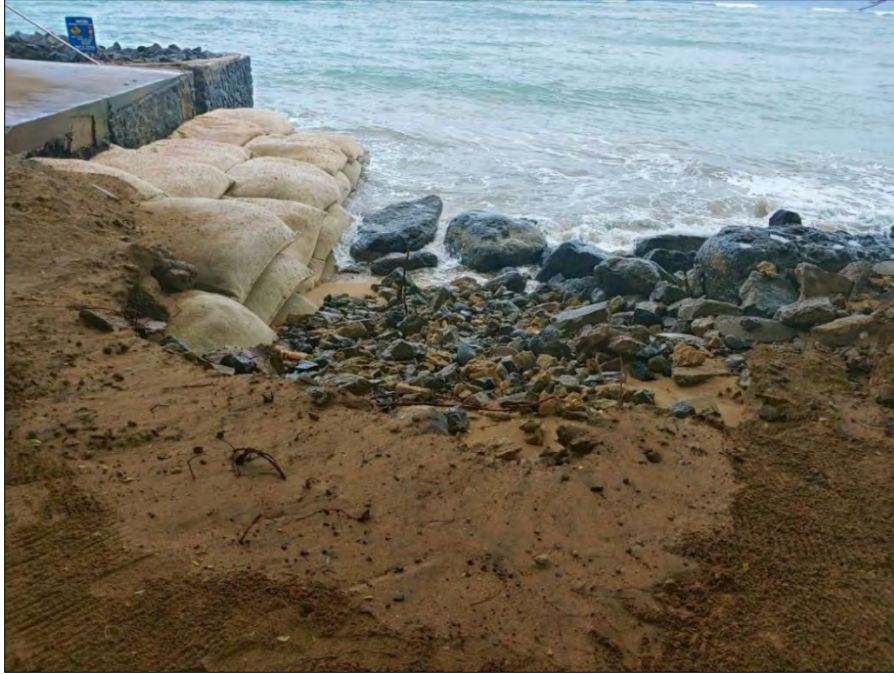
Figure 38. Coastal erosion at the Sadang property. Notice the difference from the previous figures. Trees and cement are gone and now sandbags are present (Courtesy of Mr. Felimon Sadang)
