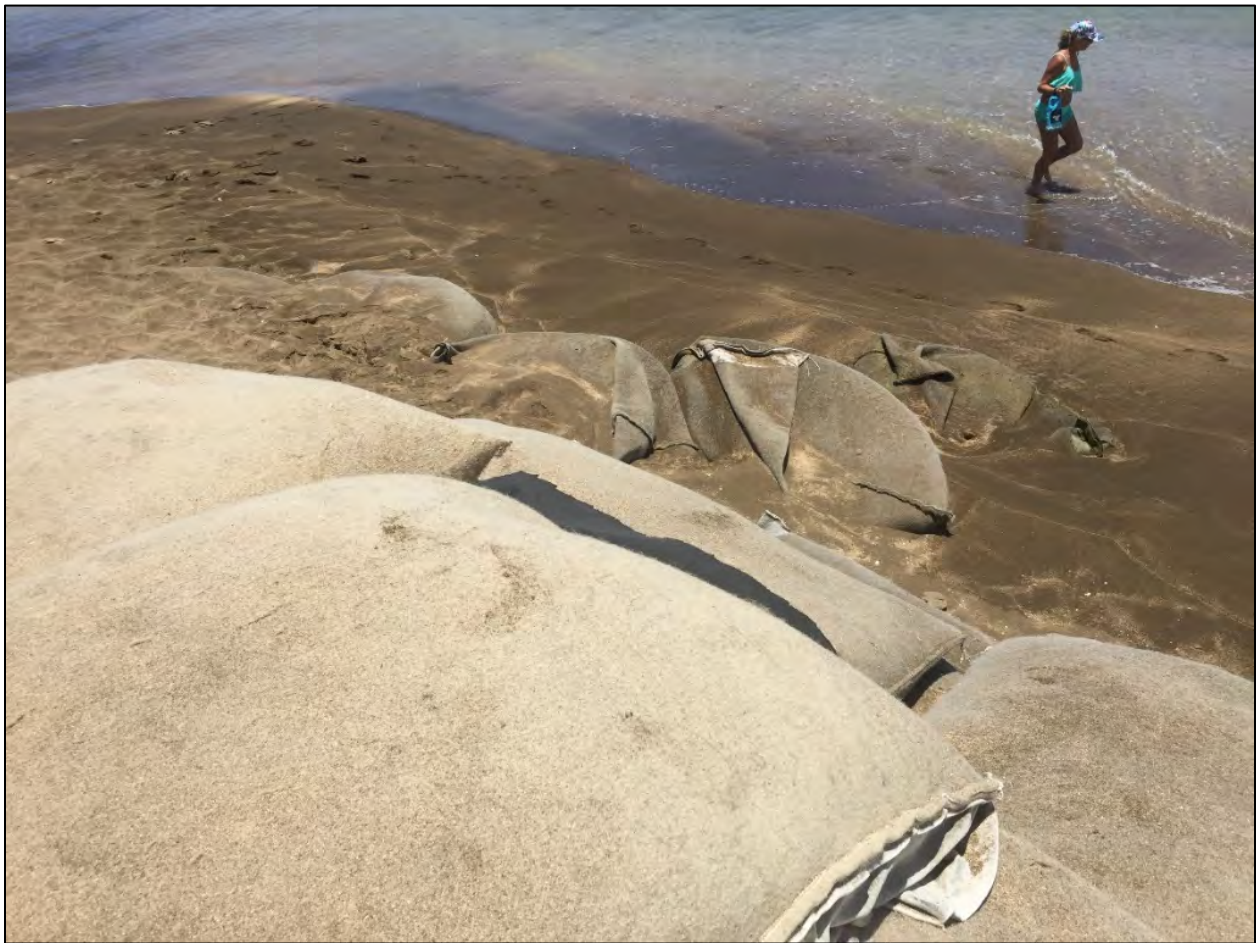
Figure 23. Large sand bags on the shore (CSH 2019)
