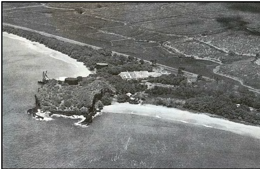
Figure 14. Aerial photo of Pu'u Keka'a with storage tanks and loading cranes visible, ca. 1940 (photo reproduced from "Dynasty in the Pacific" by Frederick Simpich, Jr., 1974)
