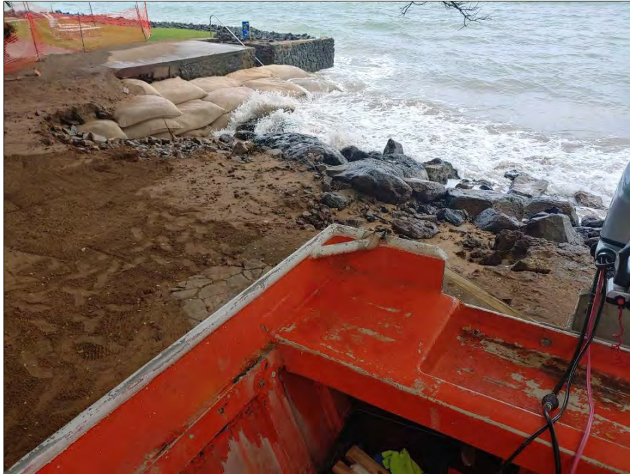
Figure 46. Coastal erosion at the Sadang property (Courtesy of Mr. Felimon Sadang)
