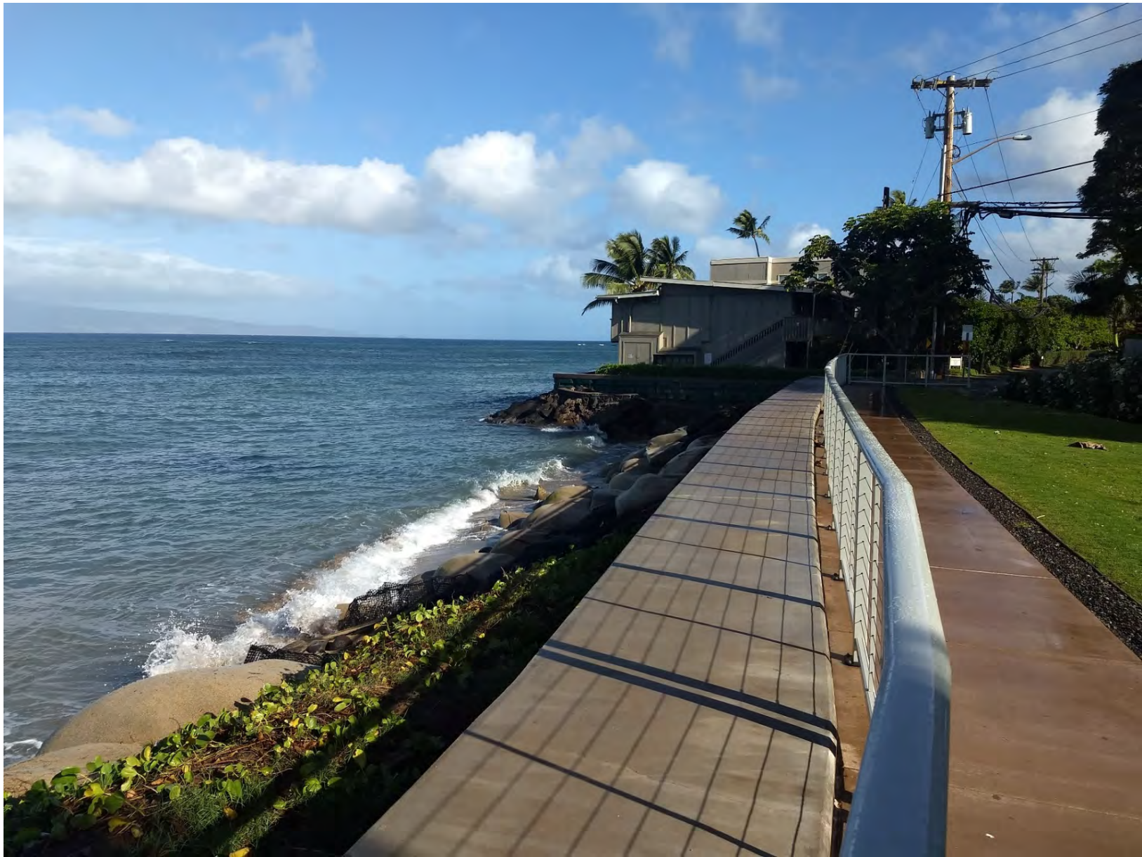
Figure 12: Coastal Photographic View of a Path in Front of the Seaward Facing Portion of the Hololani Resort and the Pohailani. Note the Sandbags Along the Shoreline. View to the North.
