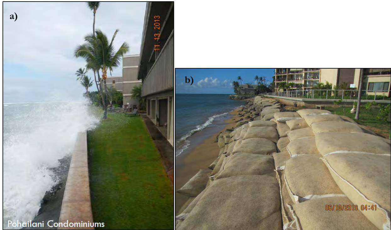
Figure 1-6: a) Wave overtopping a seawall fronting the Pohailani Condominium in 2013; b) Emergency geotextile structures along the Royal Kahana and Hololani shorelines, photo taken June 2019
