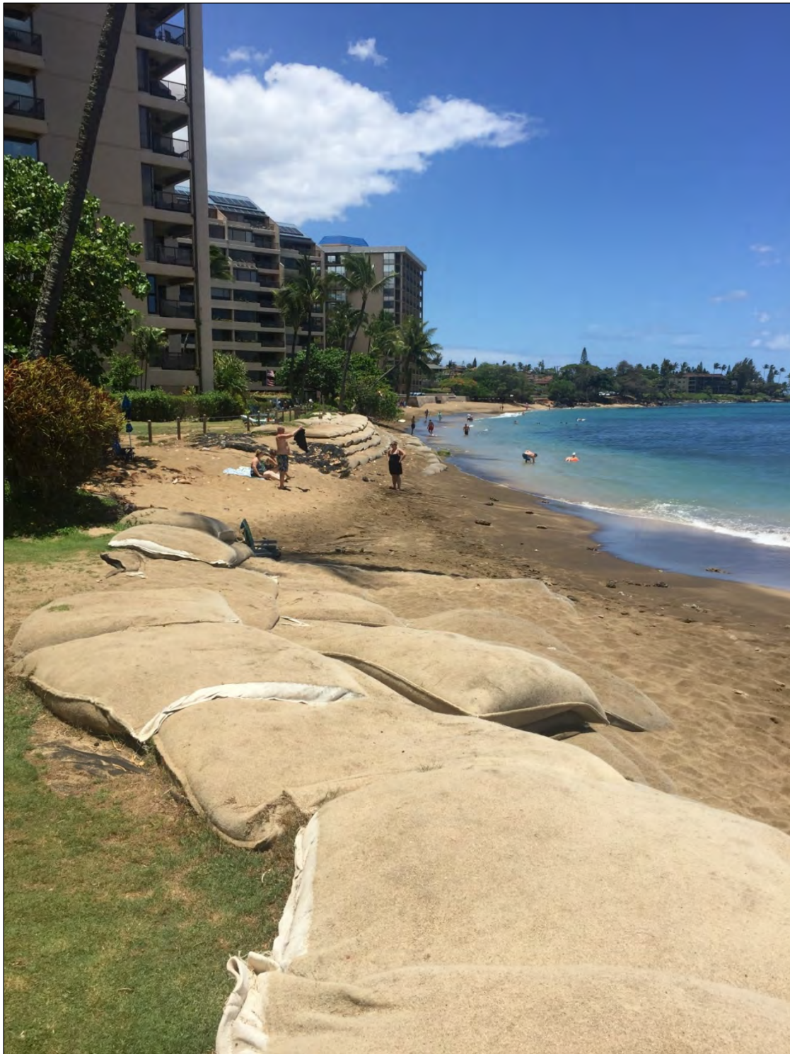
Figure 27. Looking west, sandbags stacked to prevent further coastal erosion (CSH 2019)
