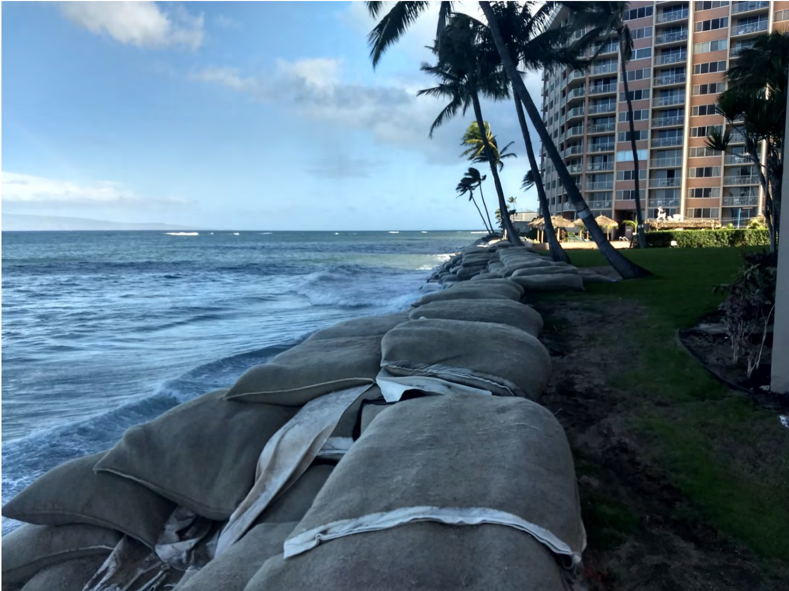
Figure 10: Photographic View of the Seaward Side of Part of the Royal Kahana and Sandbags Along the Shoreline. View to the North.
