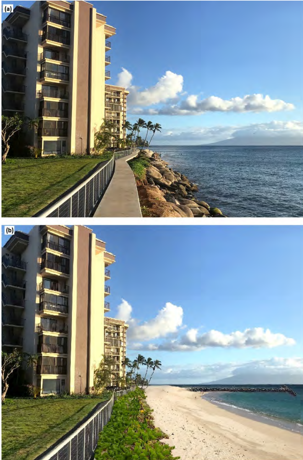
Figure 3-19: (a) Existing view looking south along the Hololani and Royal Kahana properties; (b) Artistic rendering with T-groin, widened beach, and vegetated berm
