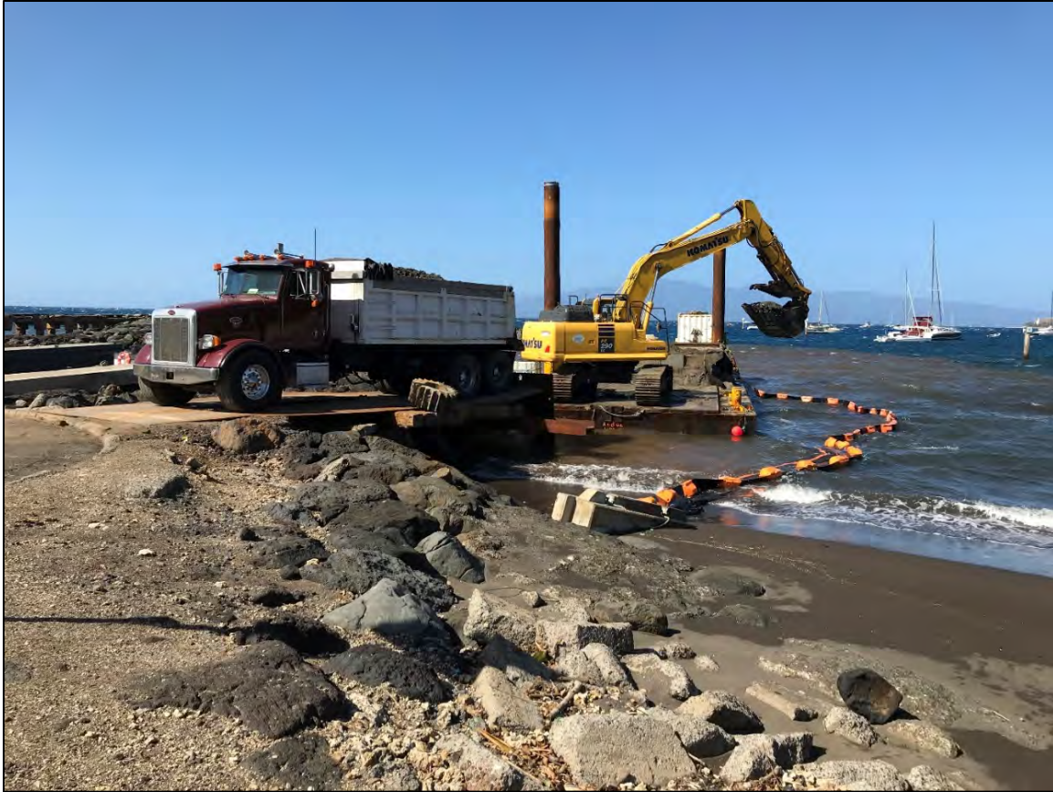
Figure 2-14: Mechanical Dredging using a Clamshell bucket at Mala Wharf on Maui
