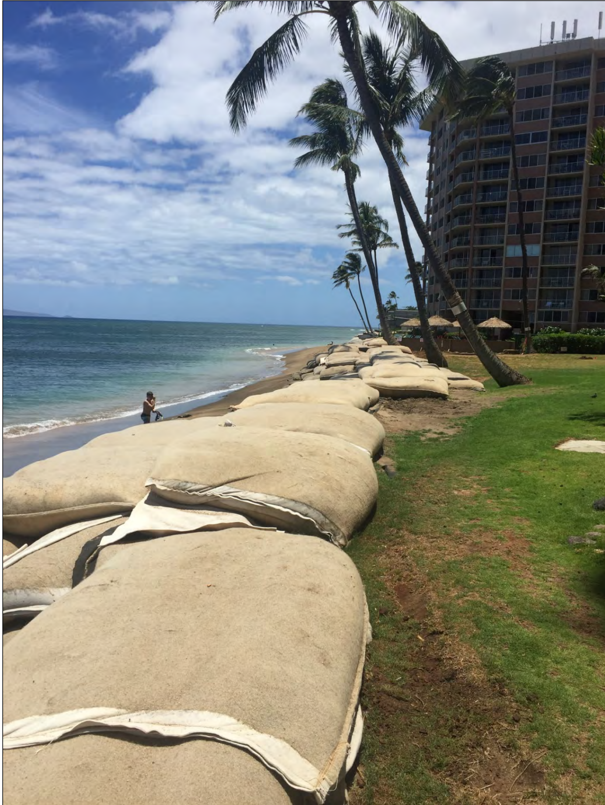
Figure 26. Sand bags are stacked and line the coast as a buffer of protection (CSH 2019)
