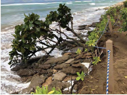
NOT JUST THE BEACH, BUT THE PROPERTY GROUNDS ARE BEING ERODED:
