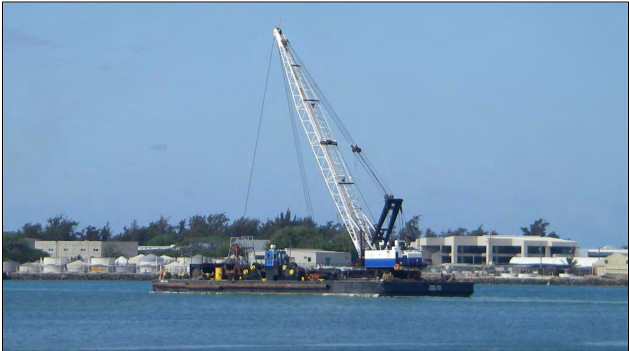
Figure 2-13: Crane Mounted to a Barge
