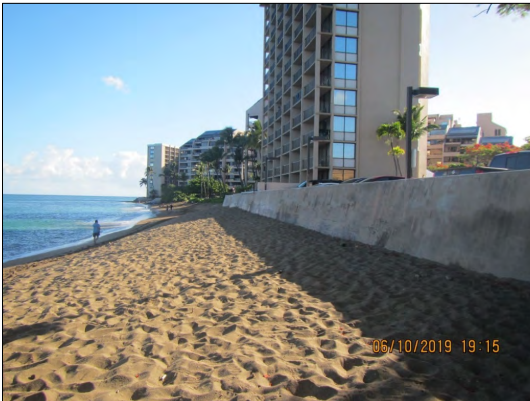
Figure 2-22: Seawall fronting the Kahana Beach Resort (June 2019)
