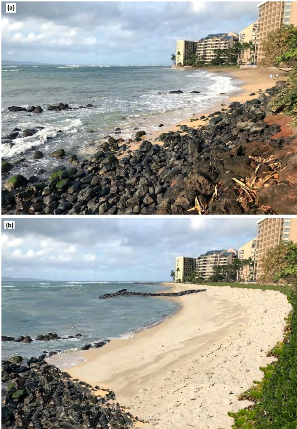
Figure 3-18: (a) Existing view looking north from the Pōhaku Beach Park toward the Kahana Beach Resort, Sands of Kahana, and Valley Isle Resorts; (b) Artistic rendering with T-groin, widened beach, and vegetated berm
