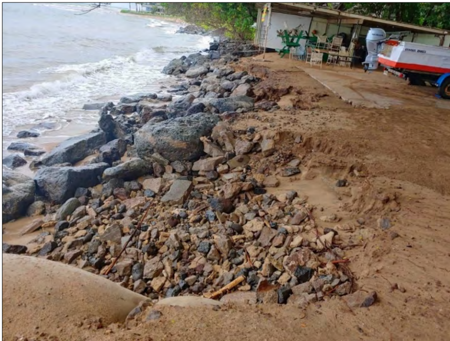
Figure 39. Looking east at the Sadang property. Cement foundation is gone, rocks are exposed, and sandy beach is gone (Courtesy of Mr. Felimon Sadang)
