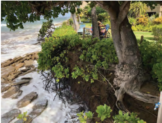
PROPERTIES ARE BEING FORCED TO CONTINUOUSLY RETREAT THEIR FENCED BOUNDARIES AS THE SWELLS REDUCE AND ERODE PROPERTY LINES EVERY DAY!
