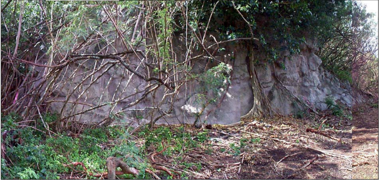
Figure 38: Photo-Gunnite Outer Wall of Revetment
