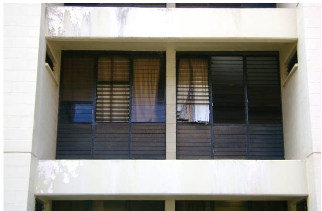
Photo 11. Damage sustained by Building 5070 as a result of improper installation of an air-conditioning unit.
