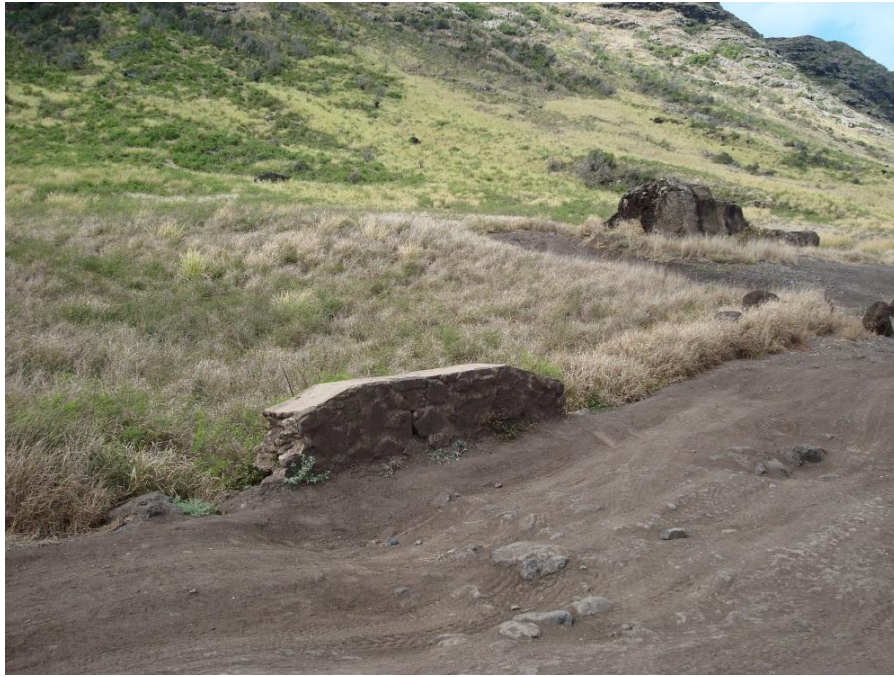
Fig. 1: Concrete-Capped Stonewall Barrier. These barrier walls were built at the edge of road where culverts pass under the road at natural drainages. Note the large boulder in the background is one of two considered by some to be culturally significant because they serves as off-shore triangulation points to locate fishing grounds.
