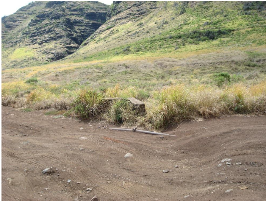
Fig. 2: Concrete-Capped Stonewall Barrier Next to Exposed Waterline. I have not counted the number of these walls, but all were constructed over drainages with culverts. I have not found any with a date but I assume that they were built when the road was in the 1950s. Proper names are etched in the concrete of some, but not a date. They are simple but are consistent in design.
