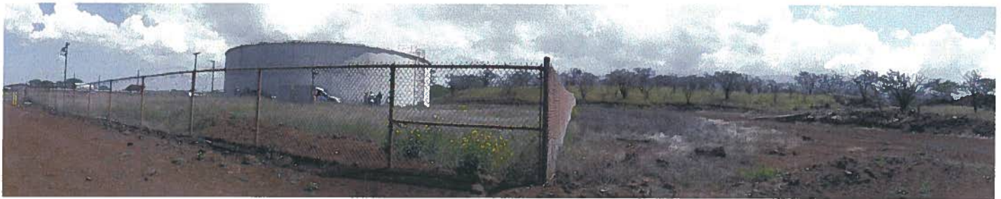
Photo 1: Existing 1.0 MG recycled water storage tank looking east/mauka.
