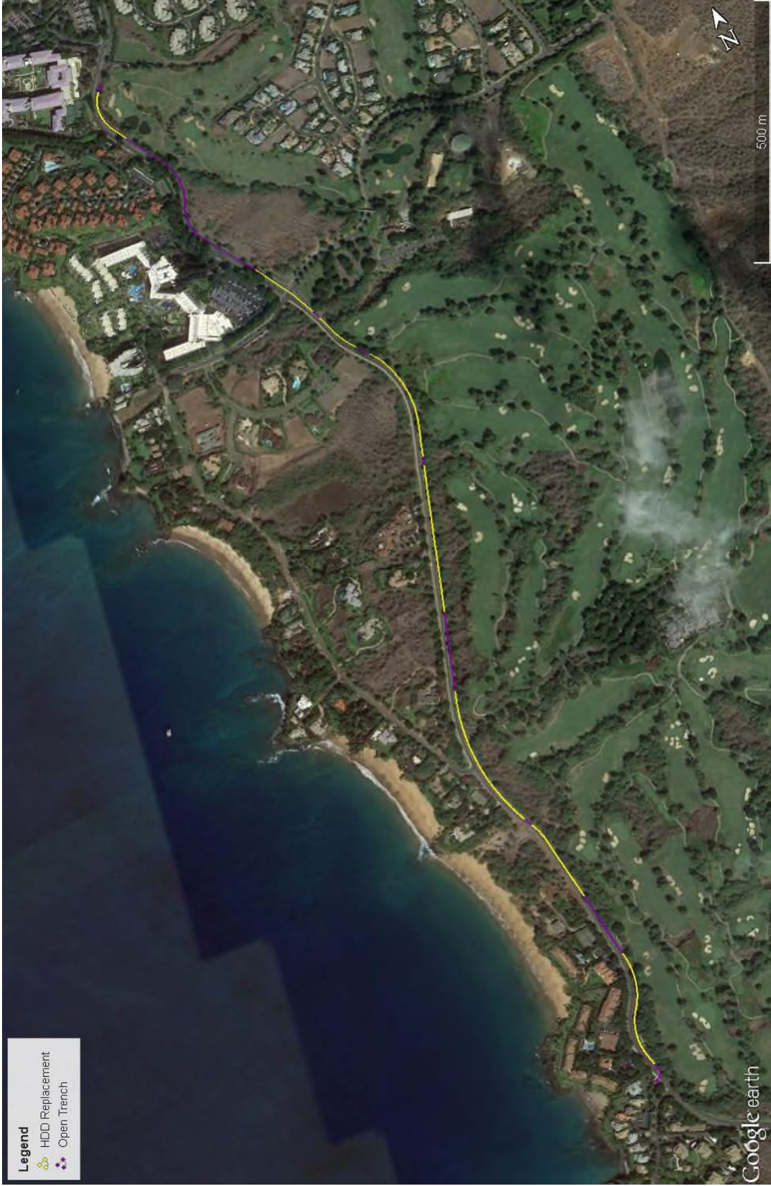
Attachment 2. Google earth map showing location of the proposed Kihei Wastewater Pump Station No. 16 Force Main (SFM) route.
