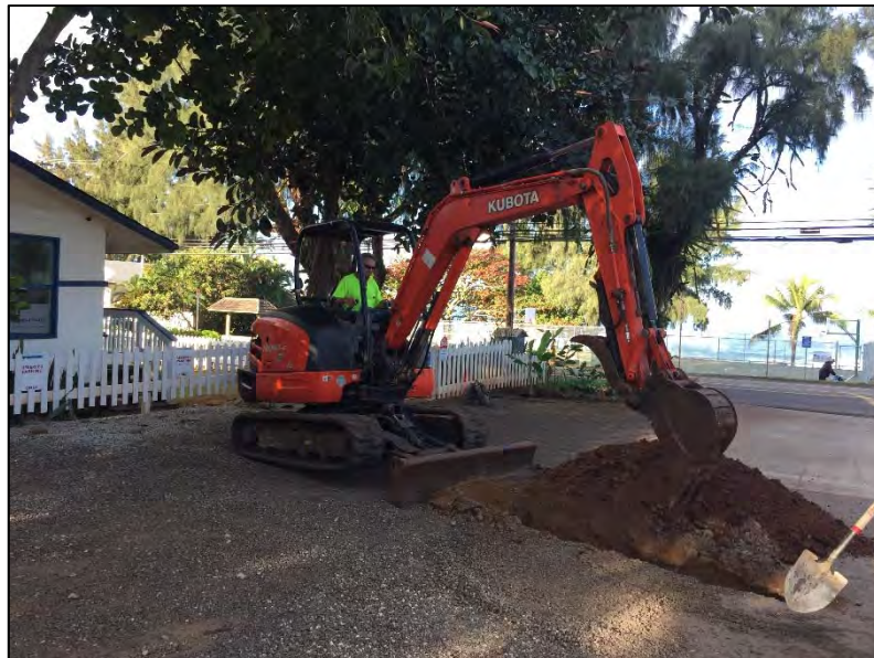
Figure 9. Excavation of TR 1 with mini excavator. Orientation is to the southwest.
