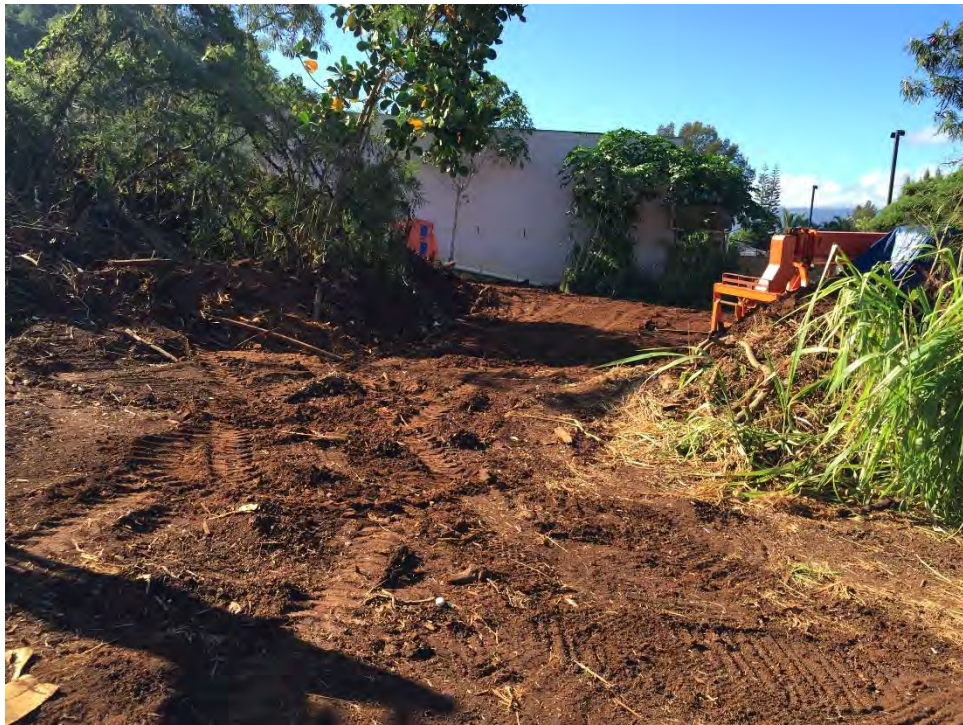
Figure 11. Bulldozed area. Orientation is to the south.
