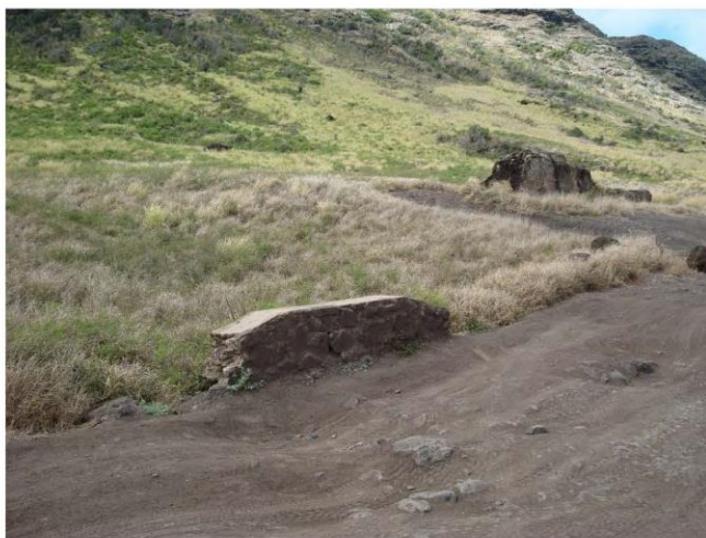
Fig. 1: Concrete-Capped Stonewall Barrier. These barrier walls were built at the edge of road where culverts pass under the road at natural drainages. Note the large boulder in the background is one of two considered by some to be culturally significant because they serves as off-shore triangulation points to locate fishing grounds.
