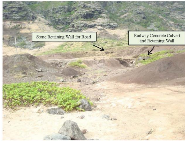
Fig. 3: Concrete Culvert and Retaining Wall for Railway and Stone Retaining Wall for 1954-1956 Roadway. The concrete culvert and retaining wall provided drainage through the leveled railway bed (foreground). The stone retaining wall was built along the steep edge of the 1954-1956 road bed.
