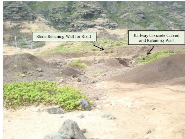
Fig. 3: Concrete Culvert and Retaining Wall for Railway and Stone Retaining Wall for 1954-1956 Roadway. The concrete culvert and retaining wall provided drainage through the leveled railway bed (foreground). The stone retaining wall was built along the steep edge of the 1954-1956 road bed.
