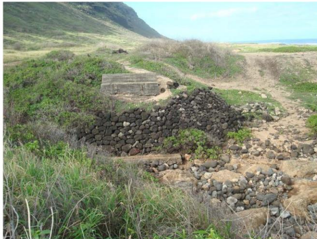
Fig. 6: Remnant of Railway Bridge Foundation and Stone Retaining Wall ( See Fig. 5). The characteristics of the leveled railway bed are still identifiable in many sections. The railway bed is raised in some sections and, in others, runs through cuts in higher ground. Low stone walls or alignments often run parallel to the railroad bed.
