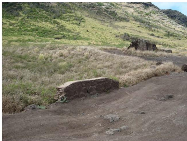
Fig. 1: Concrete-Capped Stonewall Barrier. These barrier walls were built at the edge of road where culverts pass under the road at natural drainages. Note the large boulder in the background is one of two considered by some to be culturally significant because they serve as off-shore triangulation points to locate fishing grounds.
