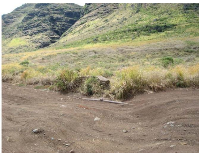
Fig. 2: Concrete-Capped Stonewall Barrier Next to Exposed Waterline. I have not counted the number of these walls, but all were constructed over drainages with culverts. I have not found any with a date but I assume that they were built when the road was in the 1950s. Proper names are etched in the concrete of some, but not a date. They are simple but are consistent in design.
