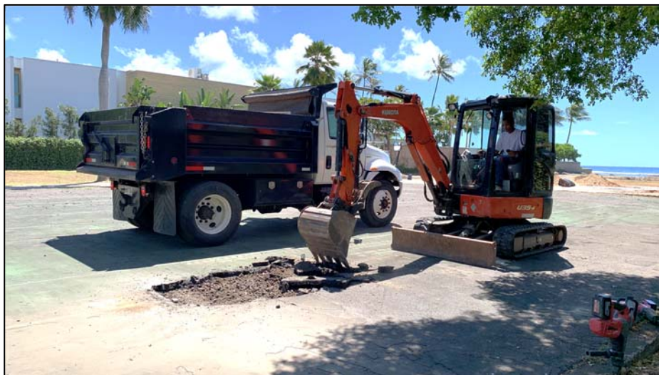
Figure 14. Heavy equipment used during the AIS. View is to the southeast.
