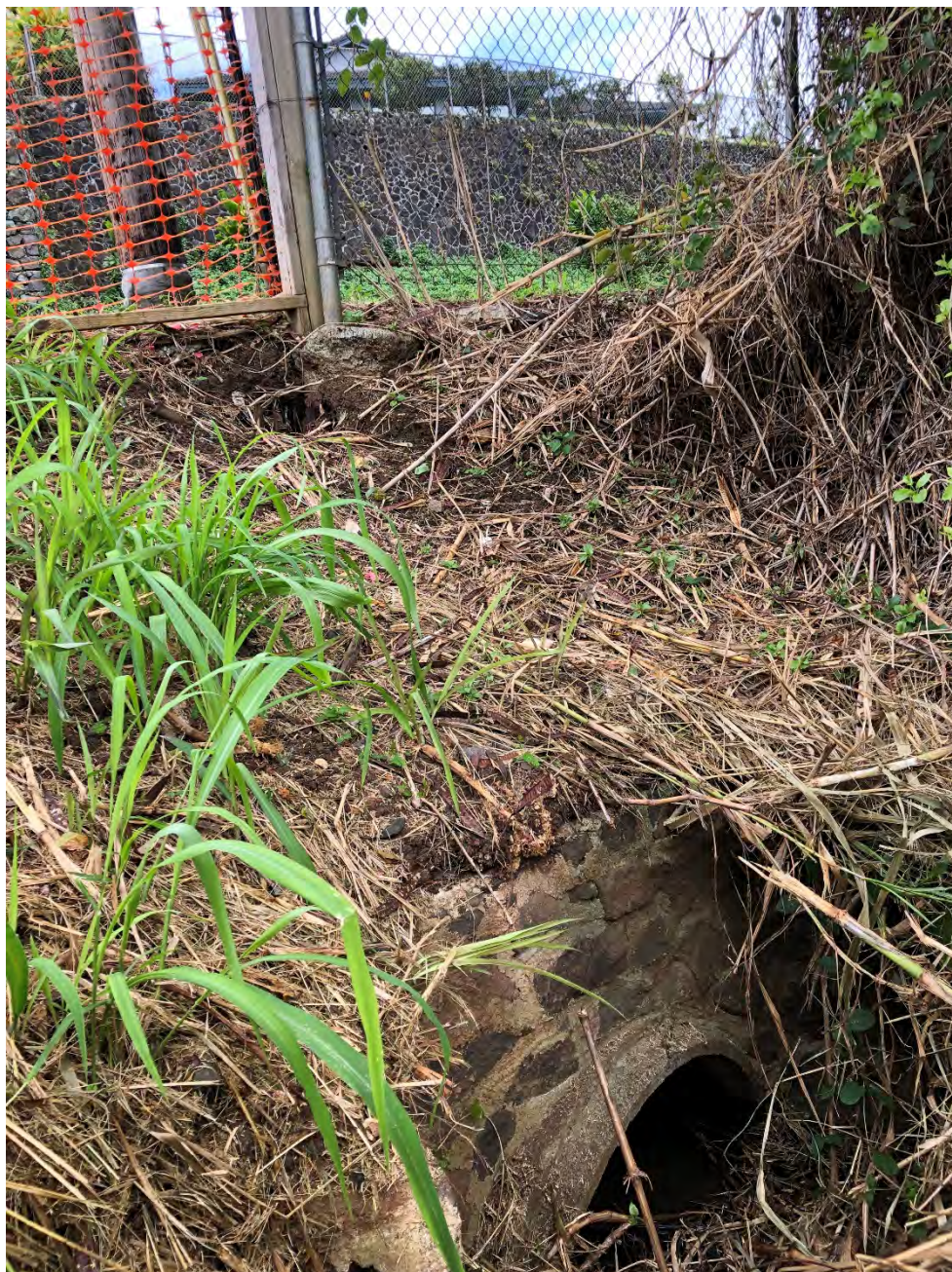
Photo 2. Concrete culvert just below Lamaula Road at the head of the unnamed ditch that runs along the northern boundary of the project site.
