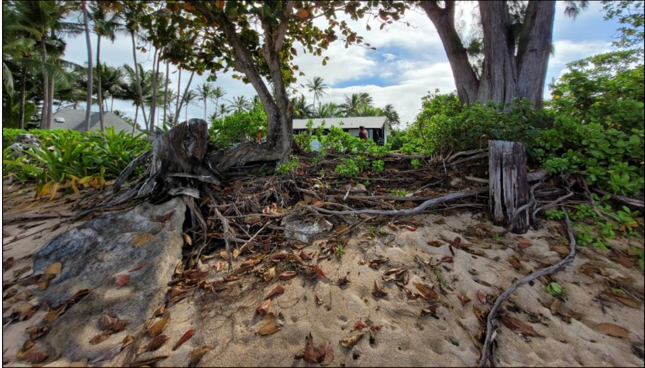
Figure 3.11: Minor Evidence of Shoreline Erosion
