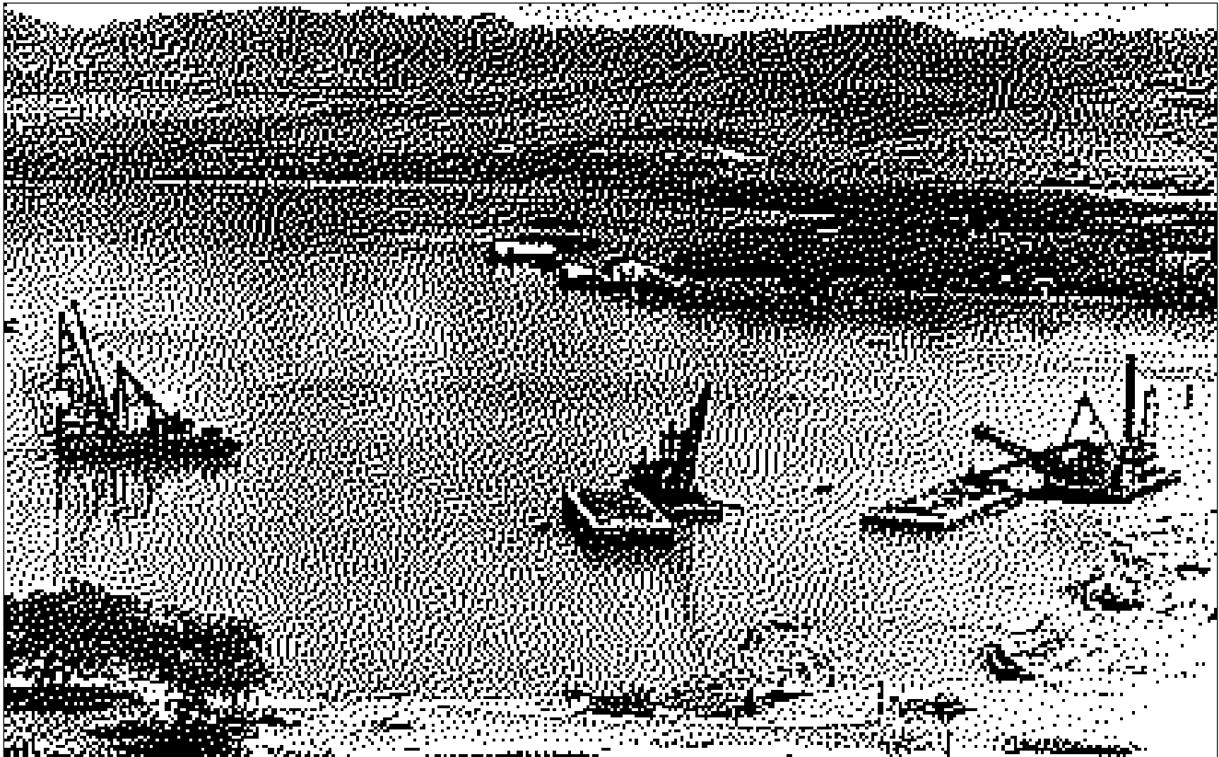
Figure 14. Dredging in Pearl Harbor ca. 1908 (Hawai'i State Archives)
