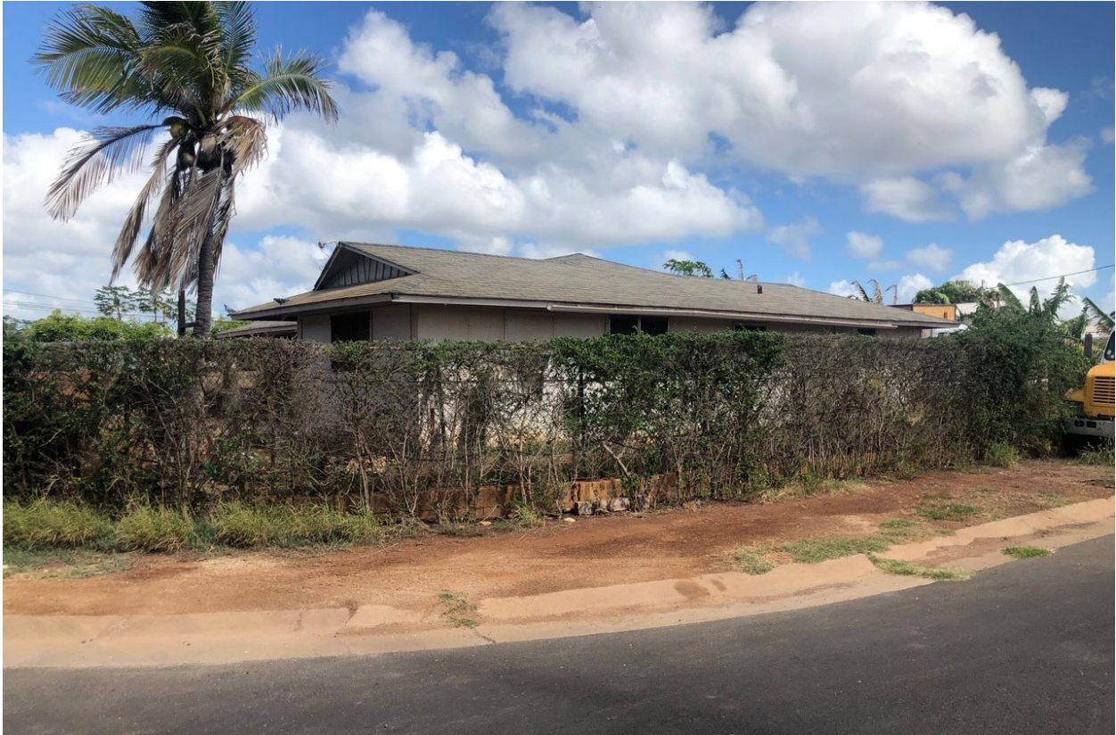
Photograph C – Existing single family dwelling at Pupu St.
