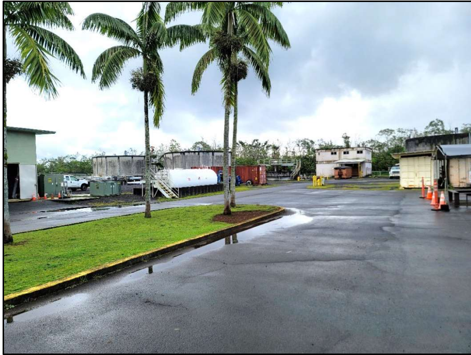
Figure 16. Photo overlooking the Hilo WWTP from the parking lot at the fenced plant entrance; view to east
