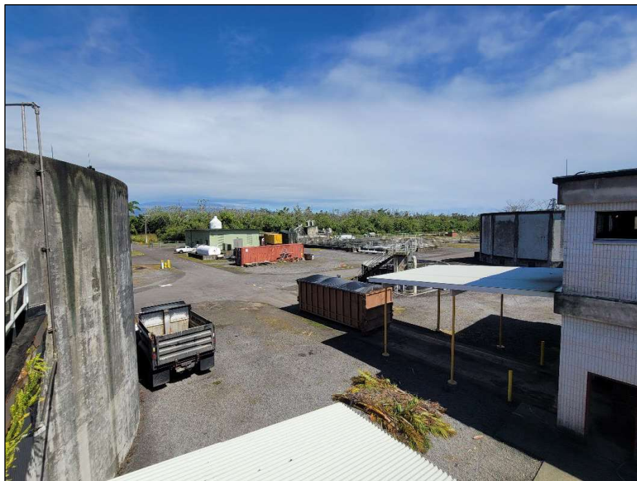
Figure 17. Photo overlooking the Hilo WWTP from the existing digester control building; view to northwest
