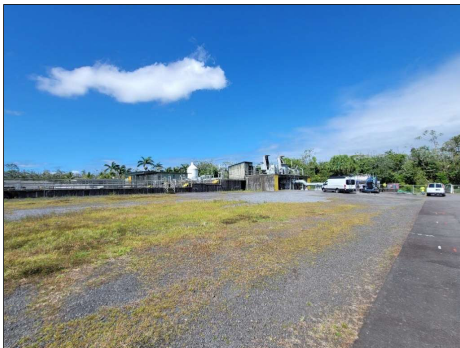
Figure 23. Photo overlooking the central-western portion of the Hilo WWTP, where several Phase 1 improvements are planned; view to southwest
