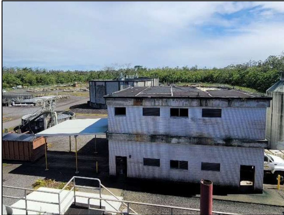
Figure 22. Photo overlooking the central-eastern portion of the Hilo WWTP, where several Phase 1, Phase 2, and Future improvements are planned; view to north
