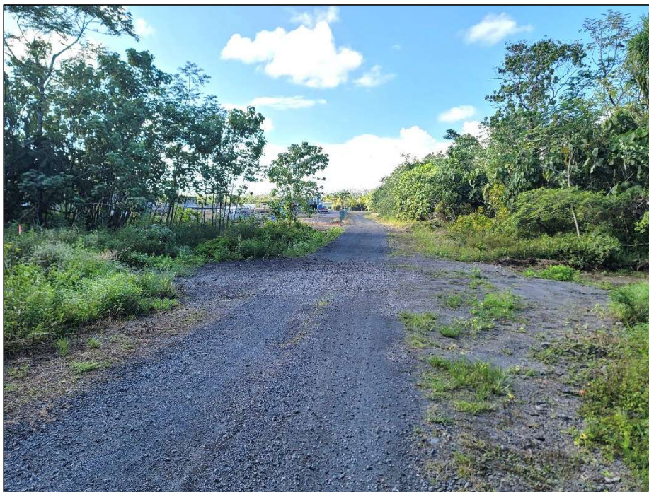
Figure 33. Photo overlooking the gravel roadway and adjacent graded areas located along the northwestern boundary of the plant property; view to south
