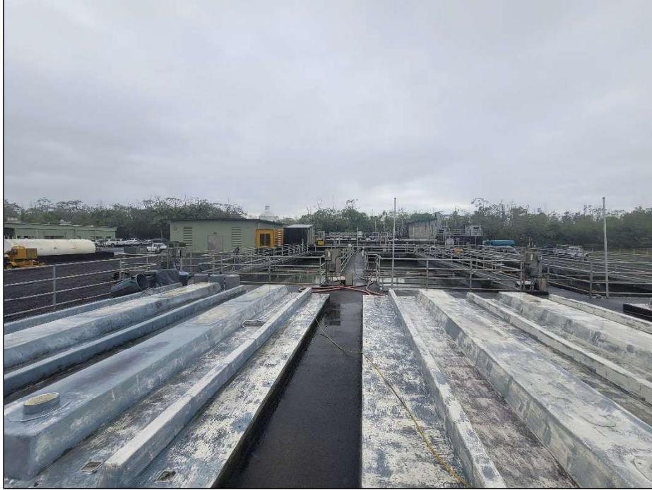
Figure 24. Photo overlooking existing sedimentation tanks in the central-western portion of the Hilo WWTP, where Phase 1 improvements are planned; view to west
