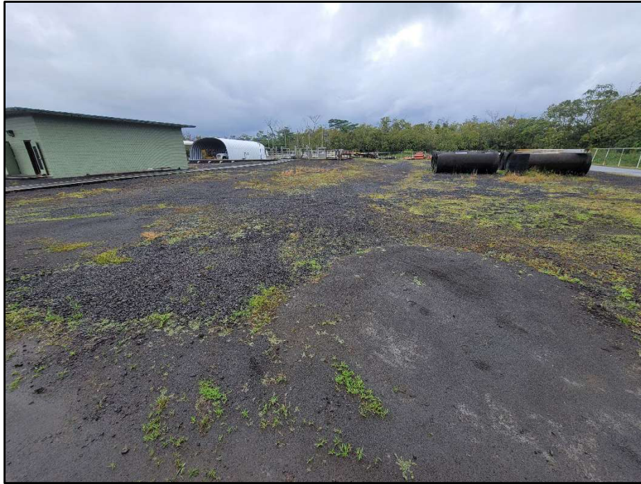
Figure 18. Photo overlooking the northeastern portion of the Hilo WWTP, where Phase 2 improvements are planned; view to north
