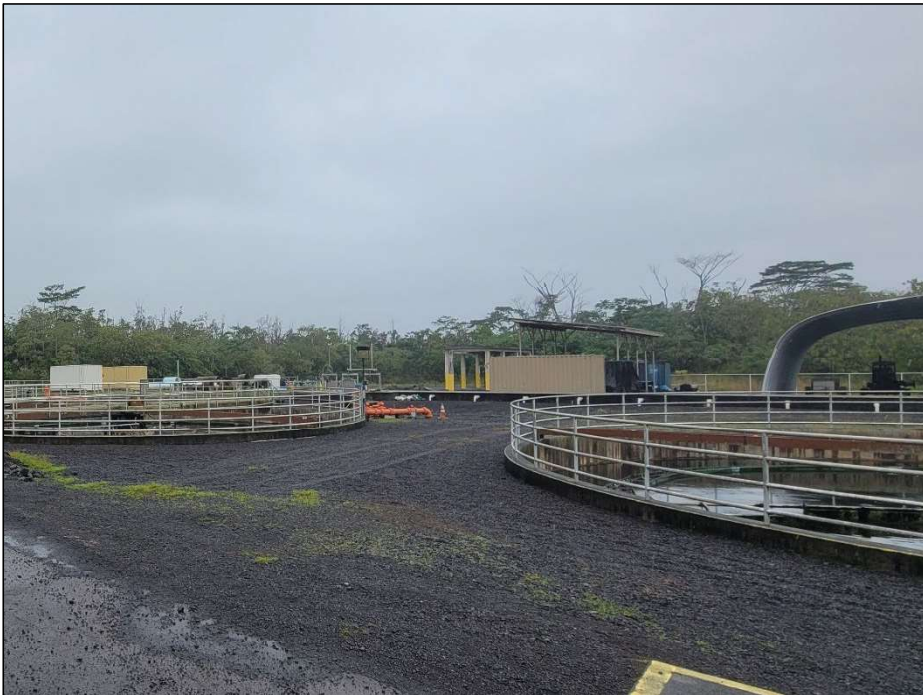
Figure 21. Photo overlooking the northwestern corner of the Hilo WWTP, where a Phase 2 improvement is planned at the tan-colored structure visible at center of photo; view to northwest
