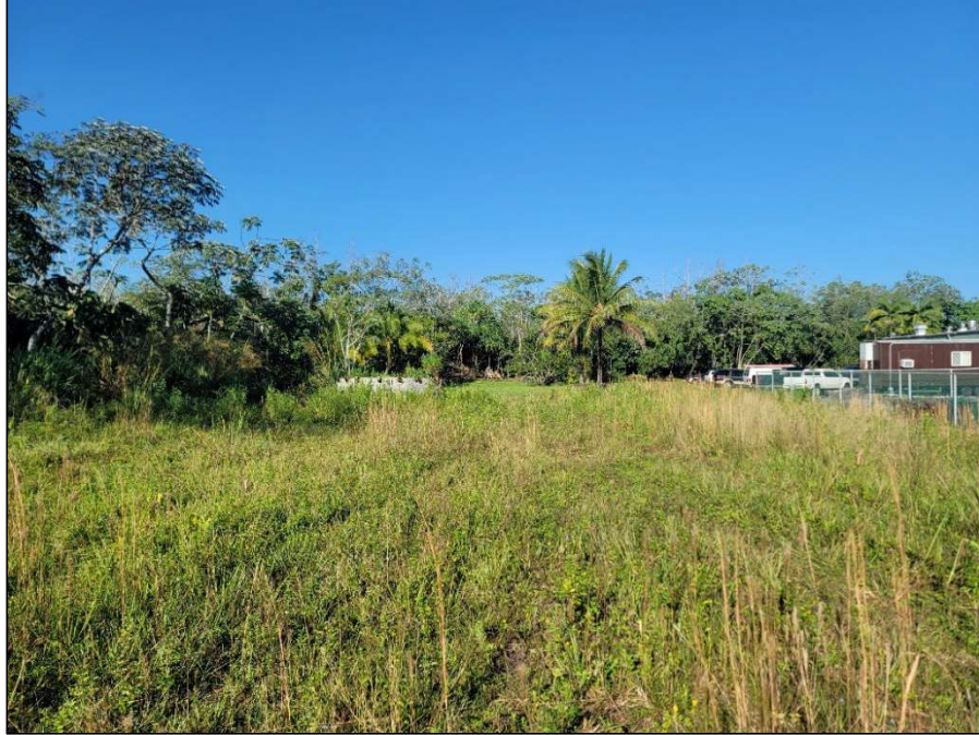
Figure 30. Photo overlooking the open, graded perimeter area immediately south of the plant security fence, where a Phase 1 flare and Future cogeneration facility are planned; view to west
