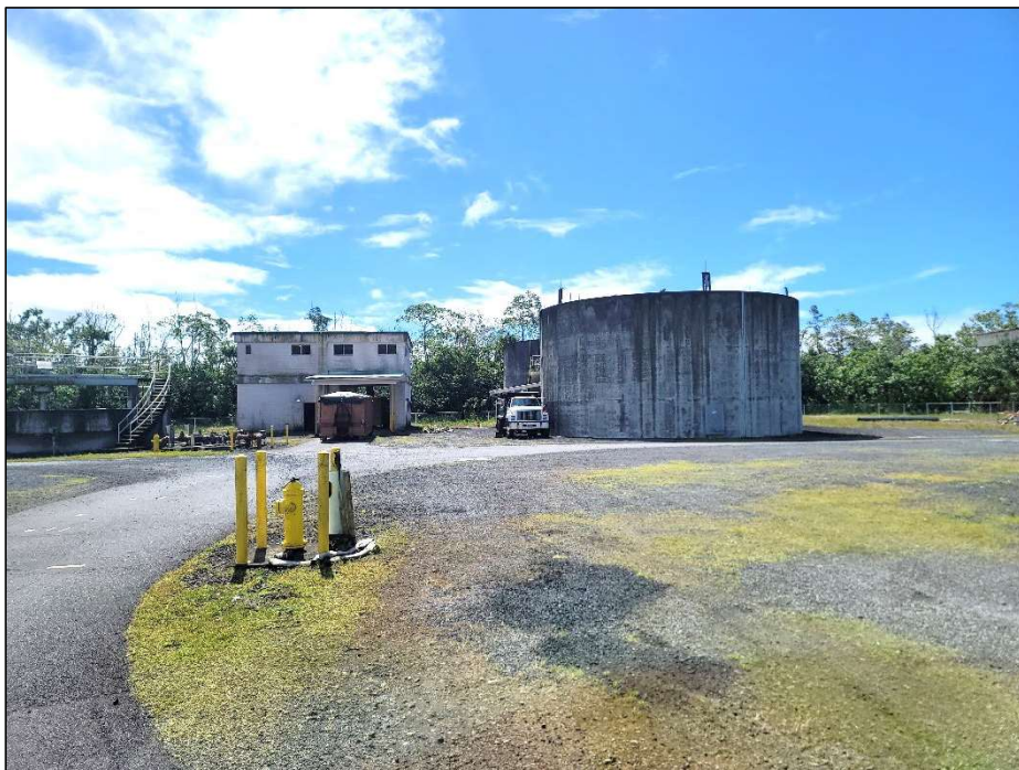
Figure 27. Photo overlooking the southwestern portion of the Hilo WWTP, where several Phase 1, Phase 2, and Future improvements are planned; view to east
