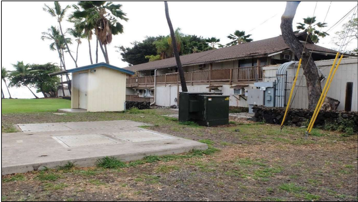
Photo 1. Sewer pump station located on the makai side of the intersection at Alii Drive and Hualalai Road.
