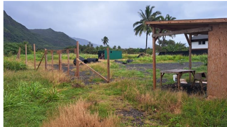
Photo 18: Unit 7 fencing & temporary shelter have been reportedly removed or properly permitted
