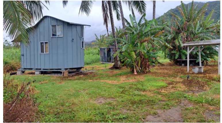
Photo 22: Tiny structure (guard shack) guard shack, located at the NW corner of unit 10 and within the wetland area, will be relocated outside the wetland near the driveway and properly permitted.
