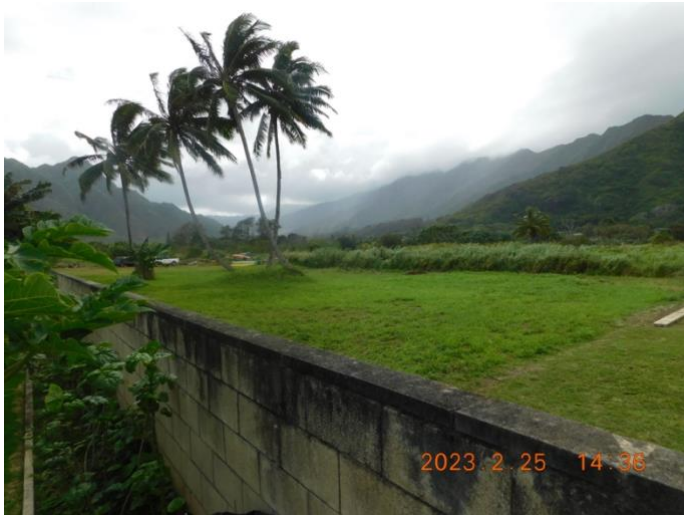
Photo 13: View of Unit 11 Lot from Unit 5 west CMU wall, facing southwest.
