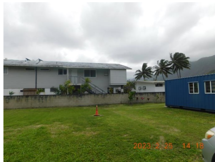
Photo 4: Unit 4 facing south, with Unit 5 Container to the right (to be permitted)
