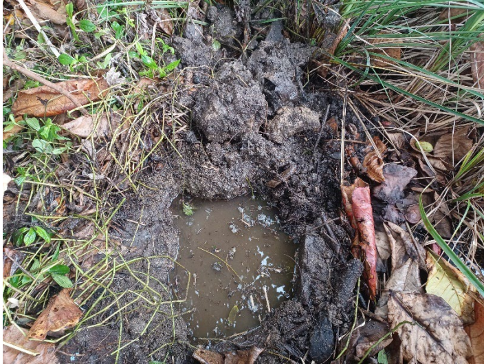
SP-02 is 16 in away from standing water. Water table is 4 in deep. Chunks of asphalt that were removed at SP-02 can be seen above it.
