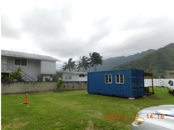
Photo 5: Unit 5, facing southwest. Dwelling to be Constructed, container to be permitted as storage.
