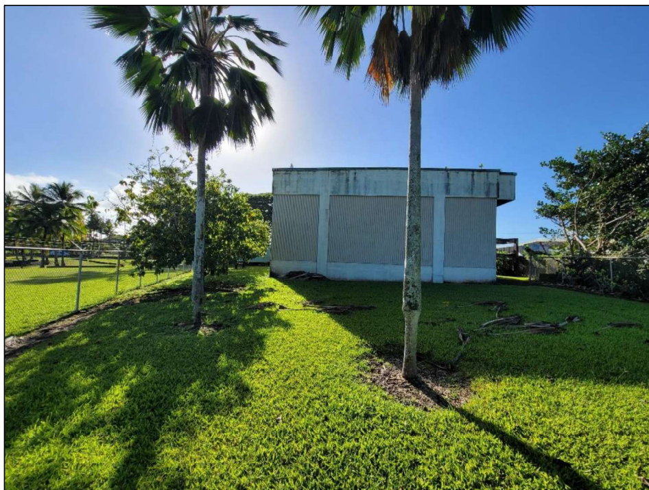
Figure 38. Photo overlooking the rear of the pump station and operations building at the Pua SPS facility; view to southeast
