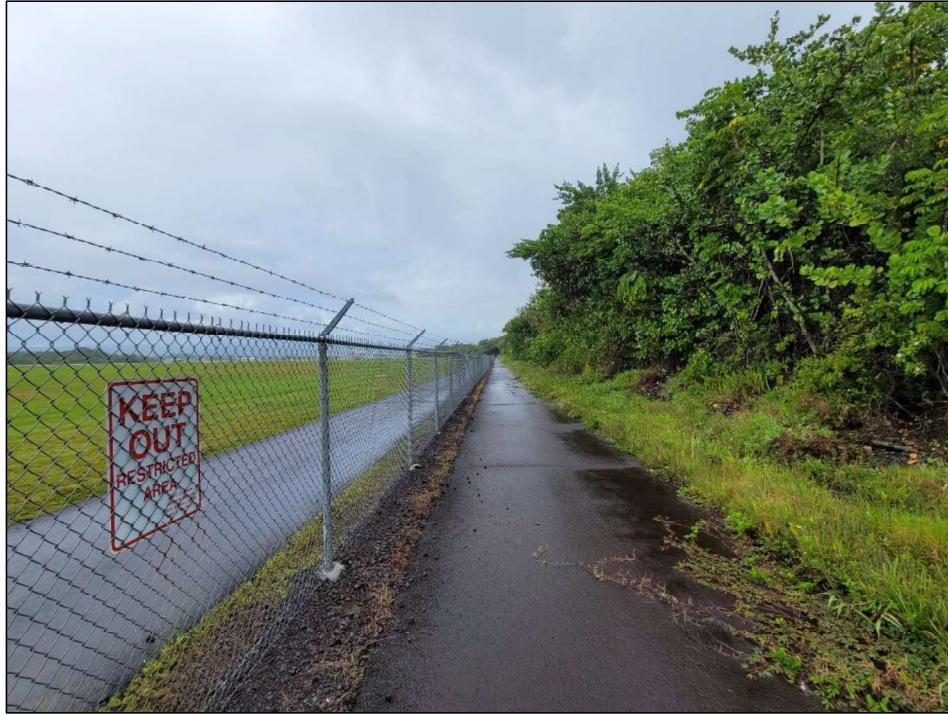
Figure 20. Photo overlooking the existing force main corridor along the northern side of the airport runway; view to west
