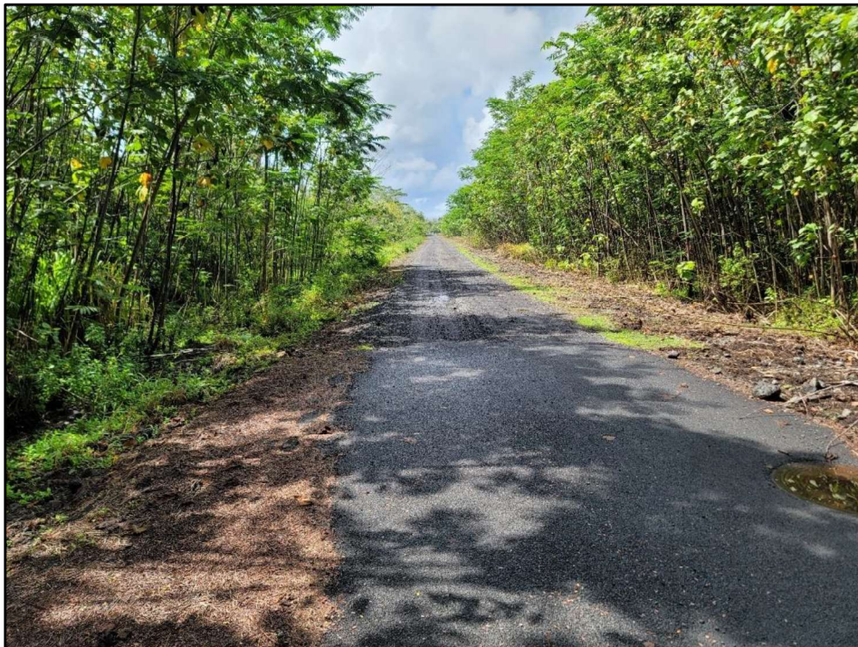
Figure 21. Photo overlooking a portion of the existing force main corridor within the project area; view to south
