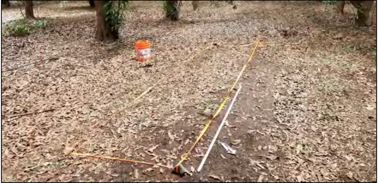
Figure 59. Photo of TE 6 marked out with flagging tape prior to excavation; view to southwest
