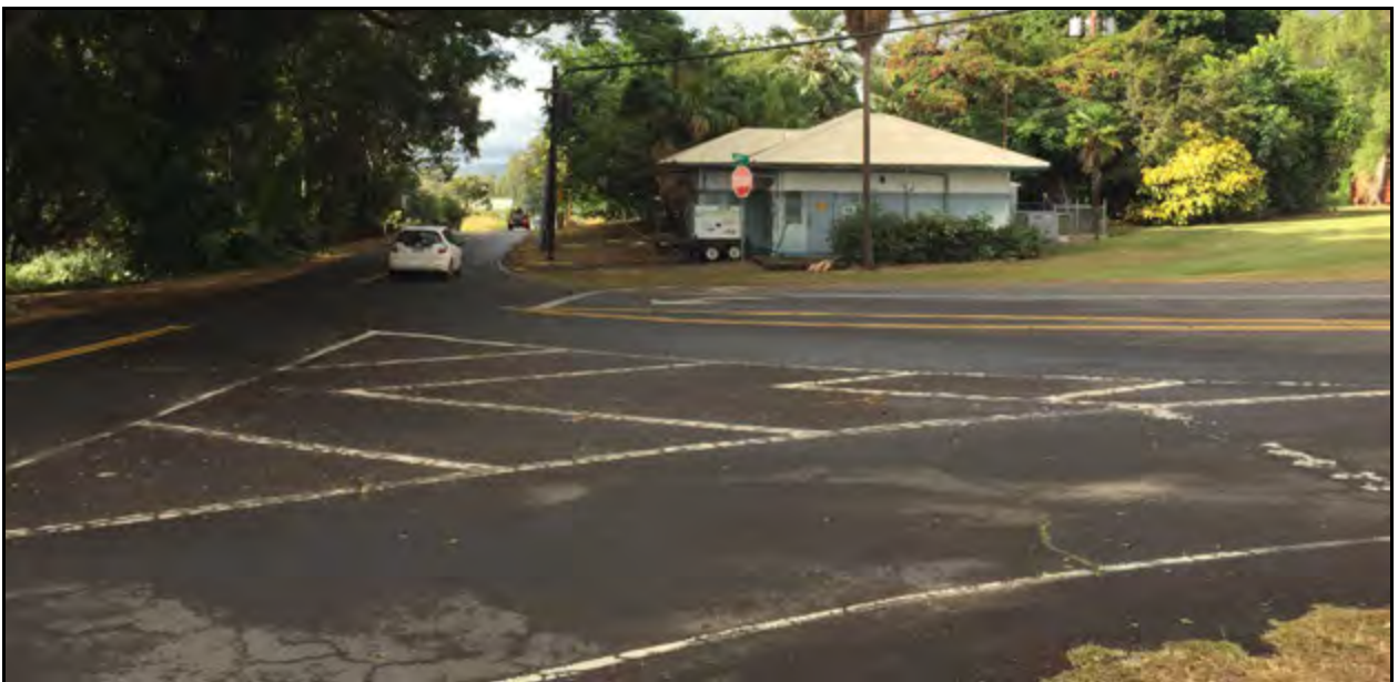
Figure 33. Photo showing the Pikake Street terminus at Maile Street; Hawaiian Telcom building is on opposite corner; view to southwest
