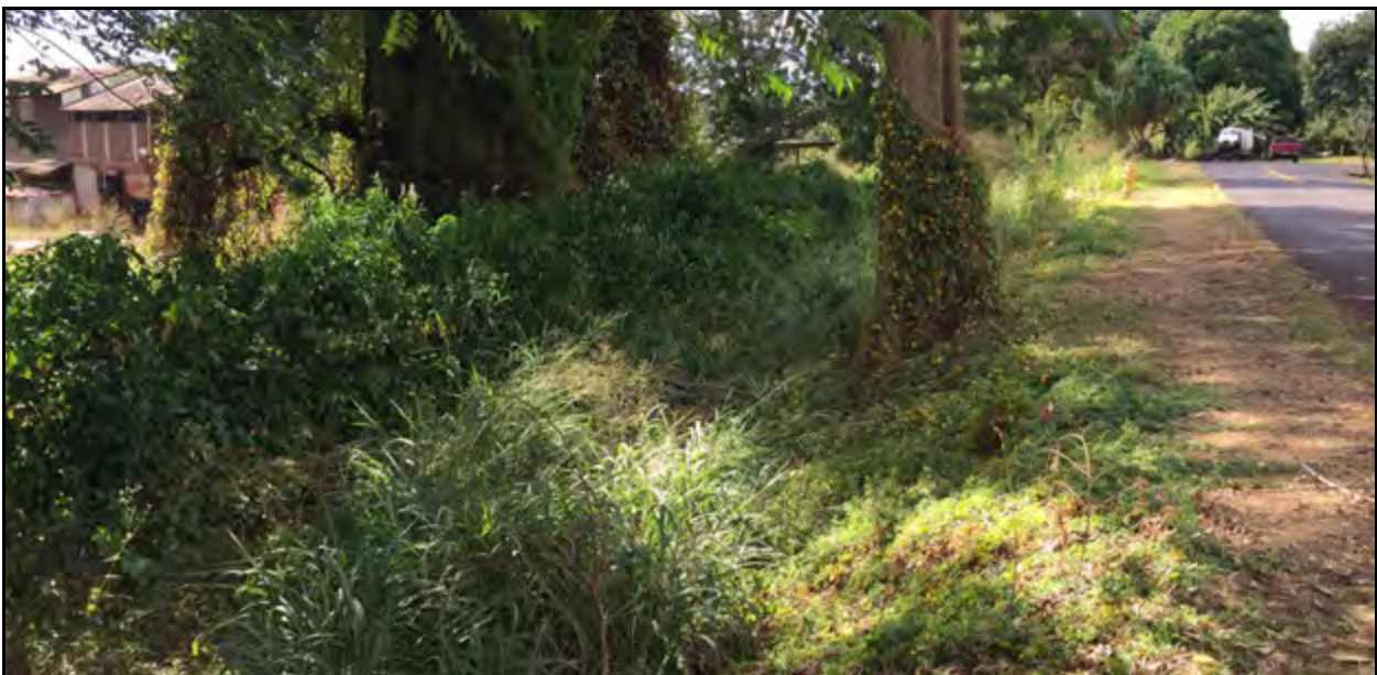
Figure 25. Photo showing the location where the easement in TMK: [3] 9-6-005:036 exits at Ilima Street (frame right); the earthen drainage channel extending from the Huapala Street culvert is beneath the grass to the left of the road; view to southwest
