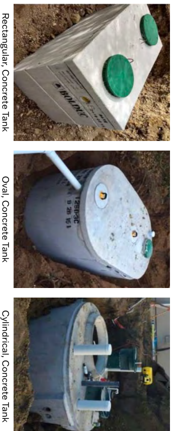
Figure 3.2: Common septic tank materials and shapes in Hawaii 1 (Carollo, 2021).
