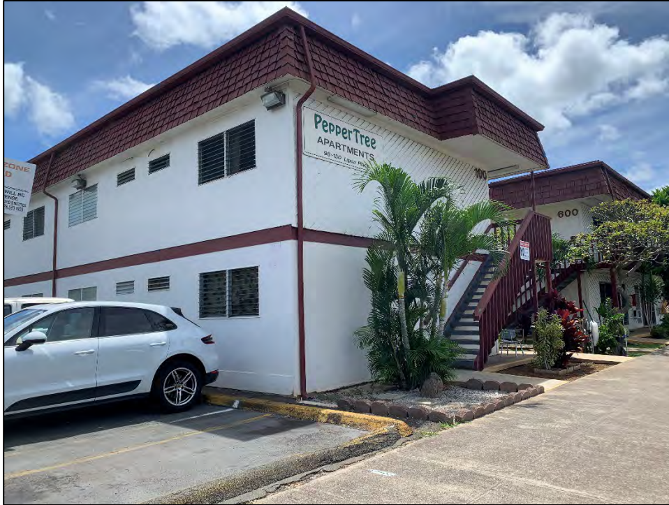
Figure 16. Corner view of PepperTree Apartments, facing east-northeast.
