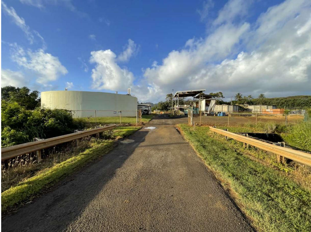
Figure 1: Street View of Access Road to Lihue WWTP
