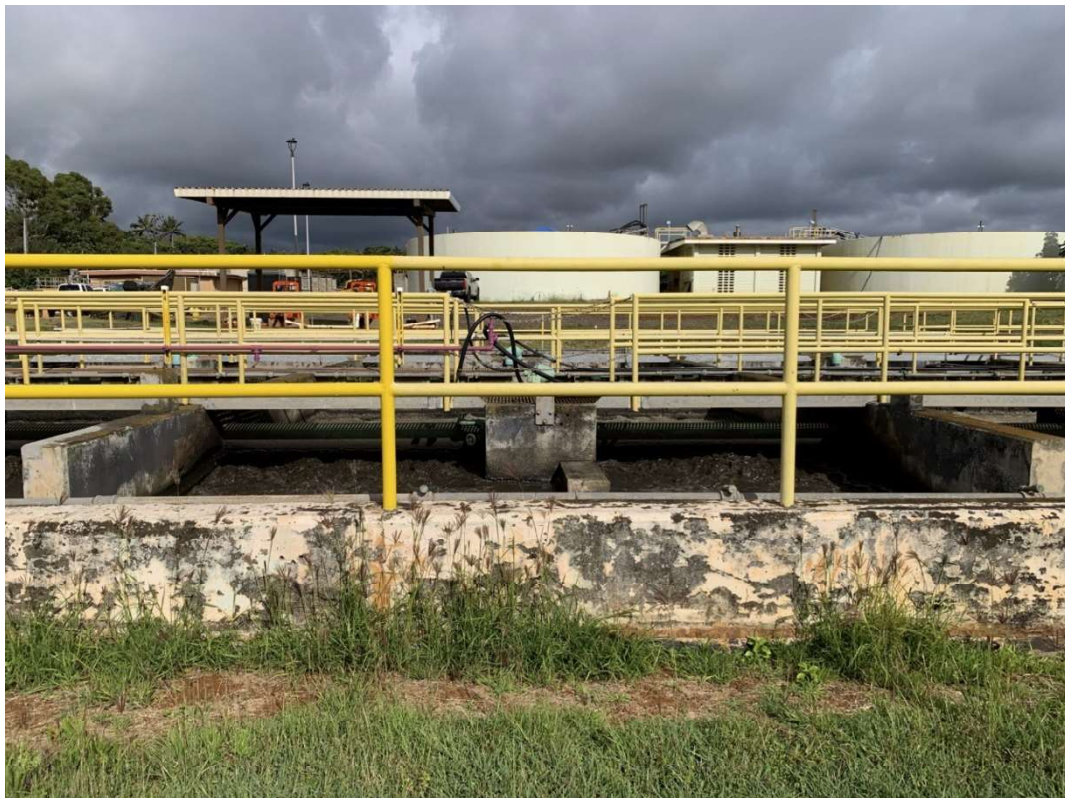
Figure 6: View of the Project Area from the East
