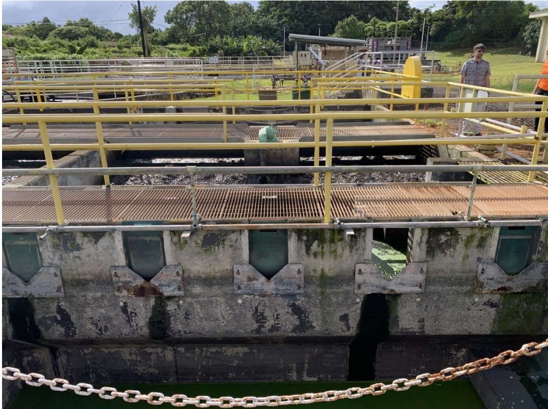
Figure 5: View of the Project Area from the West
