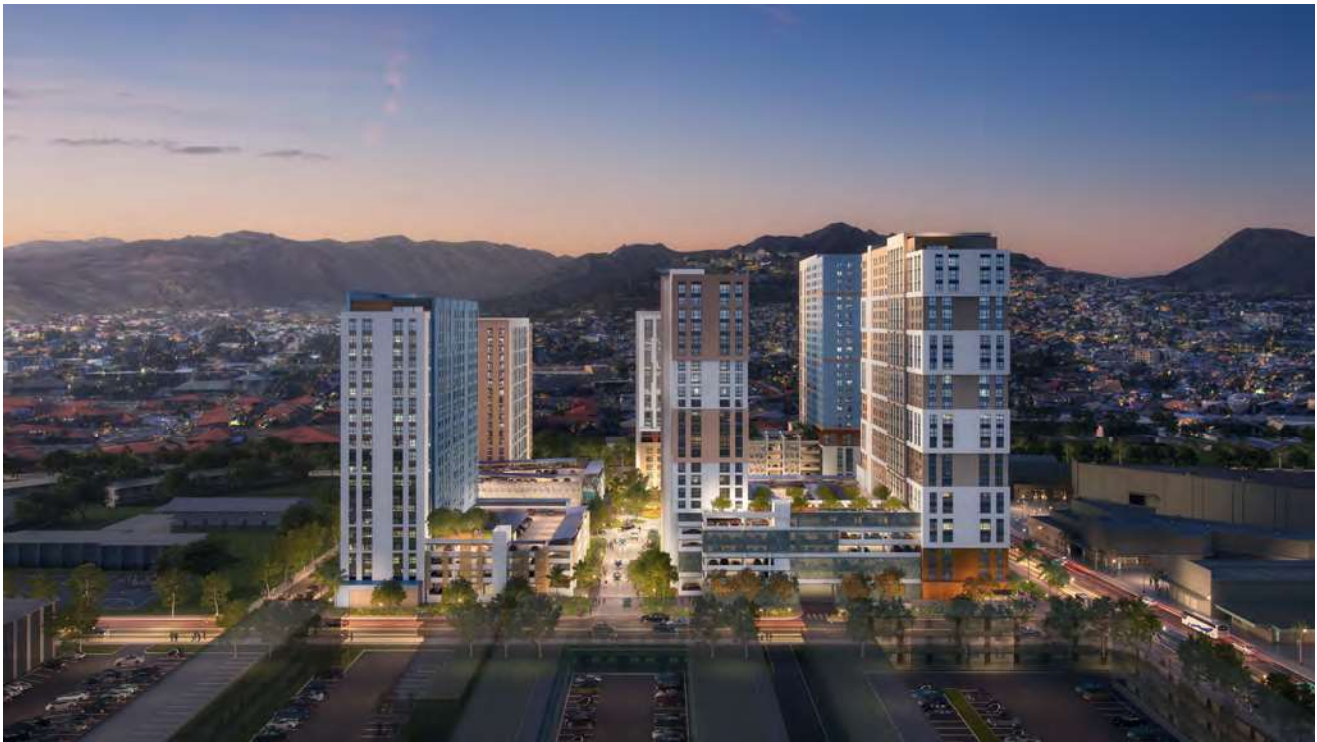
Mauka view from Skyline guideway.
