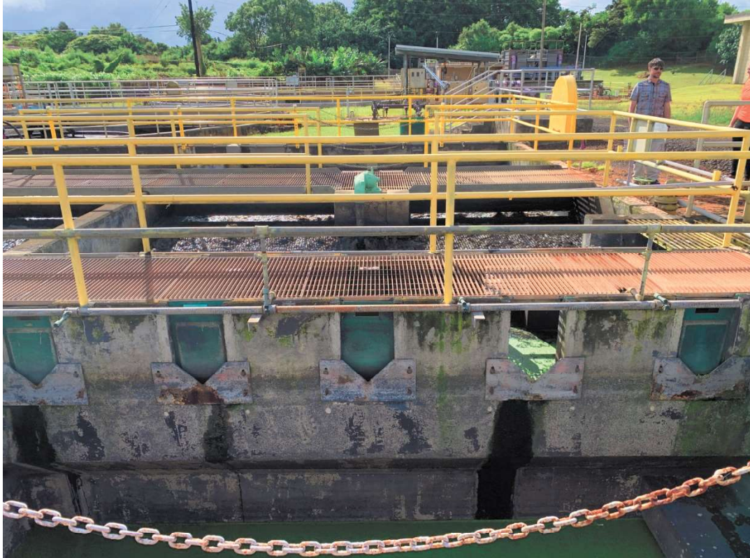
Figure 5: View of the Aerated Solids Contact Tank from the West
