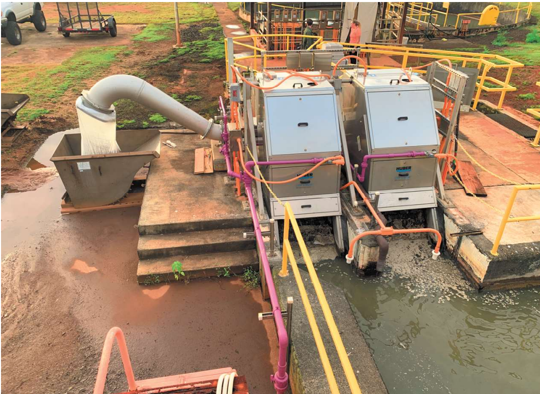
Figure 10: View of the Headworks from the West
