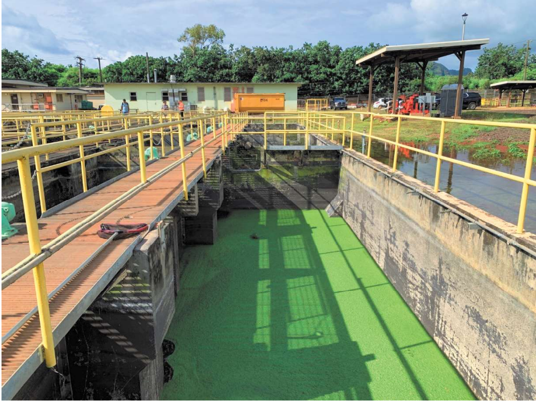
Figure 7: View of the Aerated Solids Contact Tank from the North
