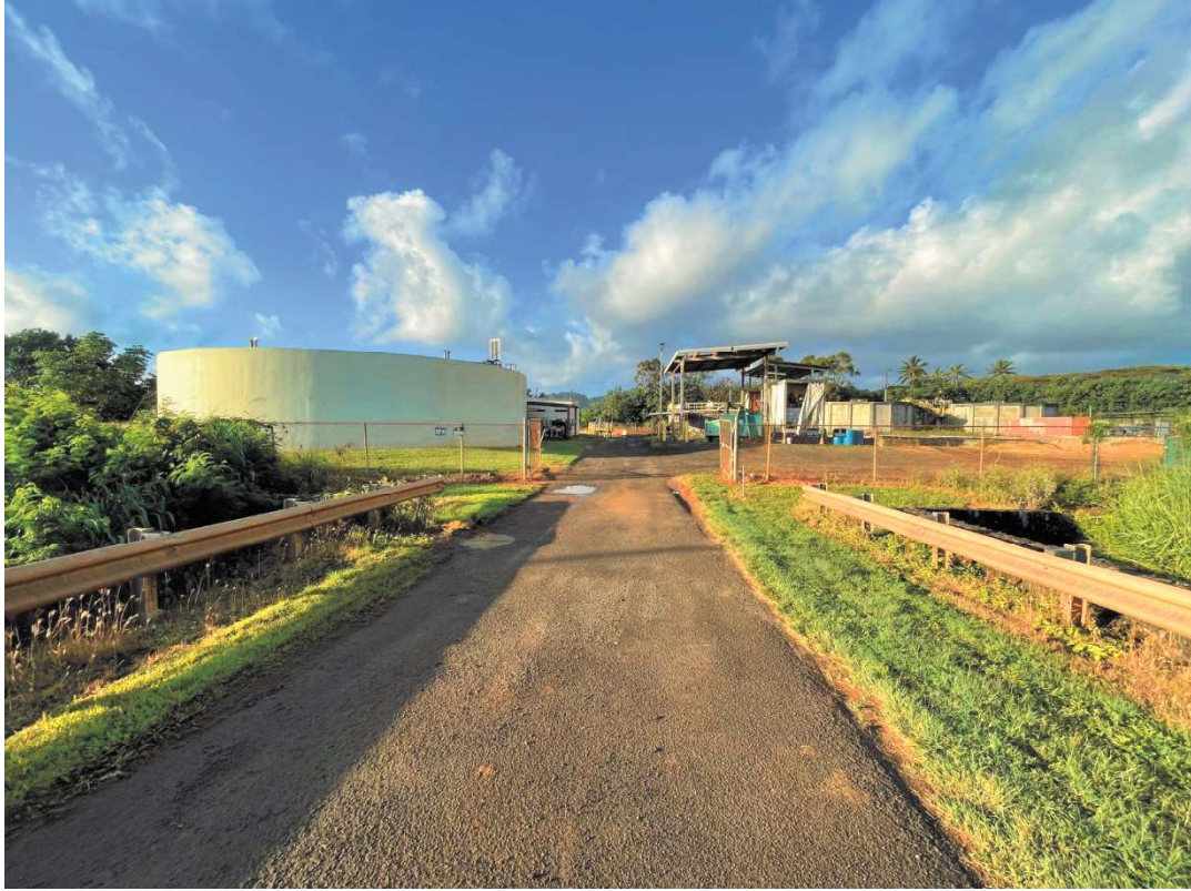
Figure 1: Street View of Access Road to Lihue WWT
