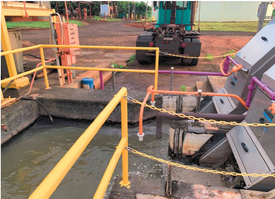
Figure 8: View of the Headworks Tank from the South
