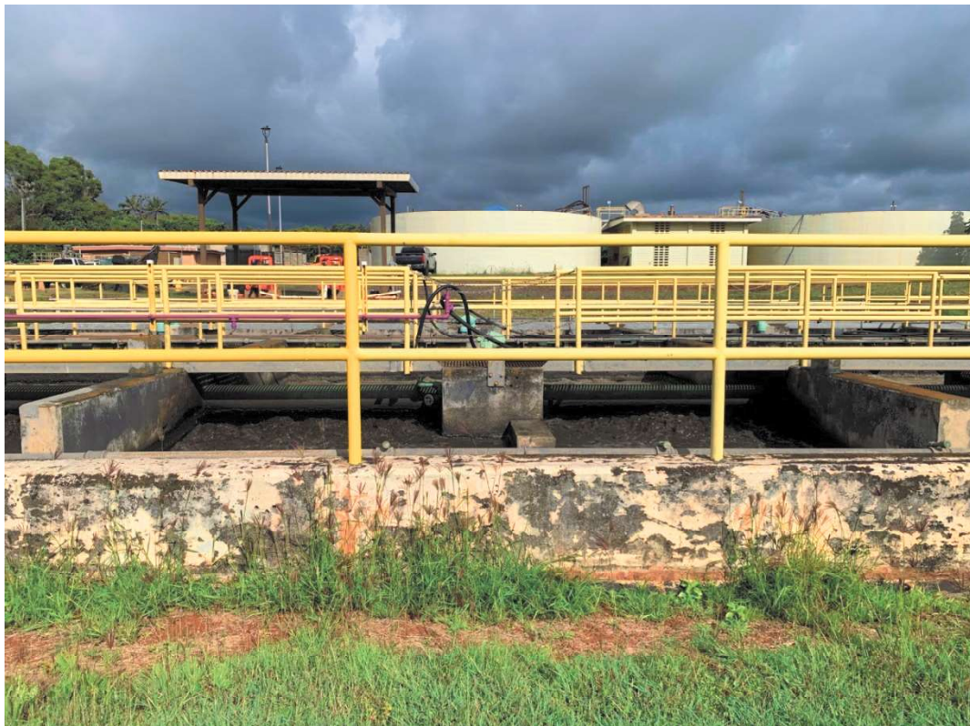
Figure 6: View of the Aerated Solids Contact Tank from the East
