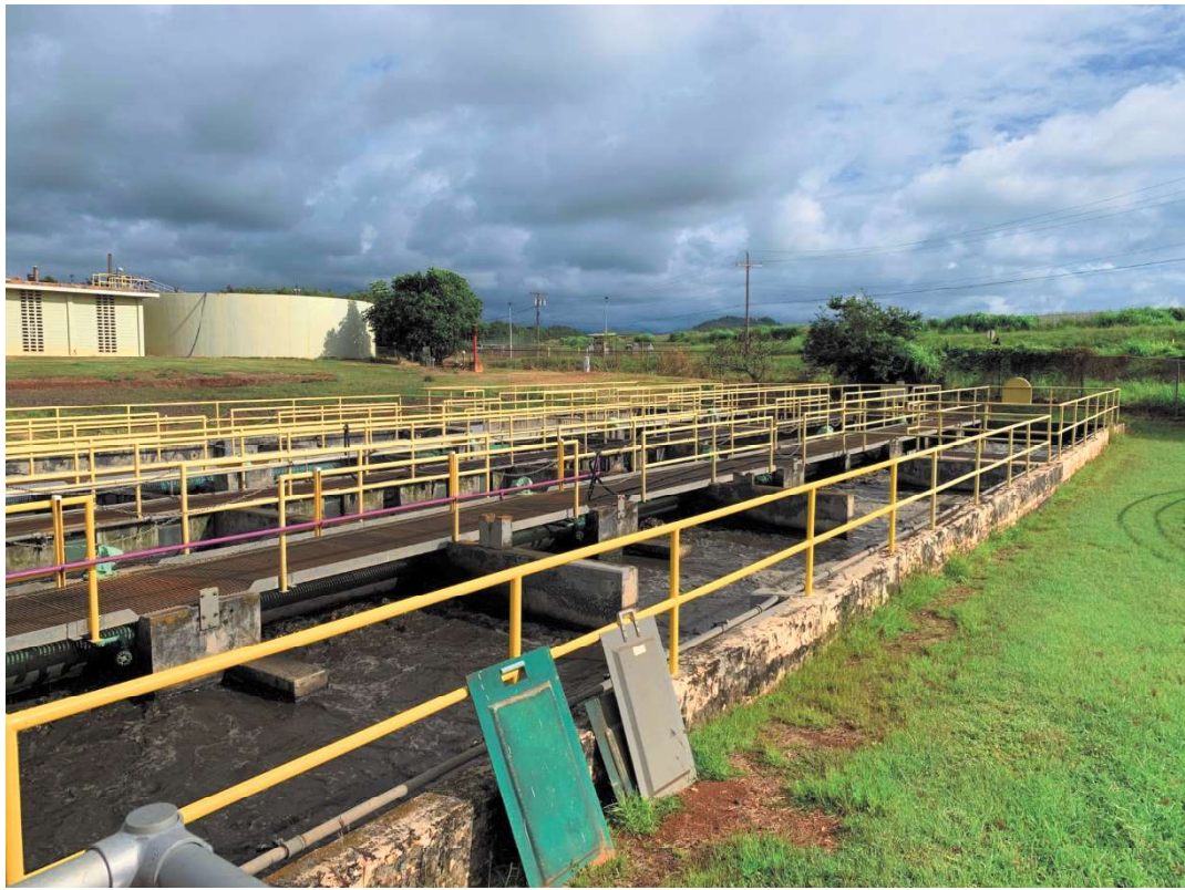
Figure 4: View of the Aerated Solids Contact Tank from the Southeast
