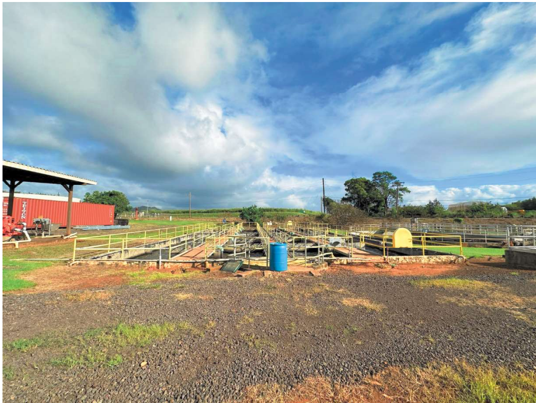
Figure 2: View of the Aerated Solids Contact Tank from the South
