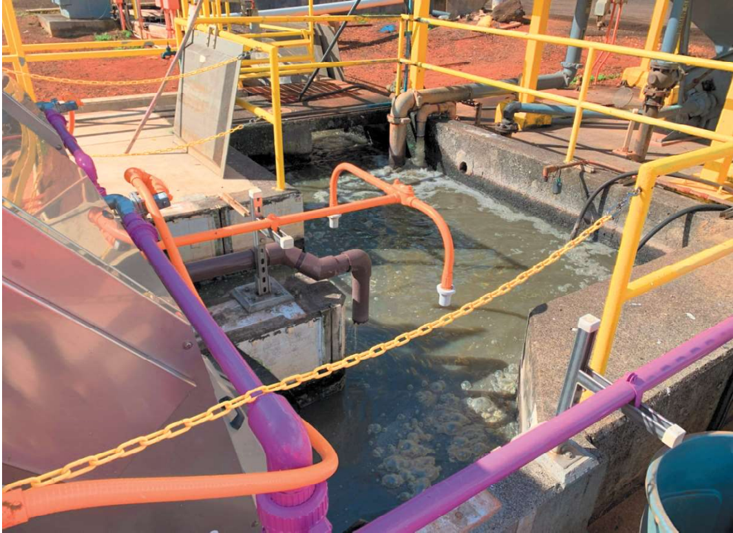
Figure 9: View of the Headworks from the Northeast
