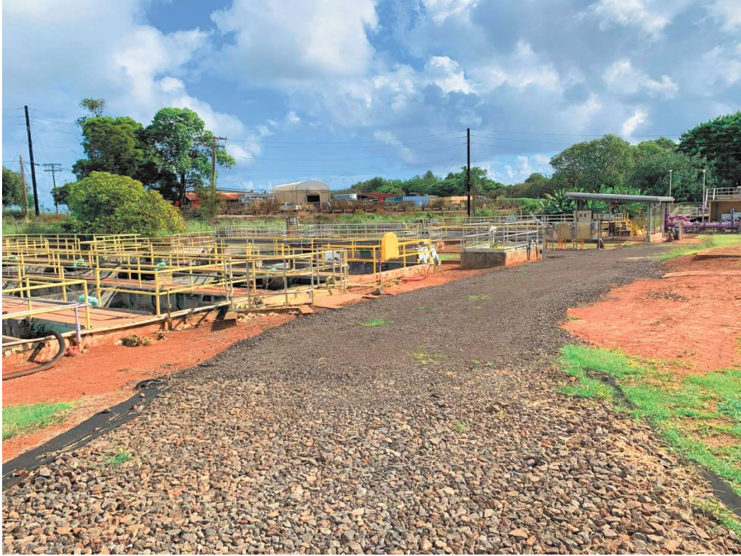
Figure 3: View of the Aerated Solids Contact Tank from the Southwest
