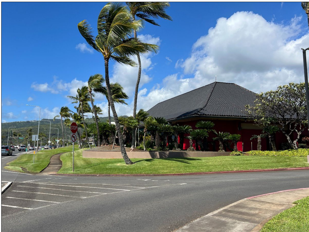
Figure 14. Slight elevation gain within parcel, view to the northwest.
