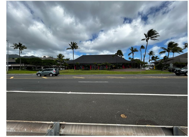
5. View Towards Scratch Hawaii Kai Building from Across Kalaniana'ole Hwy
