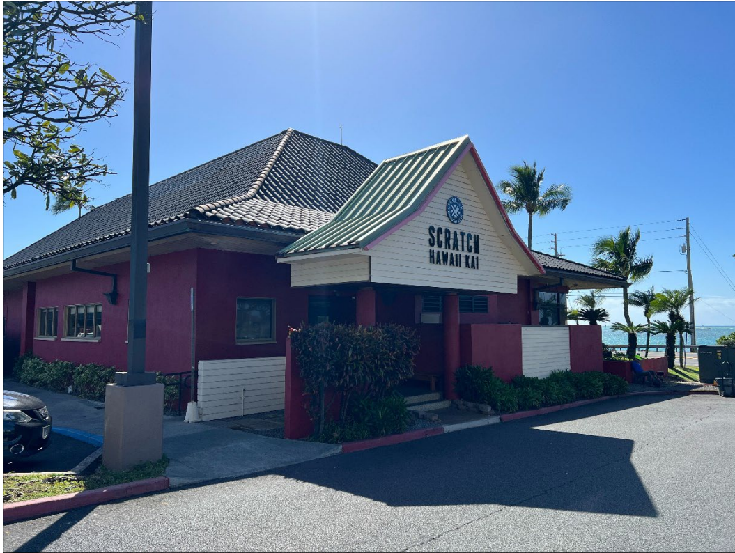
Figure 13. Restaurant building within the project area, view to the south.
