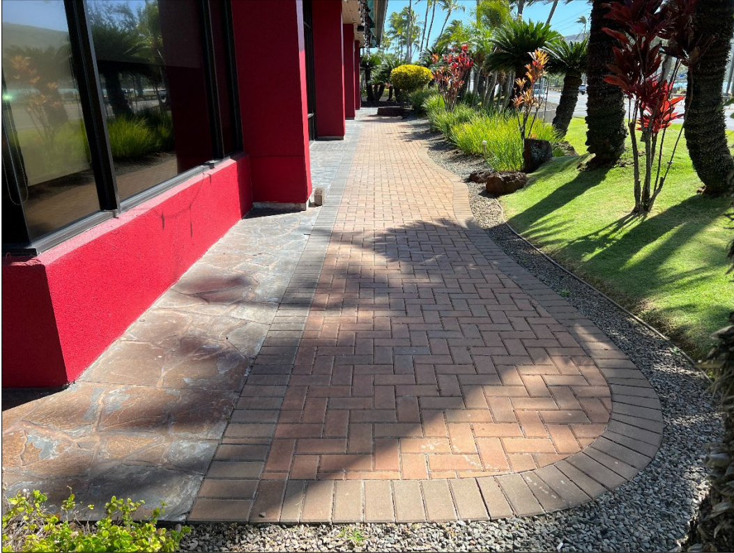
Figure 15. Walkway surrounding the restaurant building, view to the east.
