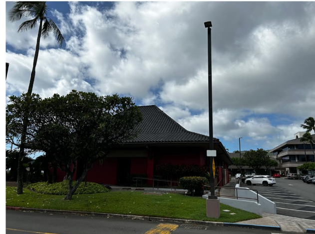
4. View Westward Towards Scratch Hawaii Kai Building
