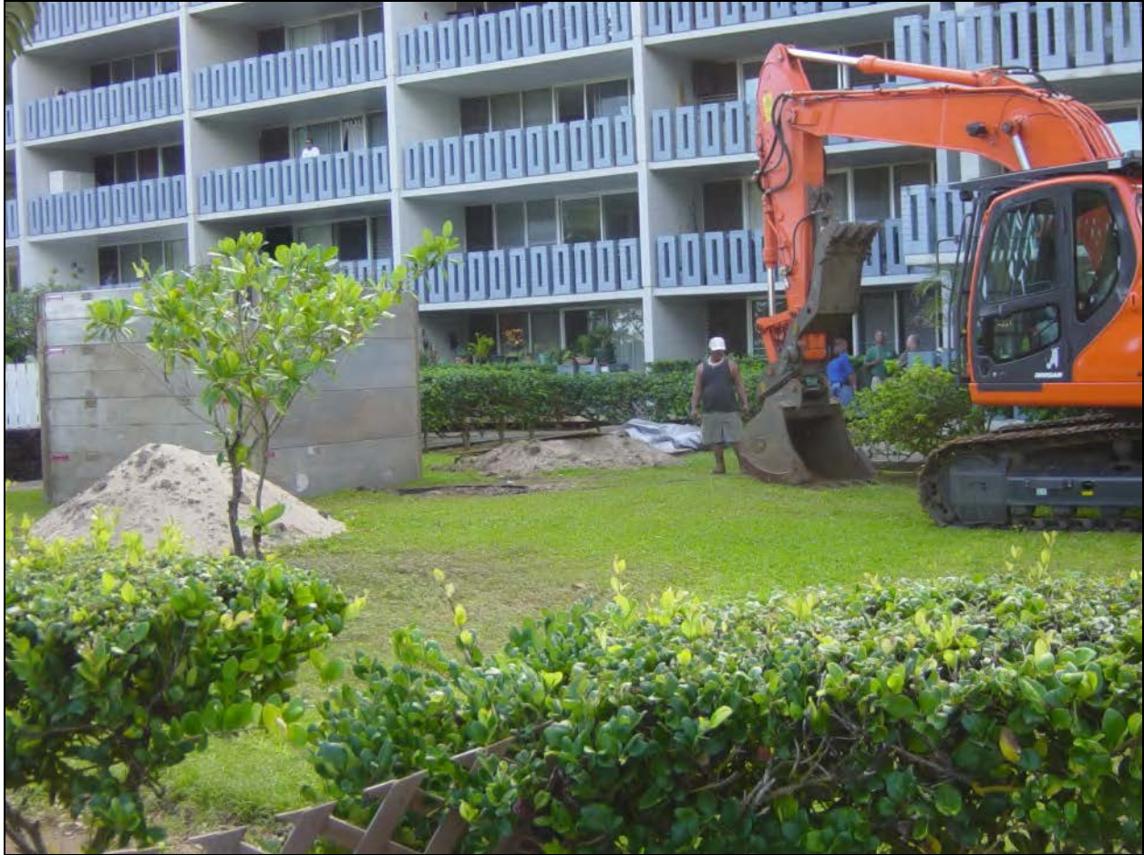
Figure 4: Photographic Overview of Project Area. View to East.
