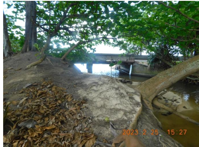
Photo 16: Punaluu Stream Bridge and Ocean In background.
