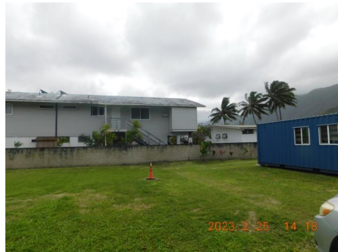
Photo 4: Unit 4 facing south. Unit 5 to right.
