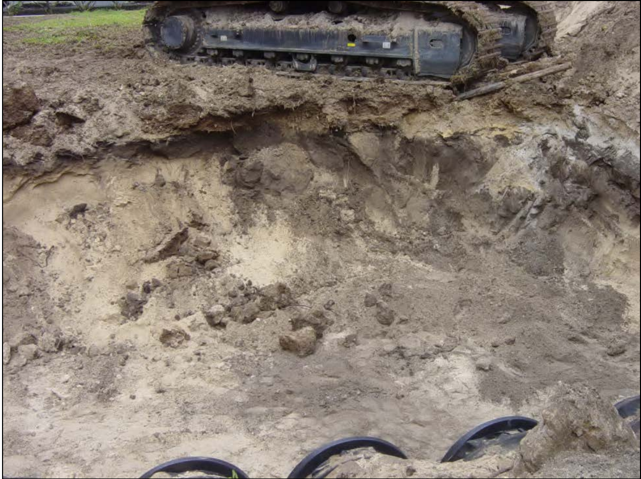
Figure 8: Photographic overview of Exposed West Section of Zone of Previous Disturbance in North Wall of Leach Field. View to West.
