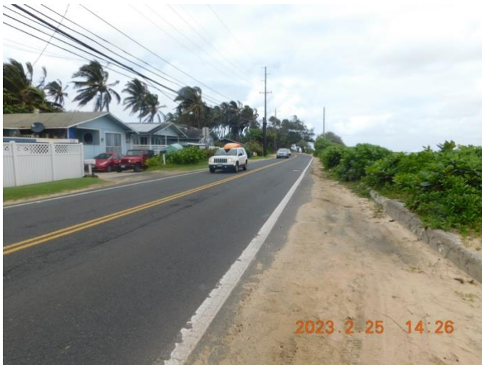
Photo 9: Kamehameha Hwy facing north, beach adjacent to the east.
