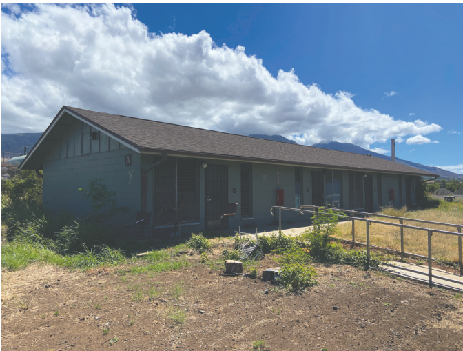
Photo 9 (facing east): View of walkway and remnant Building A.
