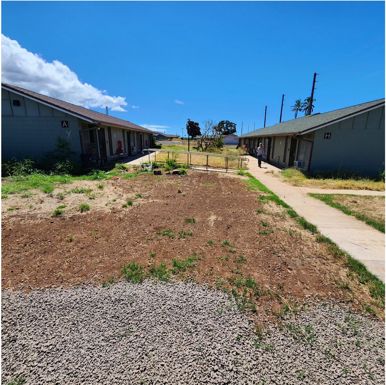
Photo 5: Piilani site buildings that were not burned (5 buildings remain onsite).
