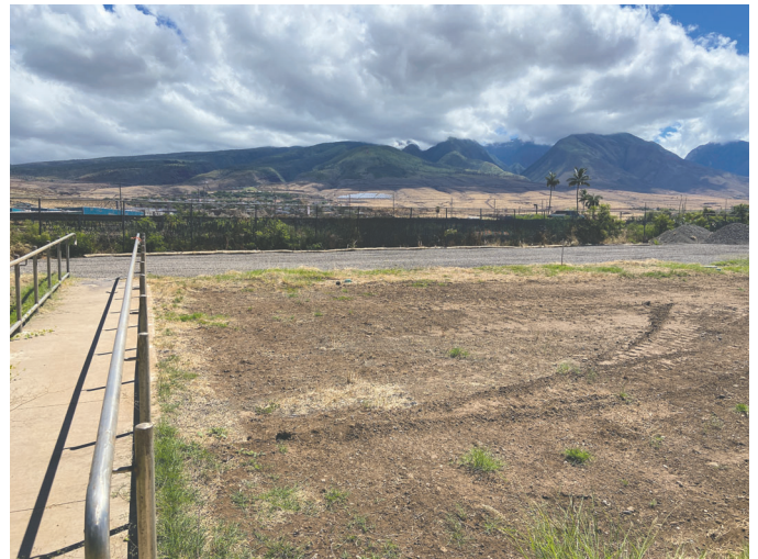
Photo 10 (facing east): View of walkway leading to destroyed Building B near northeastern boundary.
