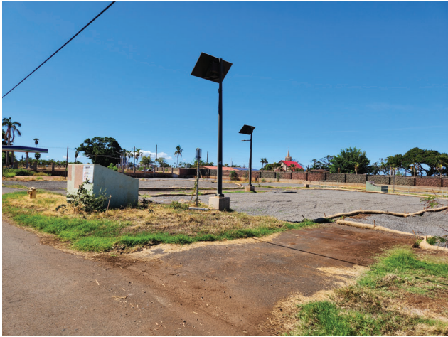
Photo 01. View of David Malo Circle Housing Site
