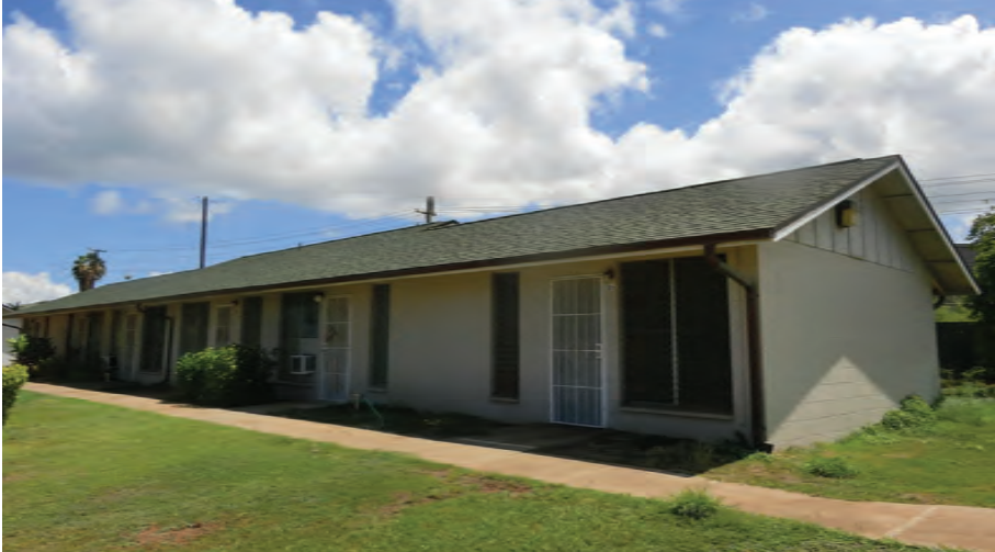
Figure 137: Piilani Homes Building B Front Elevation Source: Fung Associates Inc., 2020
