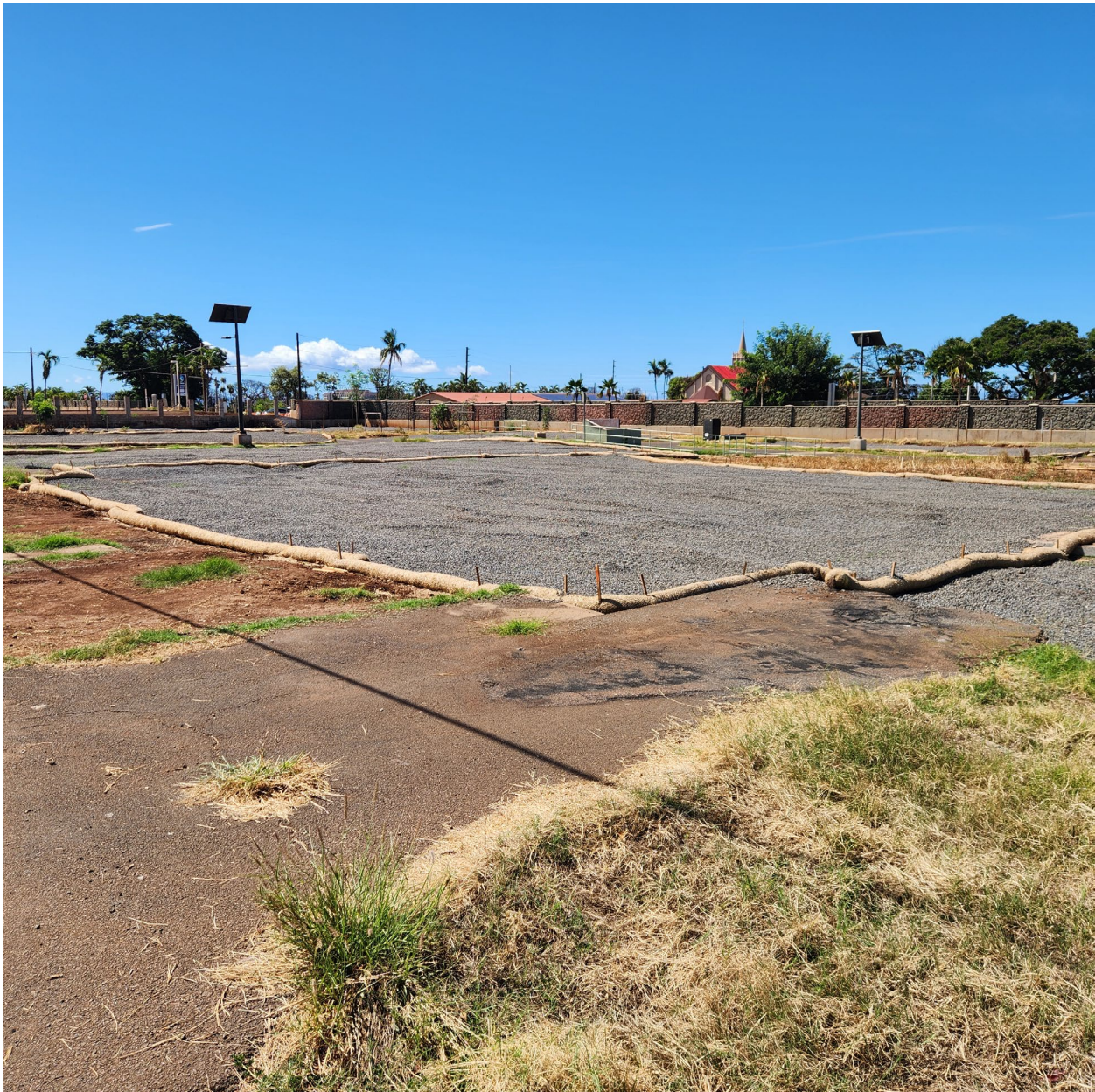
Photo 2: David Malo site condition. Note USACE-placed clean gravel and erosion protection at each former building location. Also note clear areas of soil (not gravel) was not included in USACE cleanups and may need to be tested prior to redevelopment/grading, etc.
