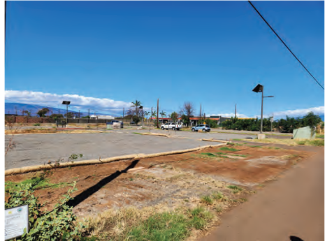
Photo 02. View of David Malo Circle Housing Site
