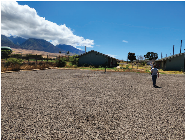
Photo 03. View of Piilani Homes Site Cleared by USACE
