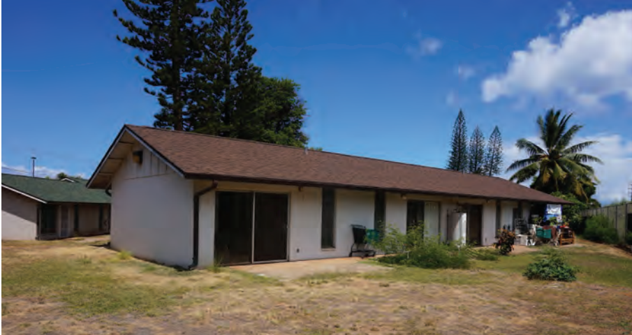
Figure 141: Piilani Homes Building D Rear Elevation Source: Fung Associates Inc., 2020
