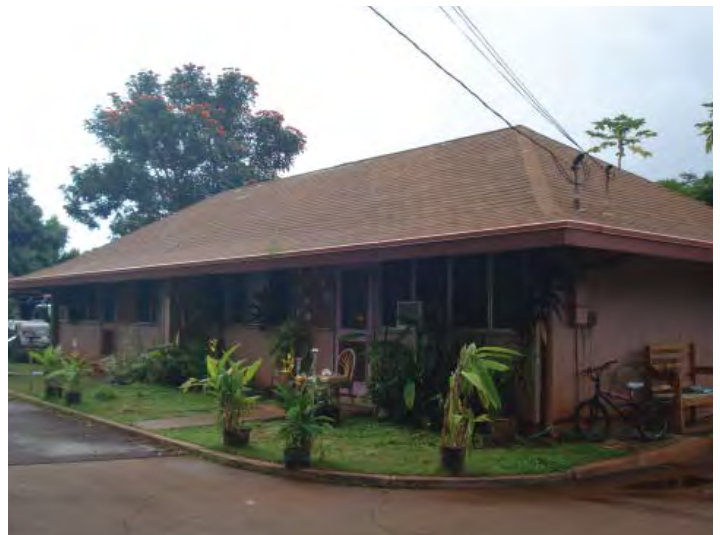
Typical Single Story Building
