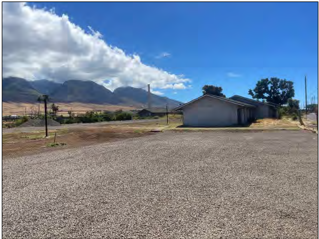
Figure 10. Former location of Building G (above) and Former Location of Building G with former location of Building C visible to the left (MASON, September 2024)
