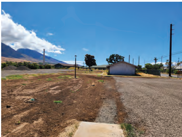
Photo 05. View of Cleared Areas for Former Buildings at Piilani Homes
