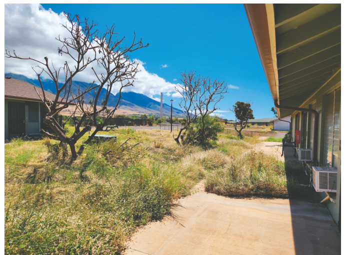
Photo 12 (facing south): View of walkway and frontage of remnant Building B.
