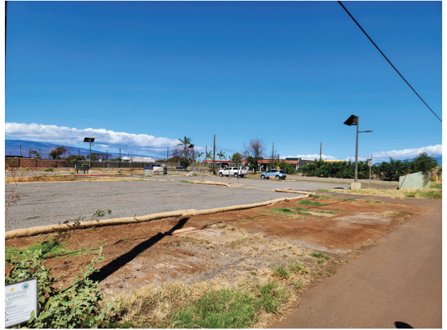
Photo 02. View of David Malo Circle Housing Site
