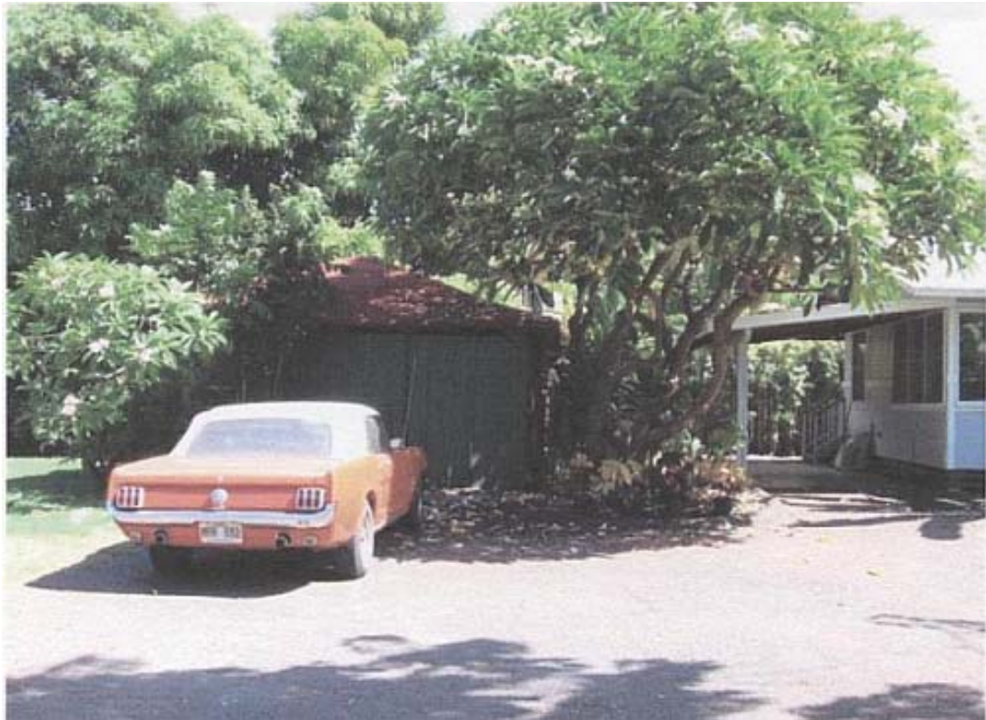
Photo of garage
