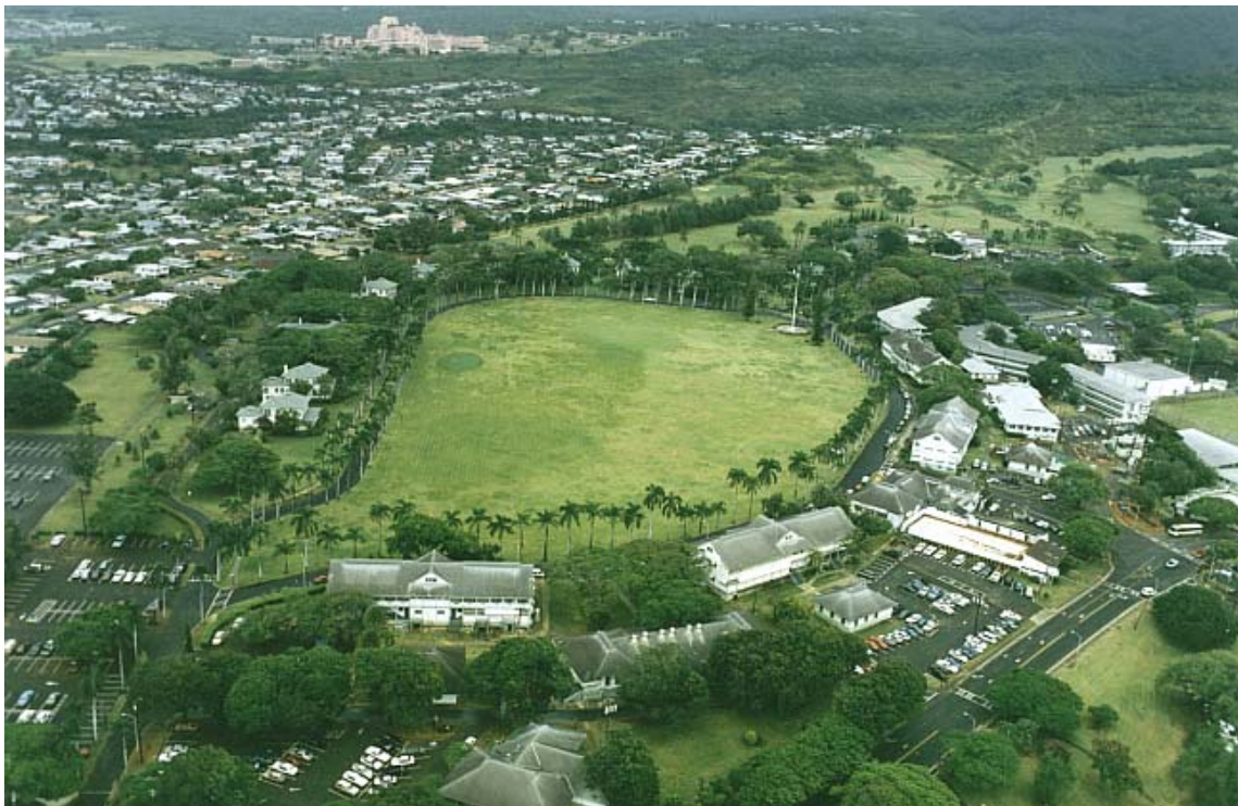
Aerial of Palm Circle
