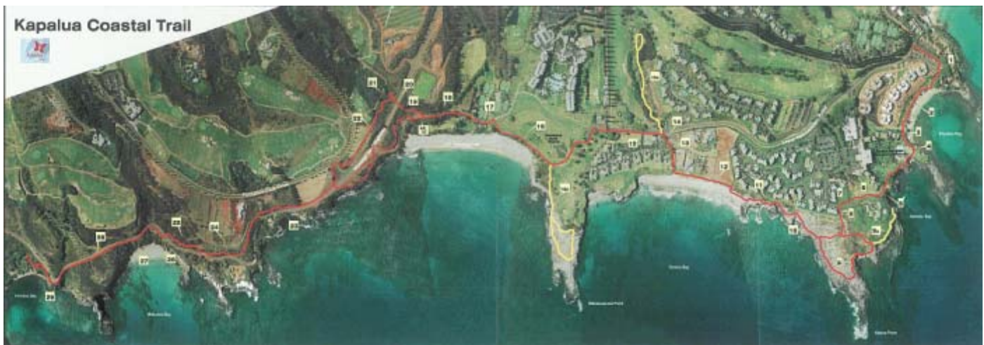
Aerial of project site
