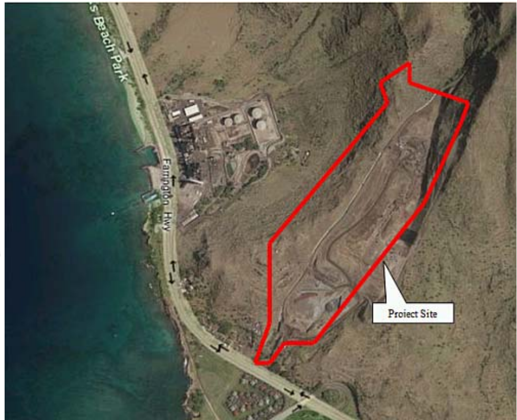
Aerial of Project Site
