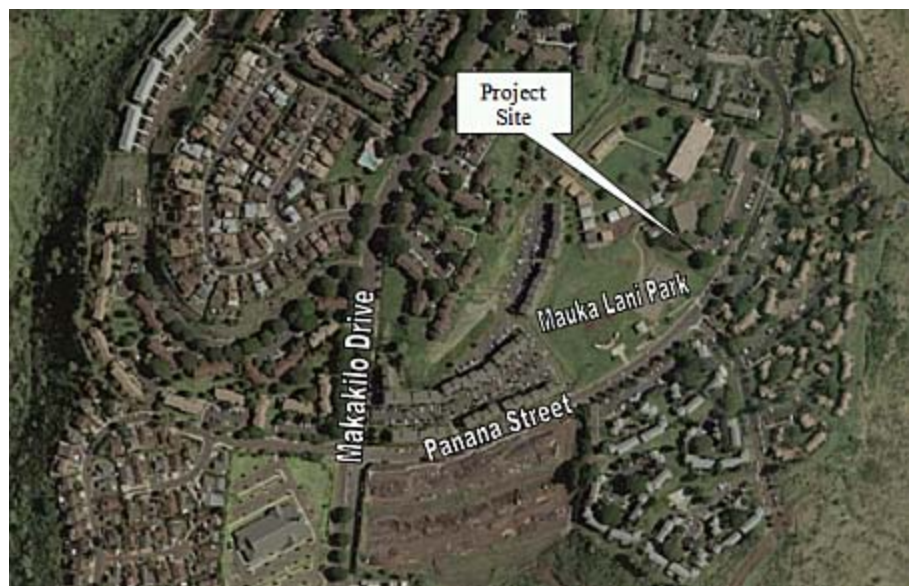
Aerial of Project Site
