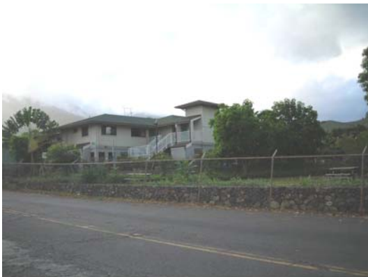
View of proposed site for Ke Kama Pono facility
