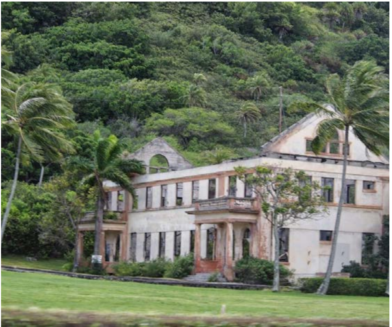
The structure and grounds on this long-used and previously abandoned site on Oahu's North Shore are planned for adaptive re-use
