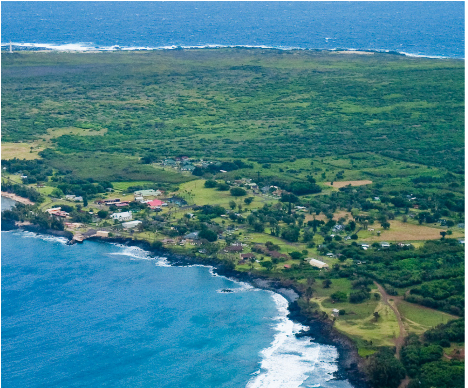
An upgraded electrical system is proposed for Kalaupapa National Historical Park on Molokai
