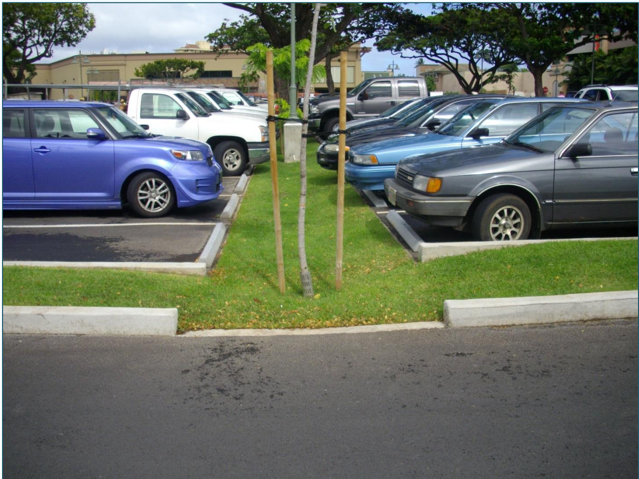
An open swale (Oahu) that accepts parking lot runoff.
