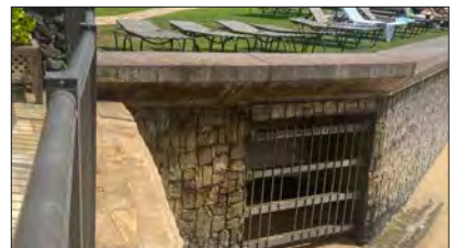
Completed storm drain repairs Source: Kahana Sunset photo archive (2023)
