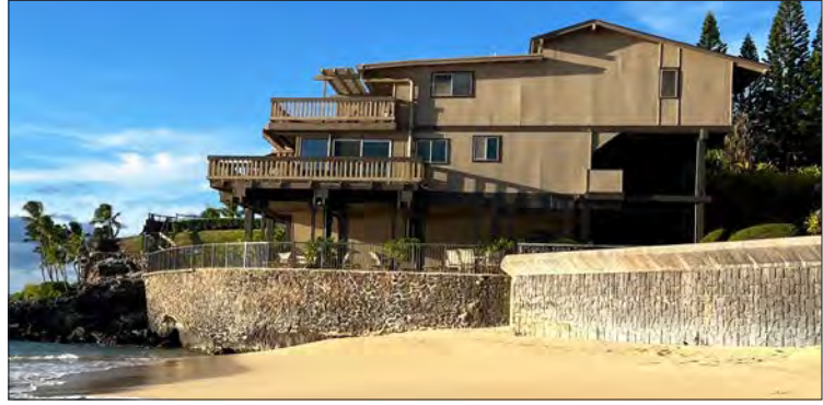
Kahana Sunset sandbags and removal of sandbags
