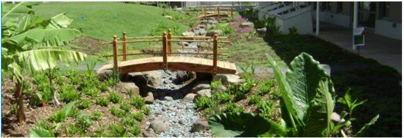
Infiltration Trench at Punahou School (Courtesy of the City and County of Honolulu)
