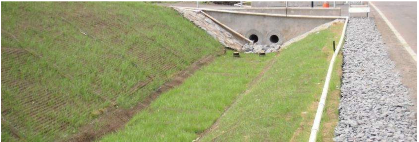
Bioswale adjacent to Kumuhaio Street, Waimanalo, O’ahu (Courtesy of the City and County of Honolulu)
