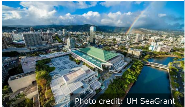
Figure 1-5: Green Roof on the Hawai'i Convention Center
